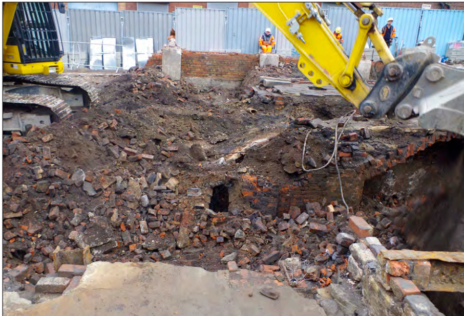
Plate 18: Entrance of north-west end of flue 4066 into engine pit. From west
