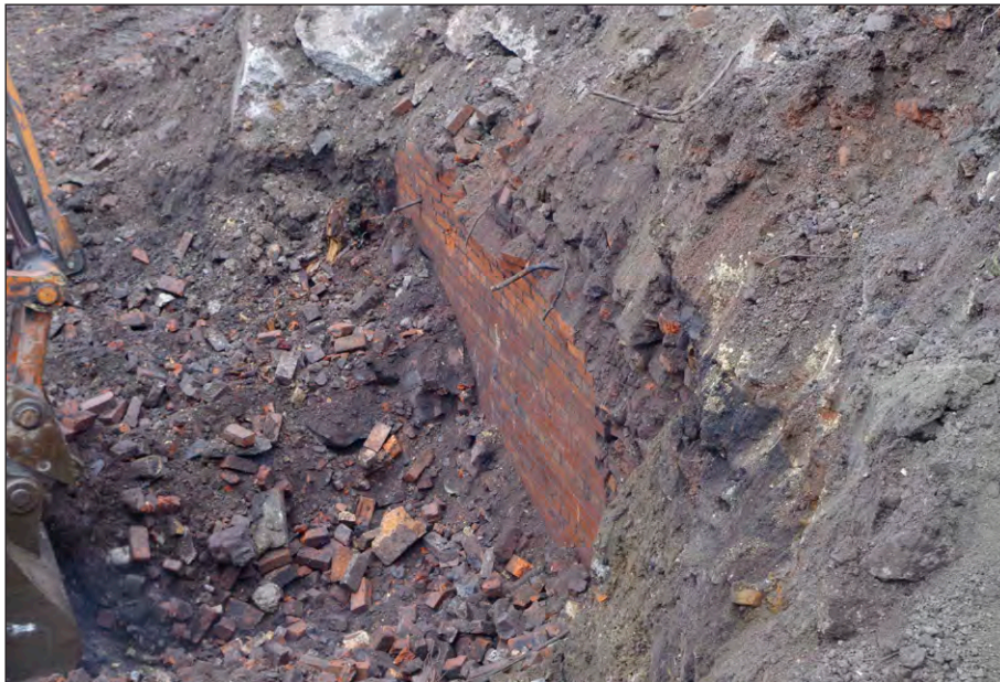
Plate 36: Structure 4357 seen under watching brief conditions from north-east
