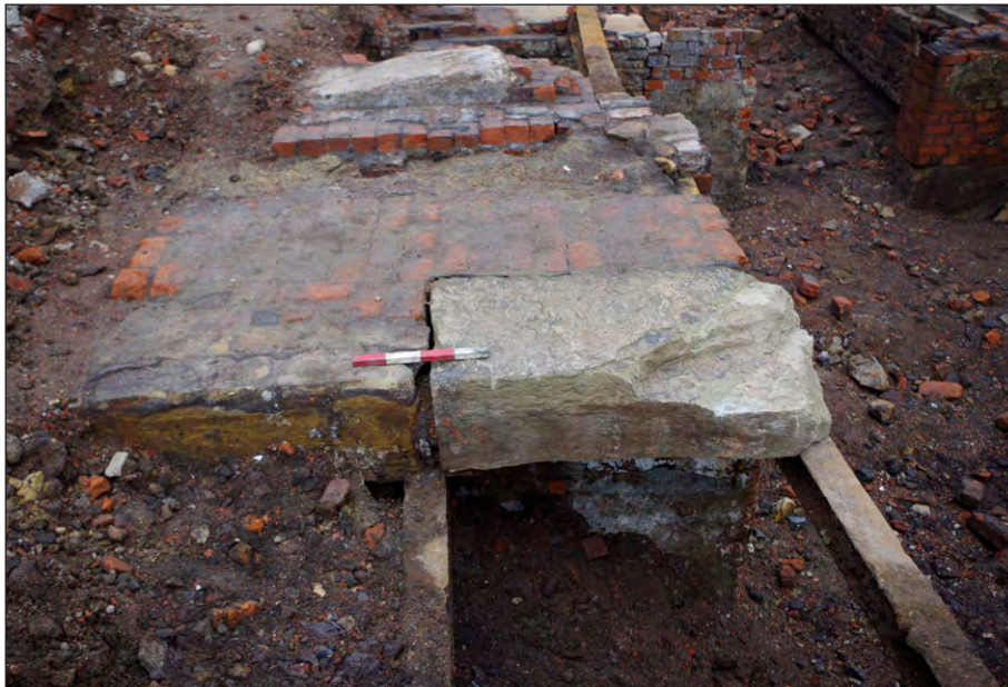
Plate 32: Girders 1010 and 4120 support sandstone surface 4117–4119 from south
