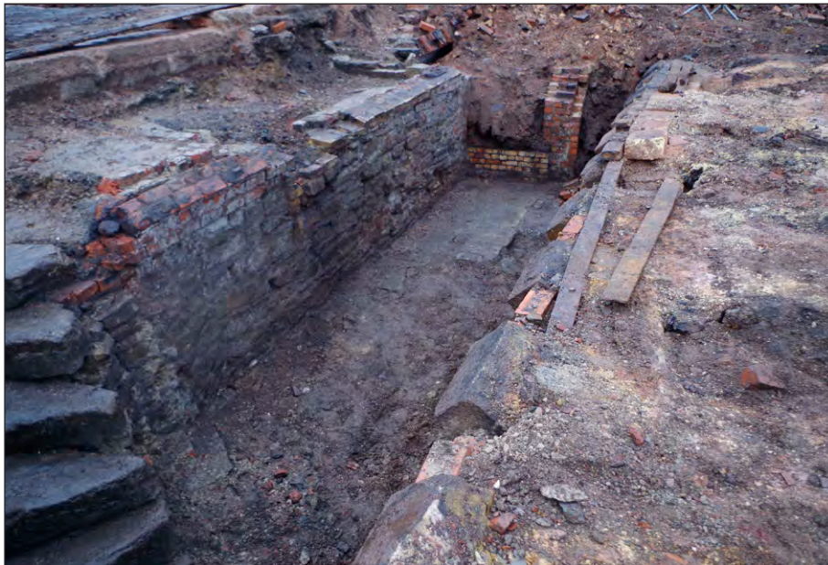
Plate 12: Crucible cellar including wall 4309 and surface 4234 from north-east
