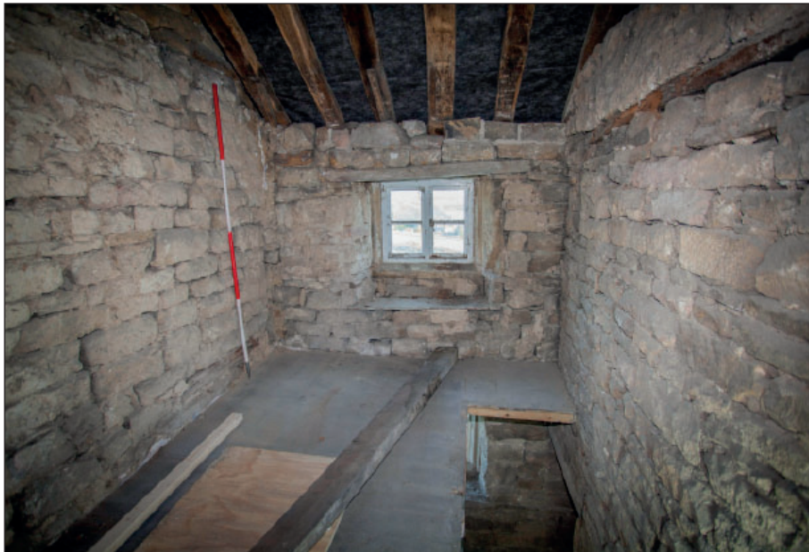
Plate 104: F3, looking east
