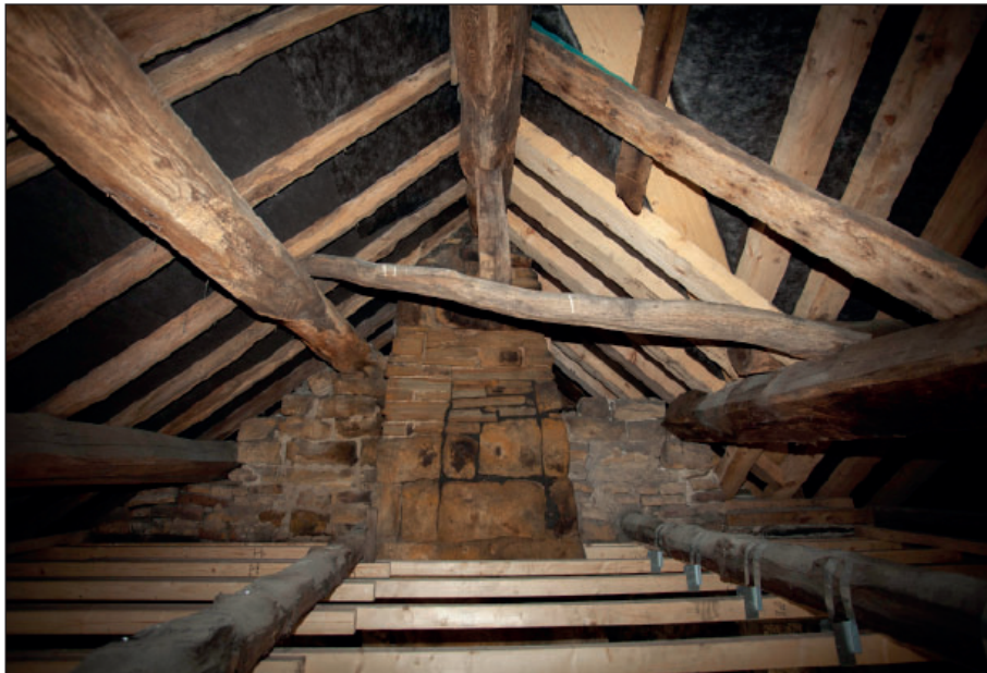
Plate 96: F1, upper section of chimney breast
