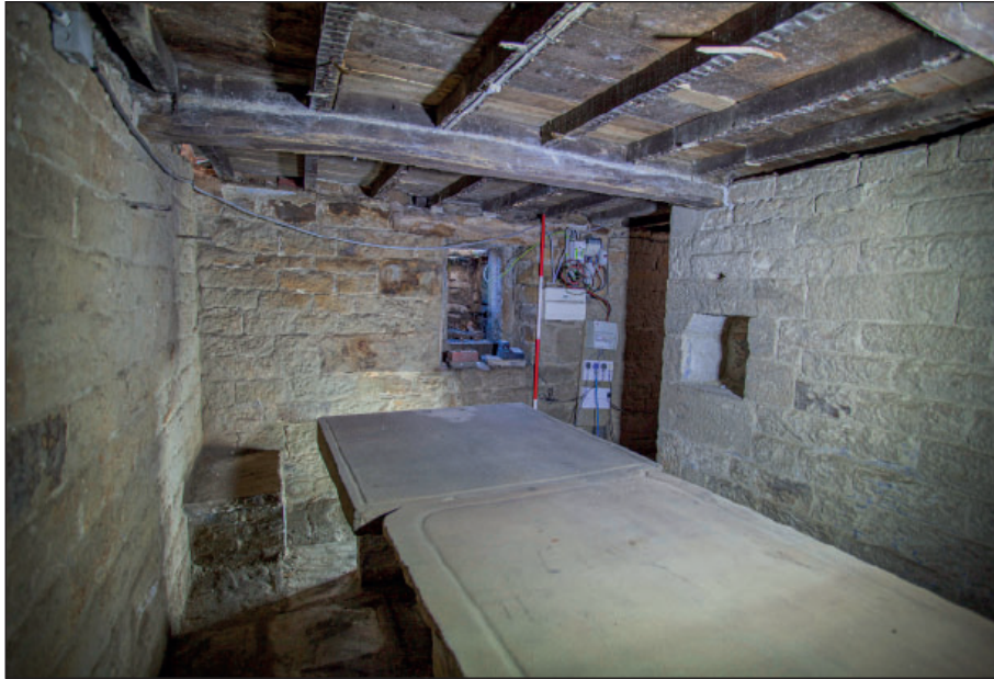
Plate 41: C1, original lightwell within the east wall
