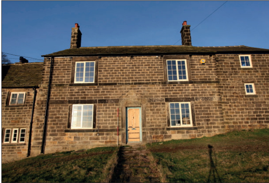
Plate 9: East elevation, detail of the Farmhouse façade
