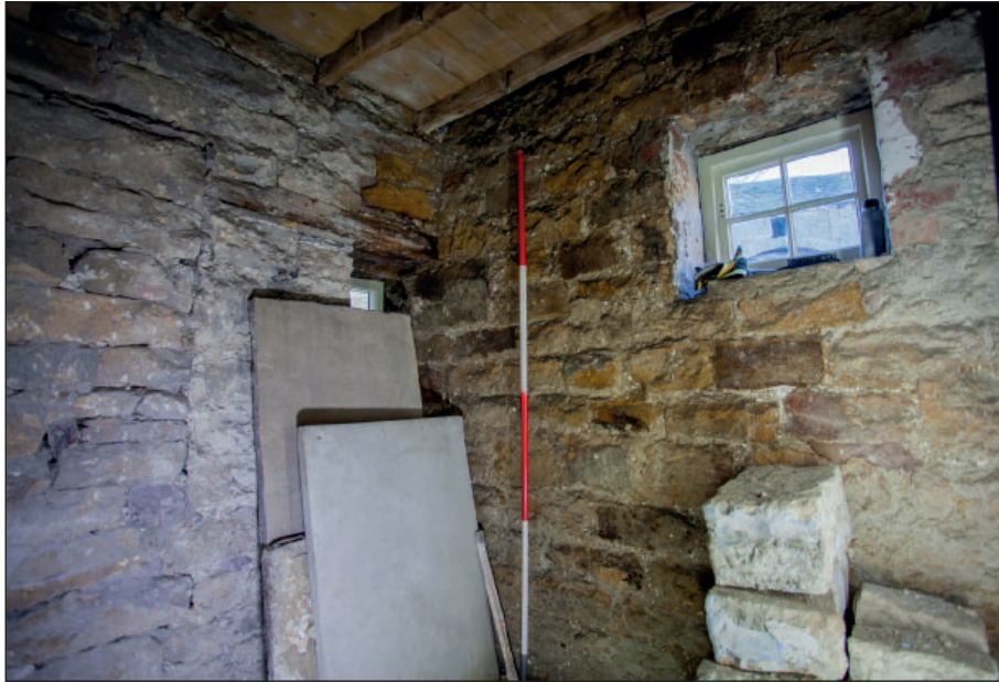
Plate 73: G7, partially blocked window within the south wall
