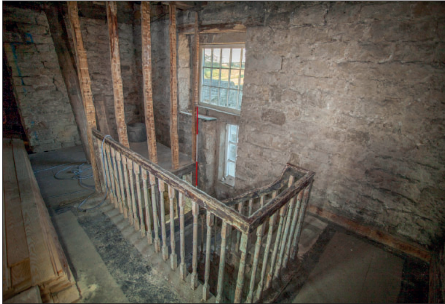
Plate 121: F7, staircase and landing
