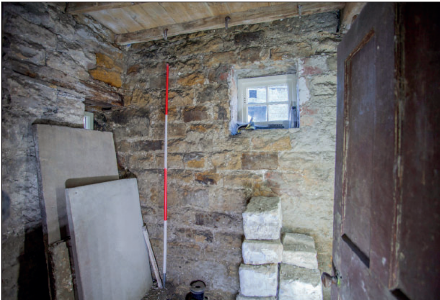
Plate 72: G7, inserted window within the west wall
