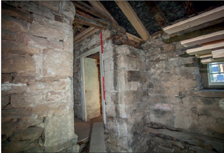
Plate 109: F3, doorway to F1, note the bullnosed jamb to the left
