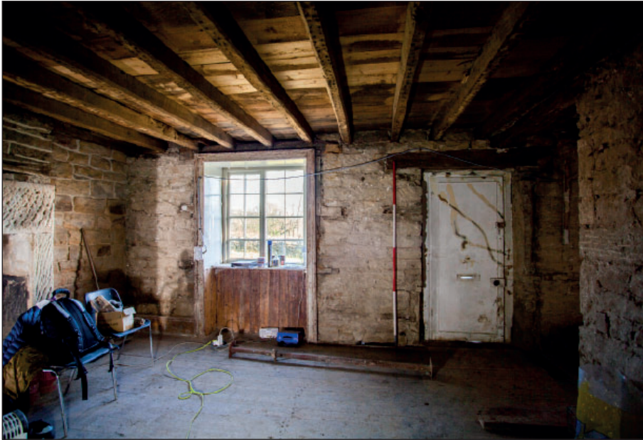
Plate 71: G6, window opening and doorway within the east wall
