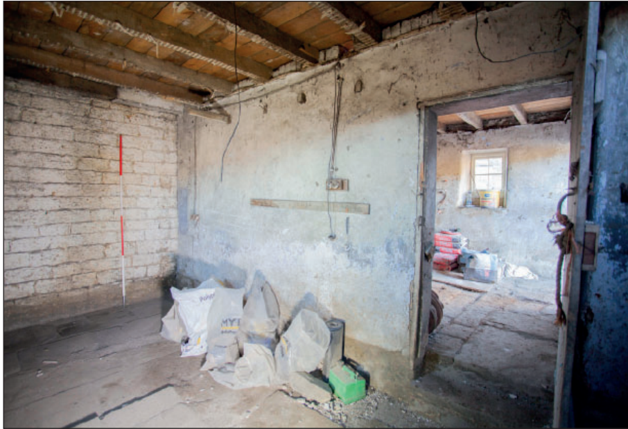
Plate 89: G11, looking west
