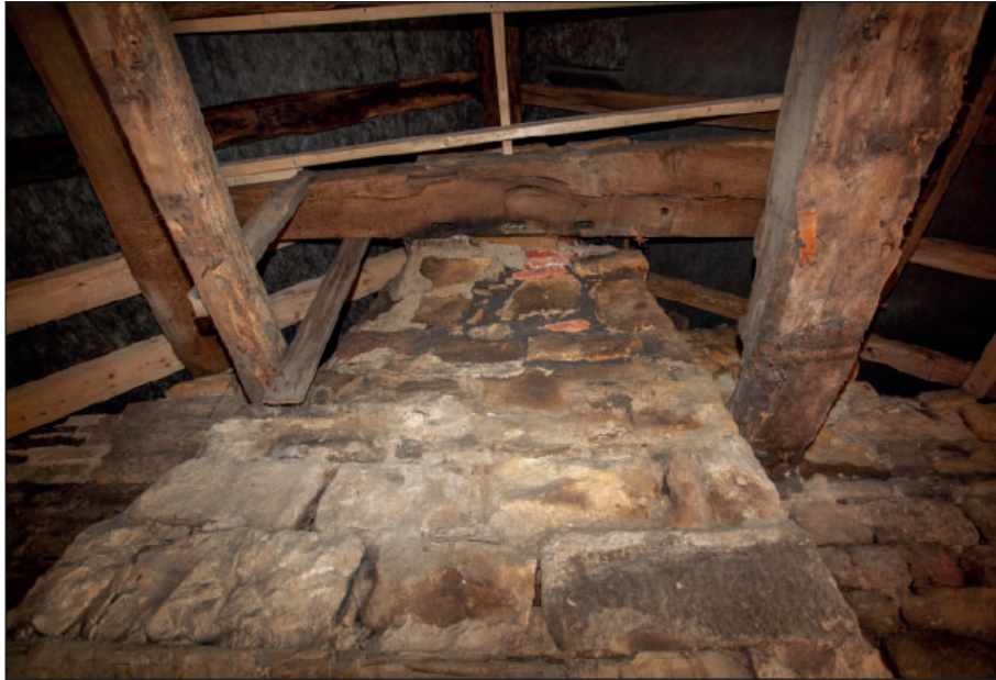
Plate 99: F2, upper section of chimney breast
