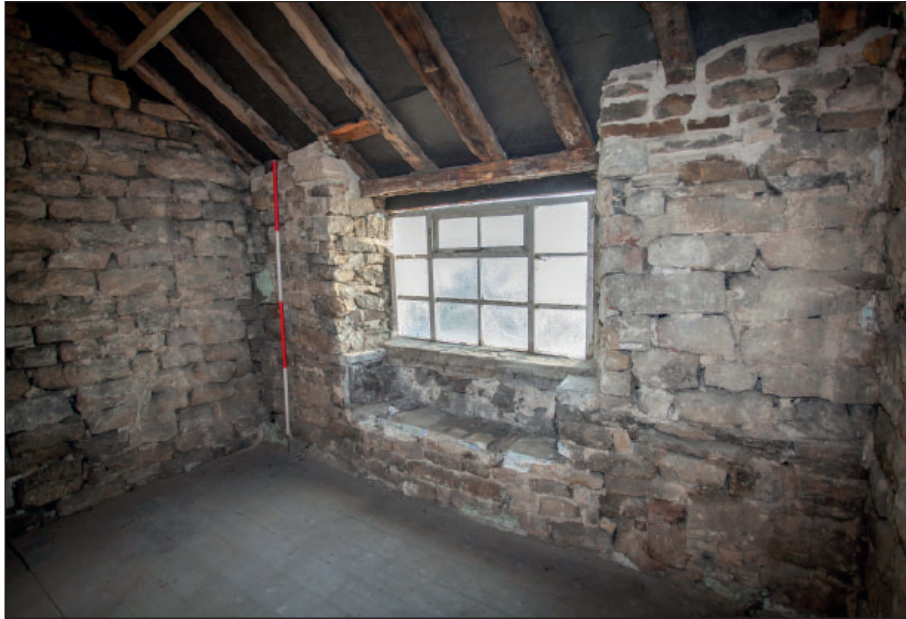
Plate 103: F2, detail of inserted window within the south wall
