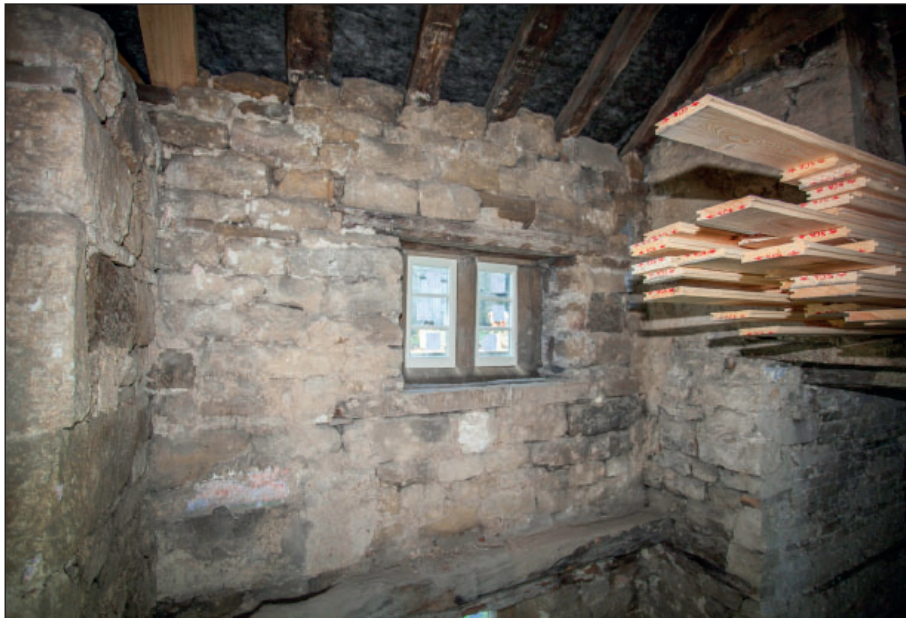
Plate 108: F3, detail of mullioned window within the west wall
