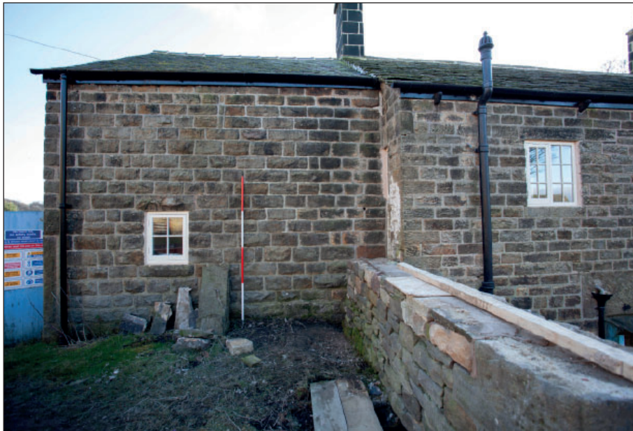
Plate 32: West elevation, detail of the northern extension
