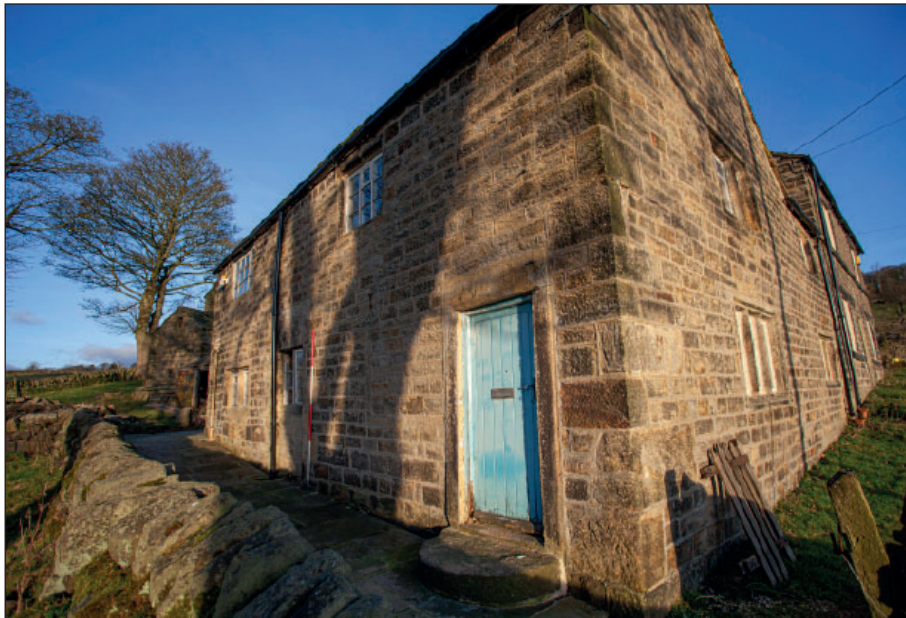
Plate 16: South elevation, detail of dressed corner quoins
