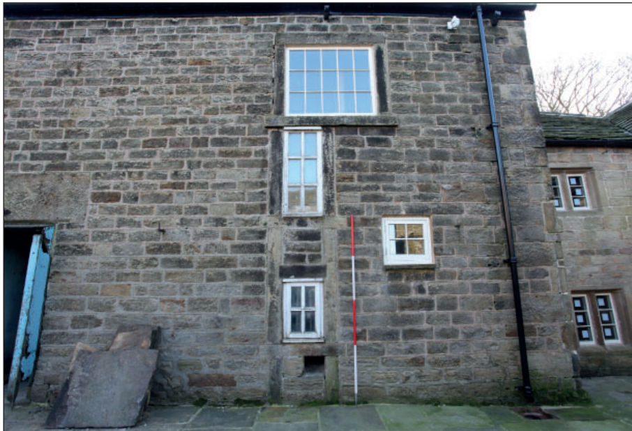
Plate 28: Detail of window architraves within the rear façade of the Farmhouse
