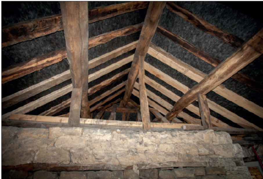
Plate 110: F3, roof structure above the dividing wall between F1 and F3
