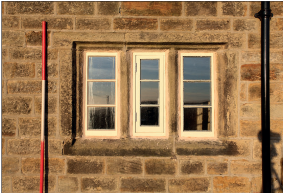
Plate 6: East elevation, ground floor northern window
