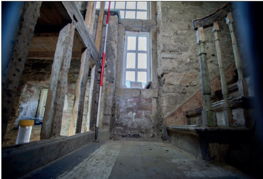
Plate 122: F7, detail window opening within the west wall
