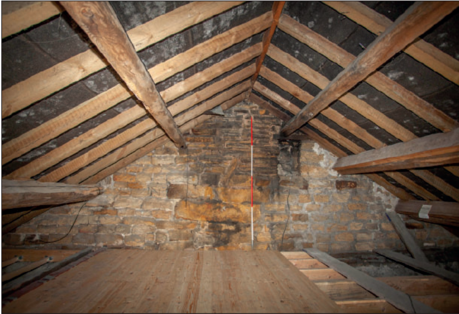
Plate 131: A1, south gable wall with blocked window opening
