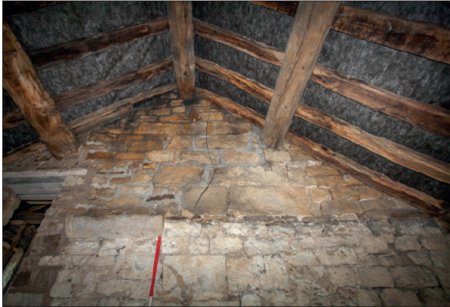
Plate 107: F3, detail of projecting corbel stone and roof structure
