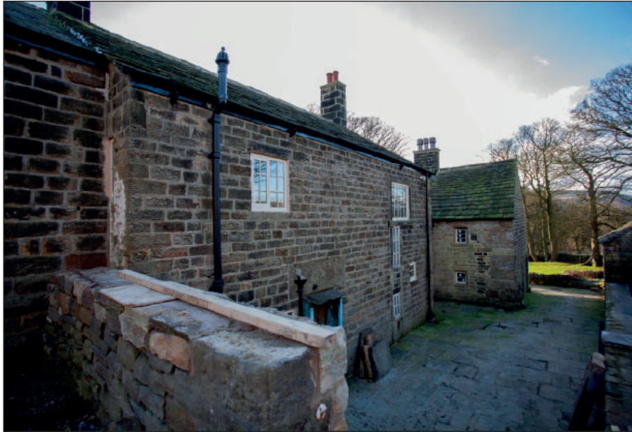
Plate 31: Rear façade of the Farmhouse, looking south
