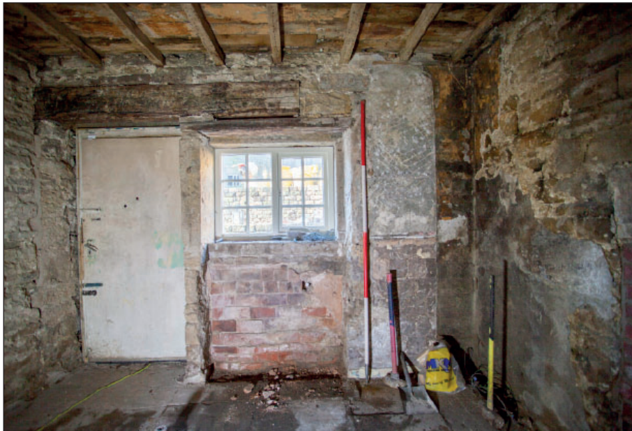
Plate 84: G9, external doorway and adjacent window opening
