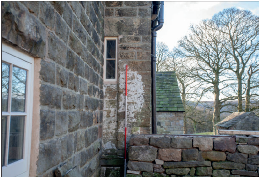
Plate 38: North-western end of the Farmhouse with partially blocked opening
