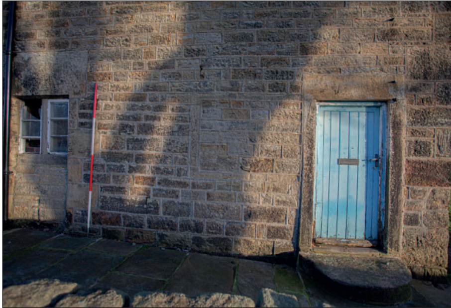
Plate 17: South elevation, detail of inserted doorway and adjacent blocked window
