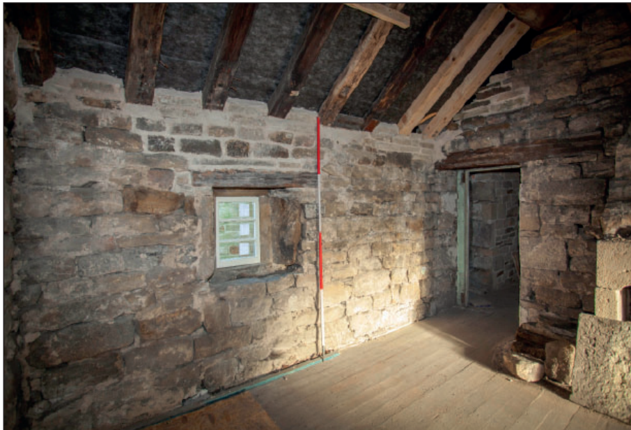
Plate 102: F2, detail of window opening within the north wall
