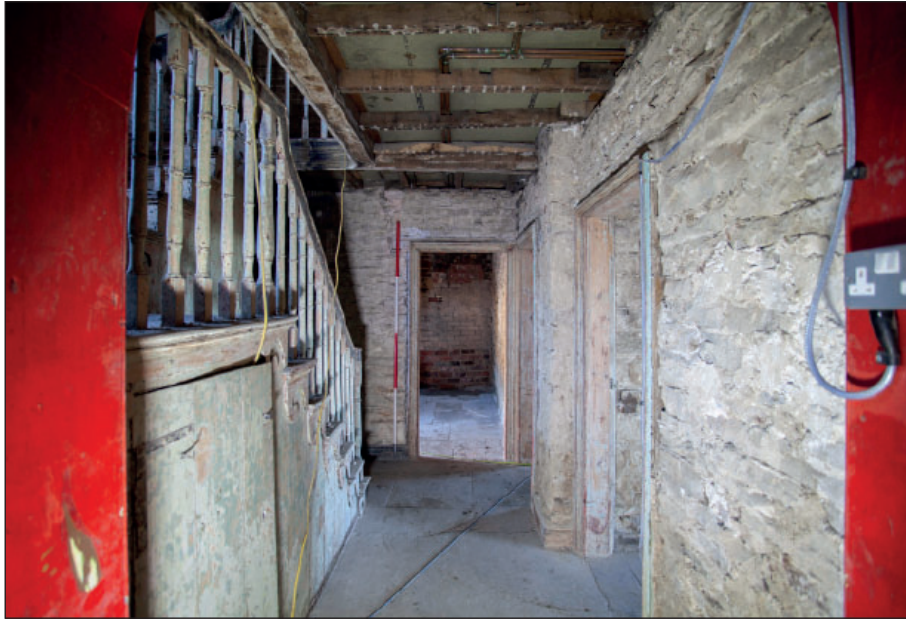
Plate 77: G8, staircase and doorways
