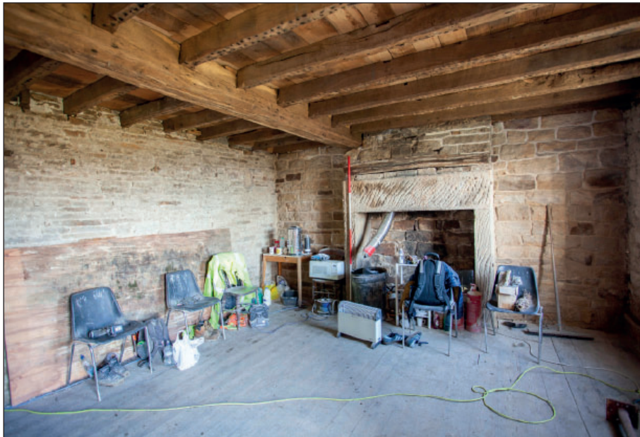
Plate 68: G6, fireplace within the north wall
