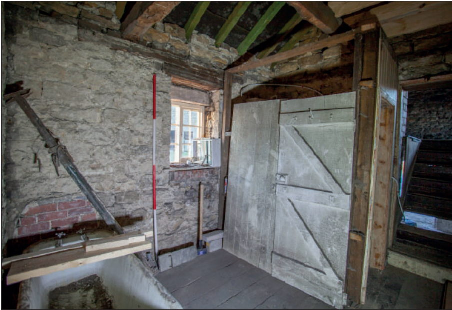
Plate 127: F8, looking north-west
