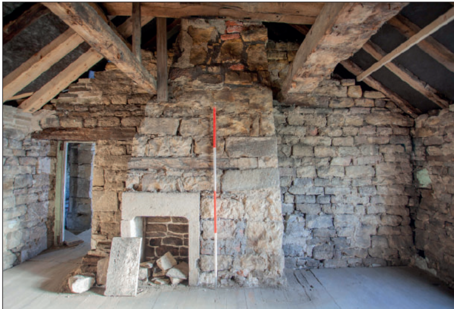
Plate 98: F2, general view of fireplace
