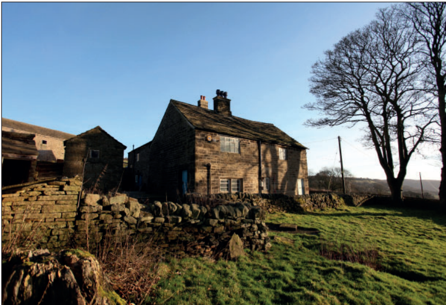
Plate 20: General view of the south and west elevations, looking north-east
