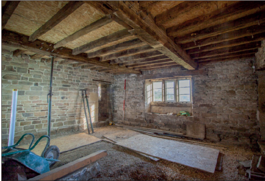
Plate 51: G1, mullioned window within the east wall
