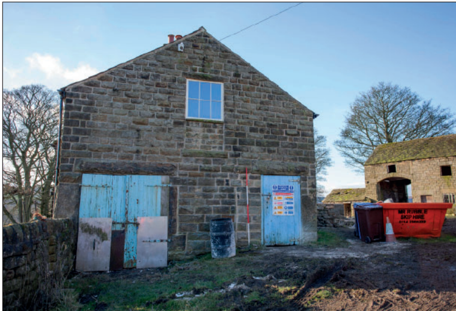
Plate 36: North elevation of the northern extension
