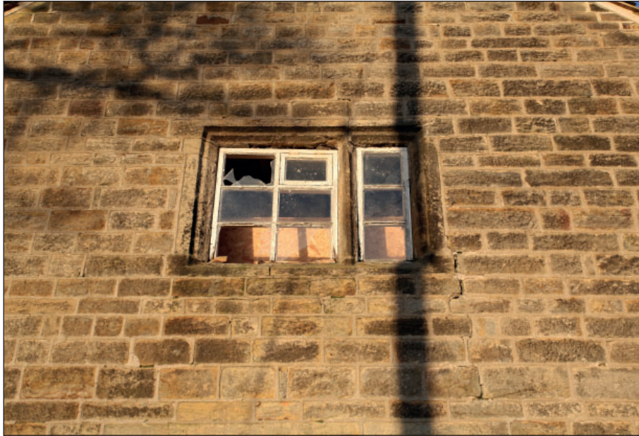
Plate 7: East elevation, first floor southern window
