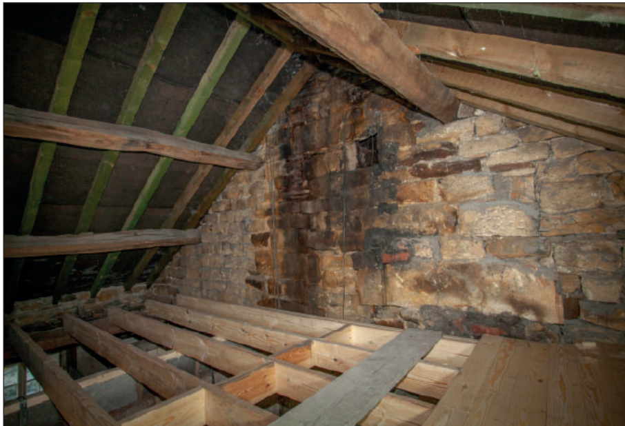
Plate 134: A2, north gable wall
