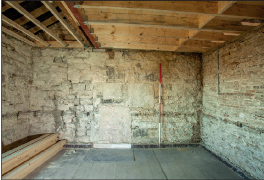
Plate 111: F4, general view of the blocked fireplace
