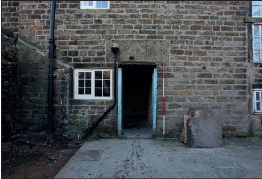
Plate 29: Detail of rear doorway of the Farmhouse
