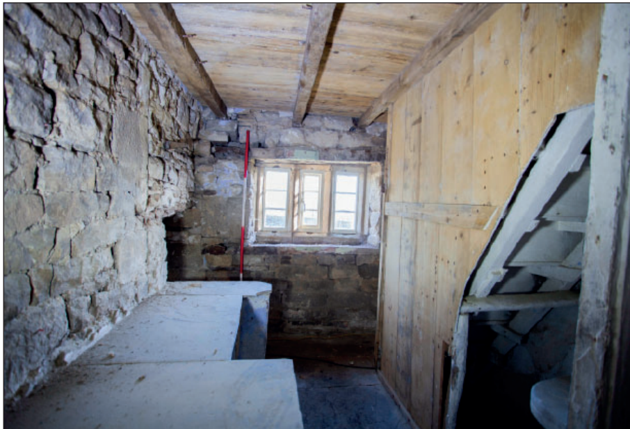
Plate 60: G4, mullioned window and inserted staircase to the first floor
