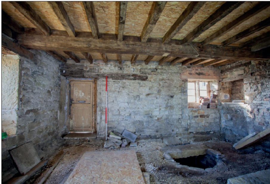
Plate 48: G1, inserted doorway and window opening
