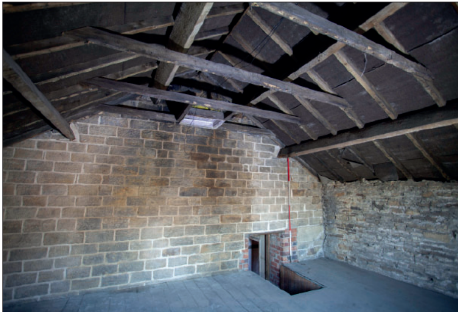
Plate 130: F10, south wall with inserted doorway and adjacent blocked opening
