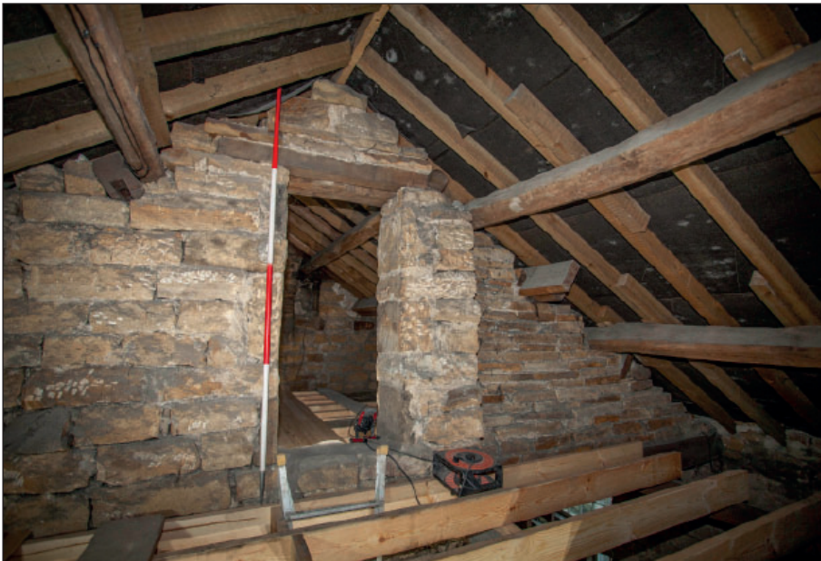
Plate 136: A2, detail of doorway and thinner wall to the right
