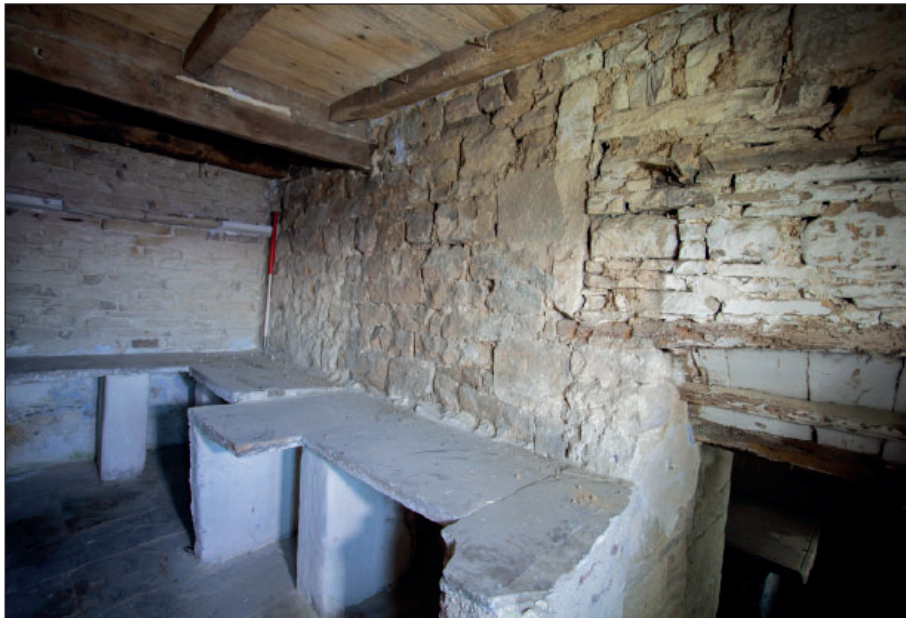
Plate 62: G4, detail of stone benches
