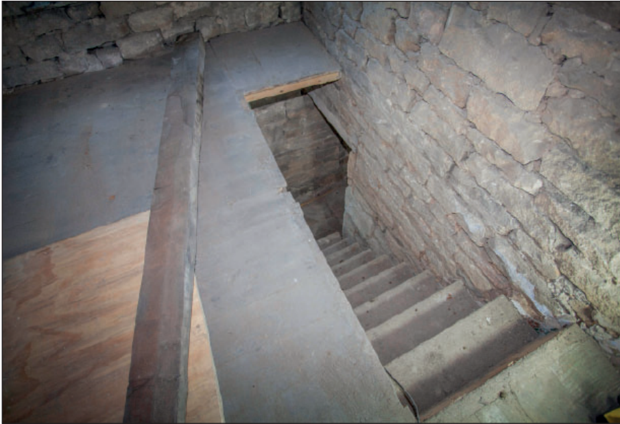
Plate 105: F3, inserted staircase
