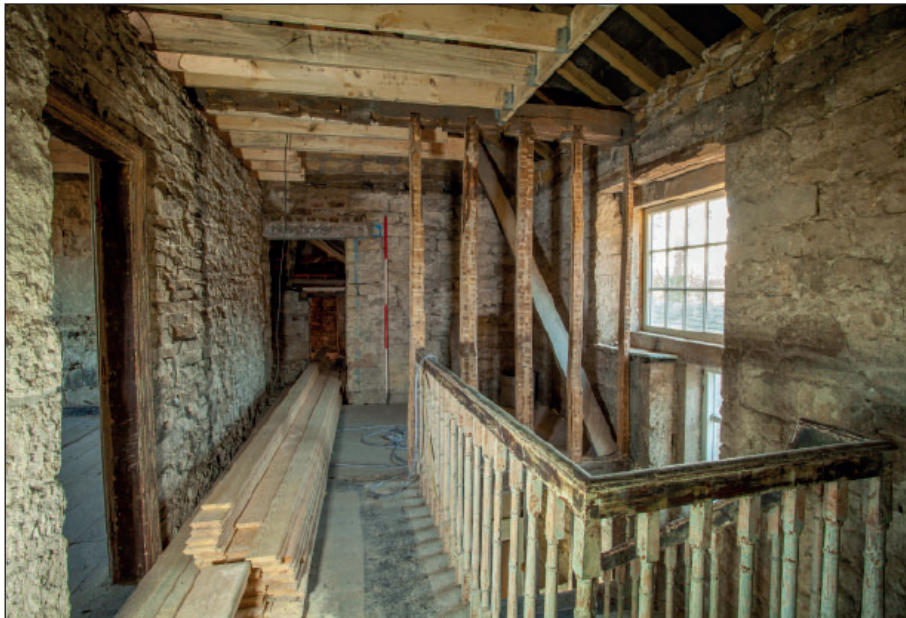
Plate 124: F7, general view of the landing
