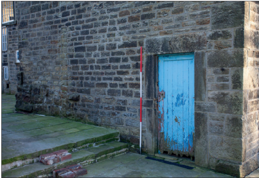
Plate 23: Cottage rear façade, detail of inserted doorway
