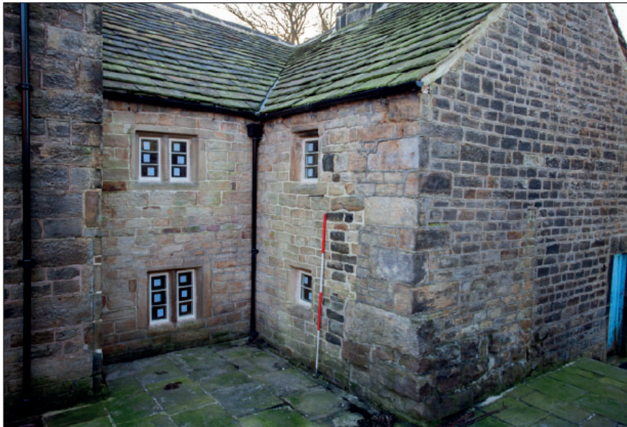
Plate 34: North elevation of the Cottage
