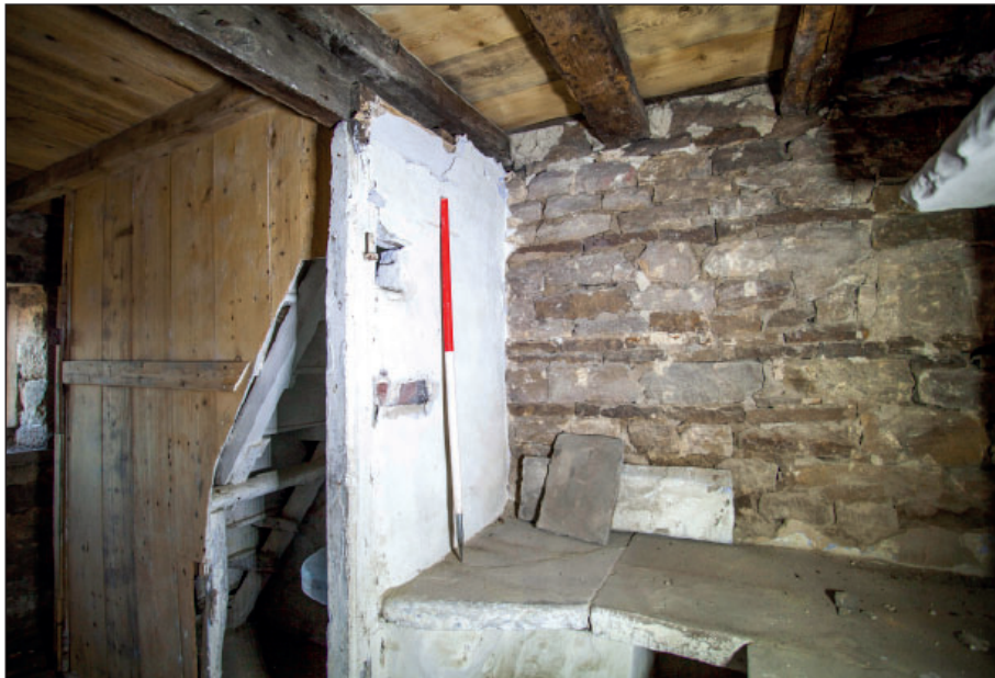
Plate 64: G4, stud partition of inserted staircase to the first floor
