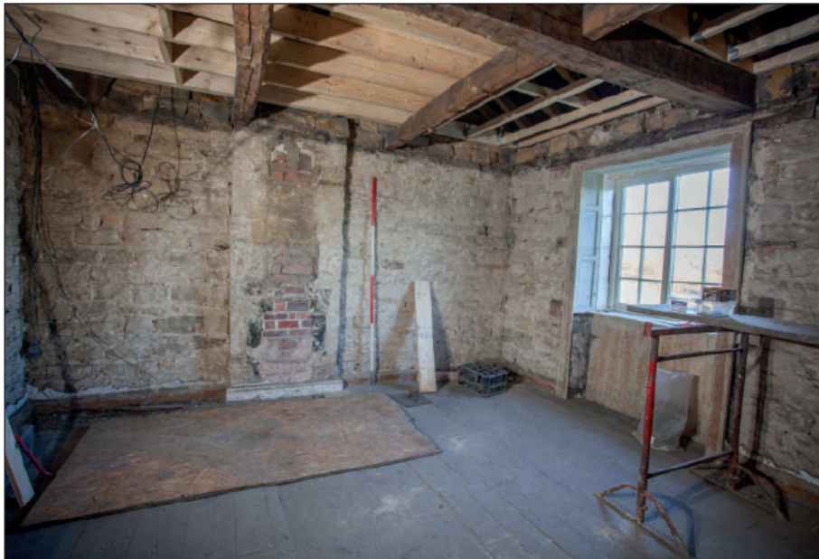
Plate 114: F5, general view of blocked fireplace
