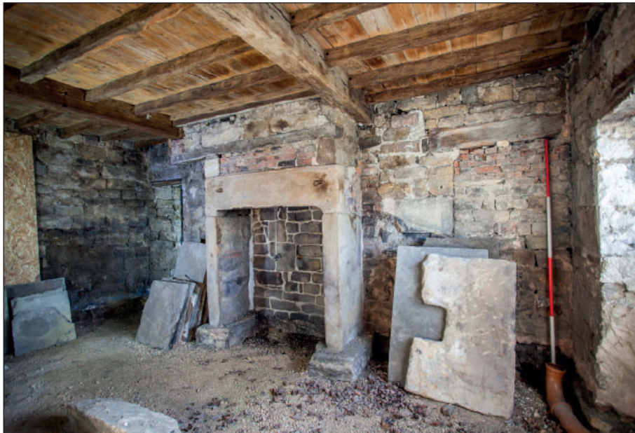
Plate 54: G2, detail of blocked doorway to the south of the fire
