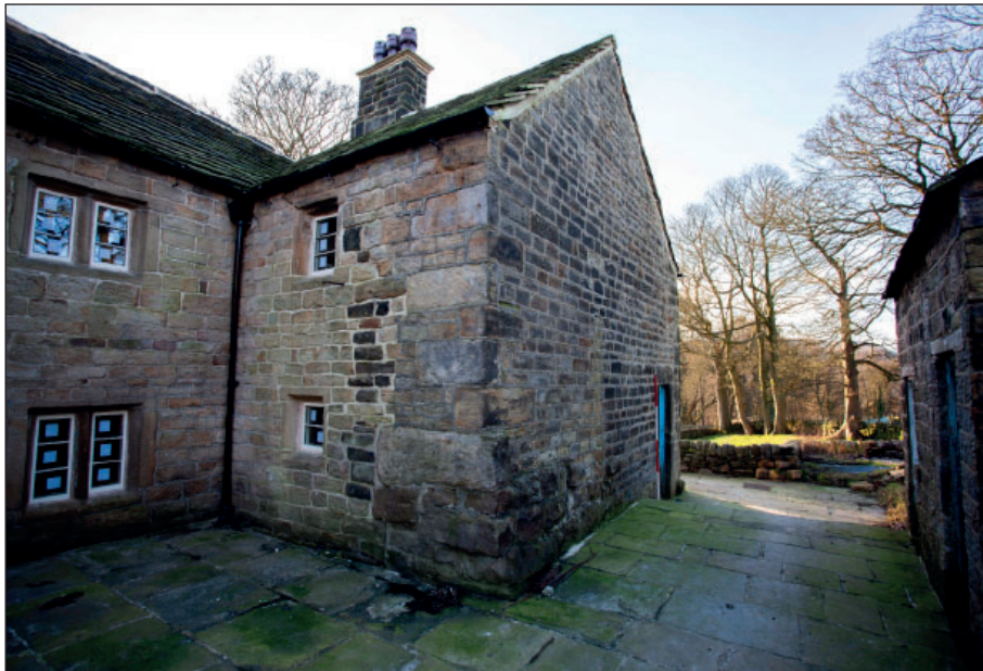
Plate 22: Cottage rear façade with dressed quoins and lower exposed foundation
