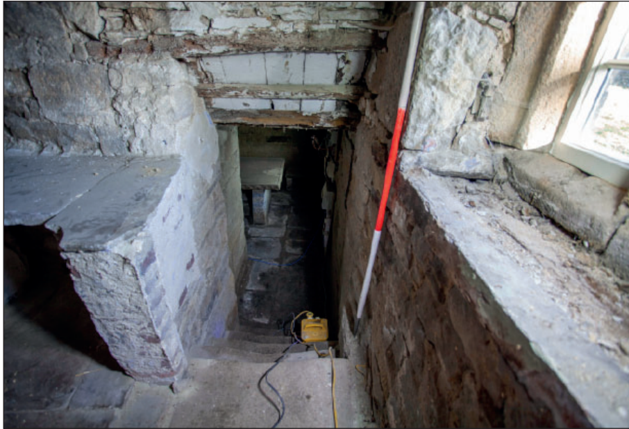
Plate 61: G4, staircase to cellar C1 and blocked door over
