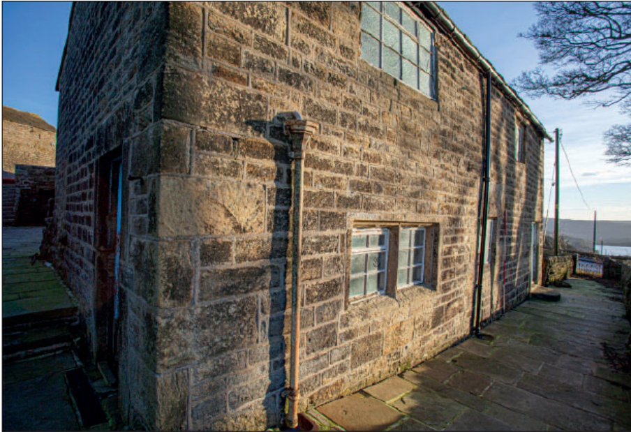
Plate 19: South elevation, western side with dressed corner quoins
