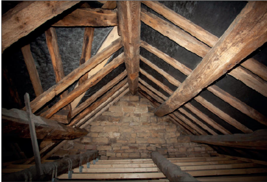
Plate 97: F1, east gable wall and roof structure
