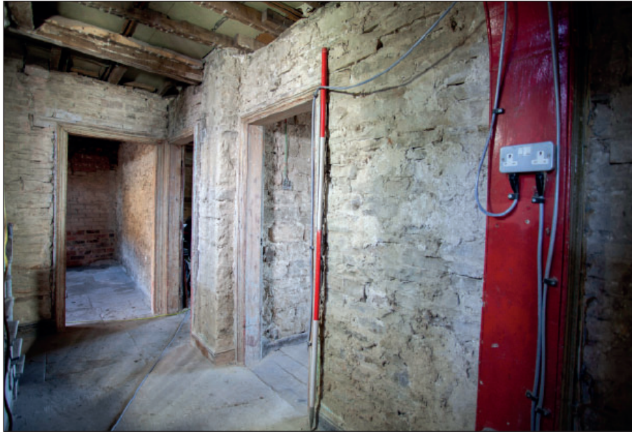
Plate 81: G8, detail of projecting wall with doorway to G6
