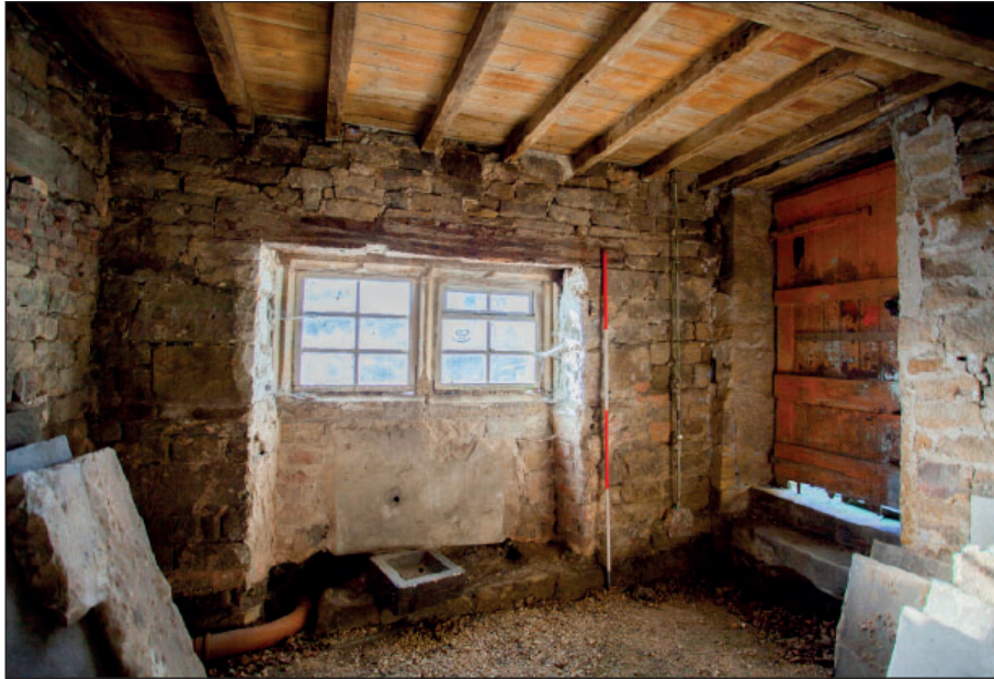
Plate 55: G2, mullioned window within the south wall and recessed lower wall
