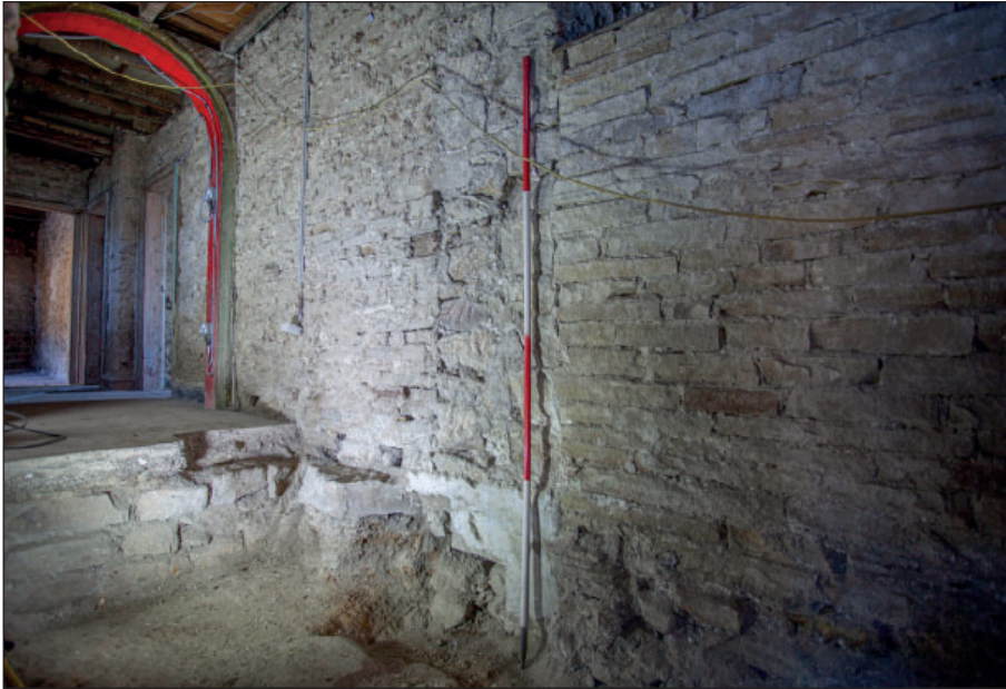
Plate 75: G8, scars of former steps within the southern end of the east wall
