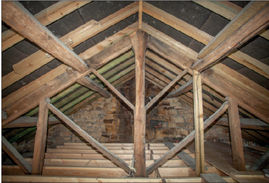
Plate 133: A2, king-post truss and staggered tenoned purlins with tusk tenon joints
