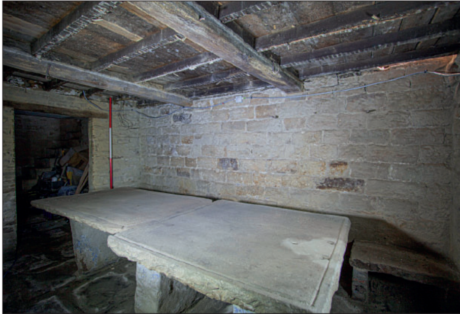
Plate 43: C1, detail of iron hooks attached to timber beams
