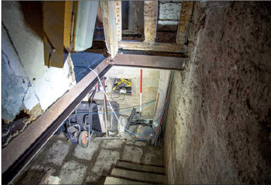
Plate 47: C2, inserted RSJ supporting the later concrete ceiling
