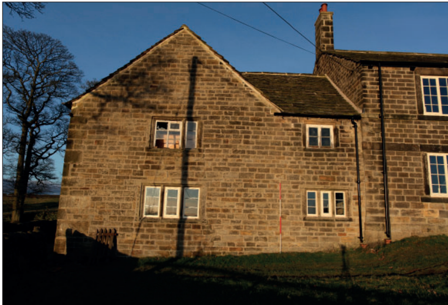
Plate 4: East elevation, detail of the Cottage façade
