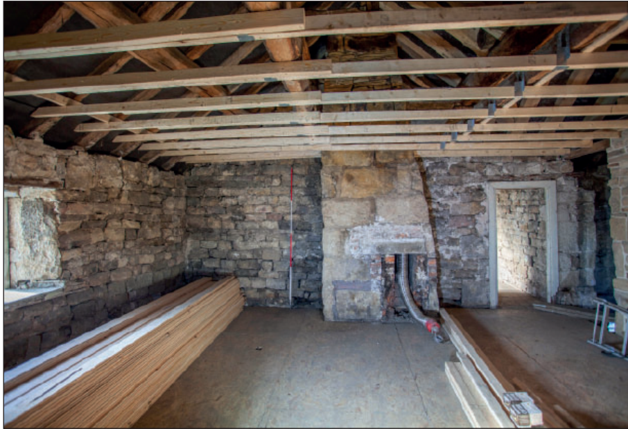
Plate 93: F1, general view of fireplace
