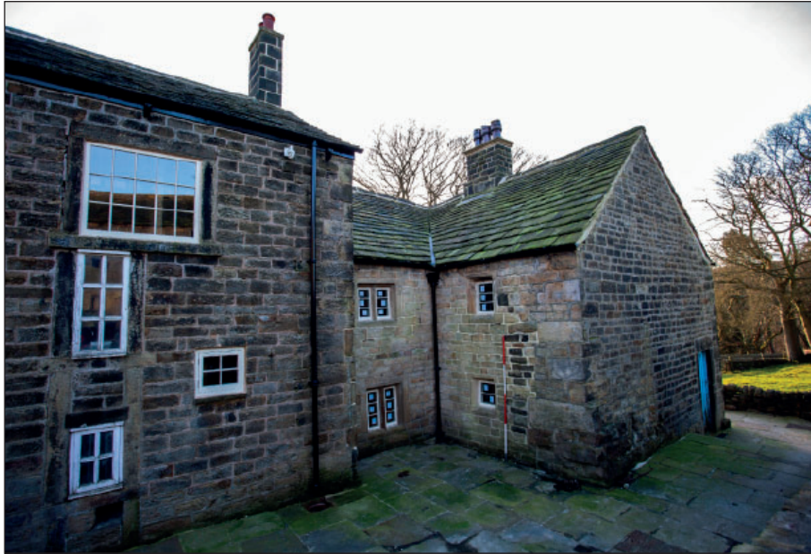
Plate 33: General view of the north elevation of the Cottage
