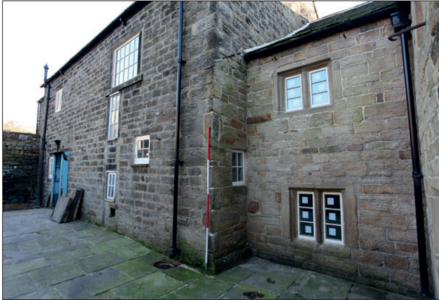
Plate 25: Detail of dressed south-western quoins of the Farmhouse
