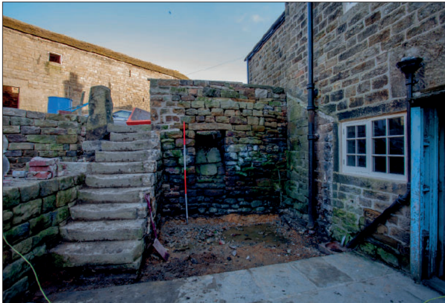
Plate 30: Partially demolished lean-to extension with coal chute
