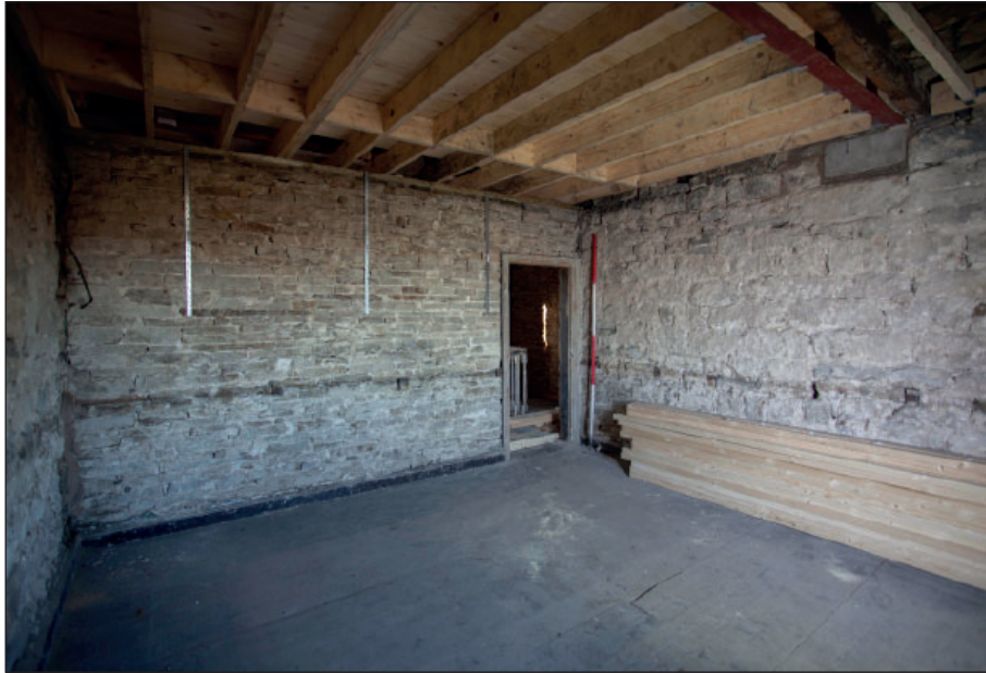
Plate 113: F4, looking north-west
