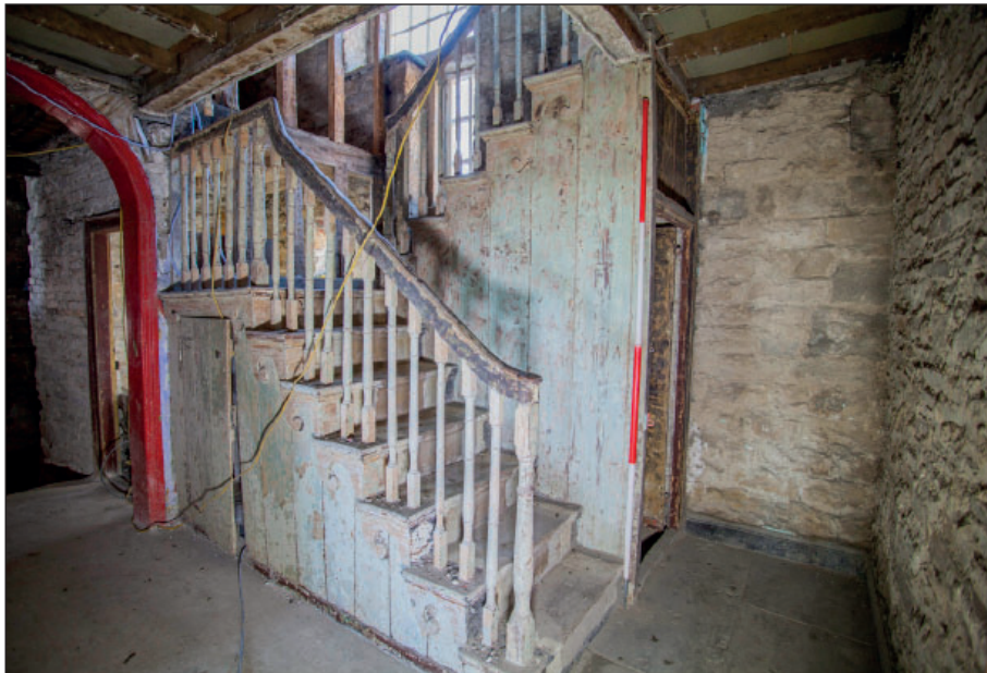
Plate 78: G8, detail of staircase
