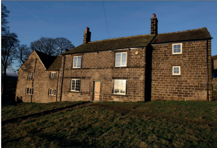
Plate 1: General view of the east elevation
