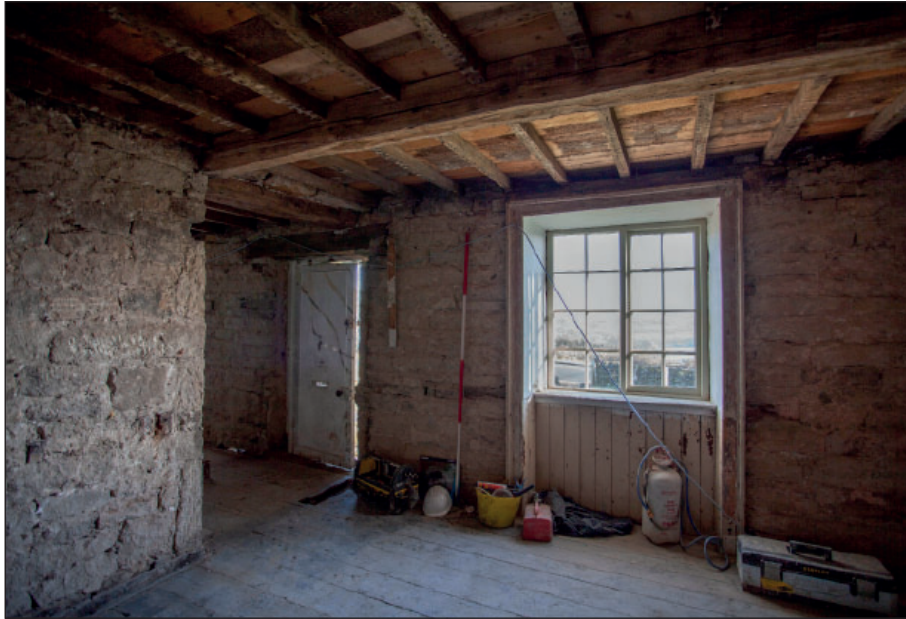
Plate 67: G5, window opening and doorway within the east wall
