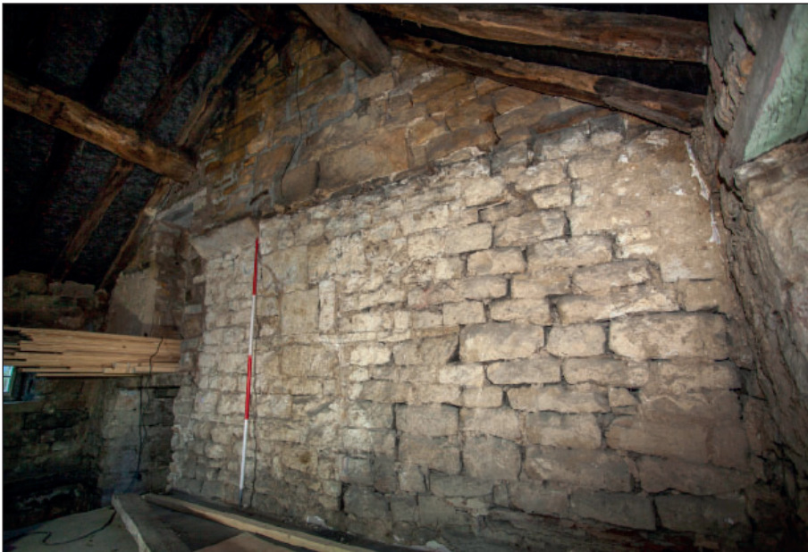
Plate 106: F3, general view of the north wall
