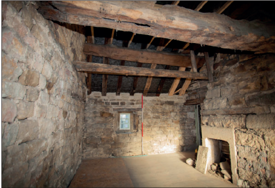
Plate 101: F2, general view of the north wall
