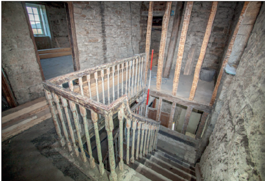
Plate 120: F7, general view of the staircase
