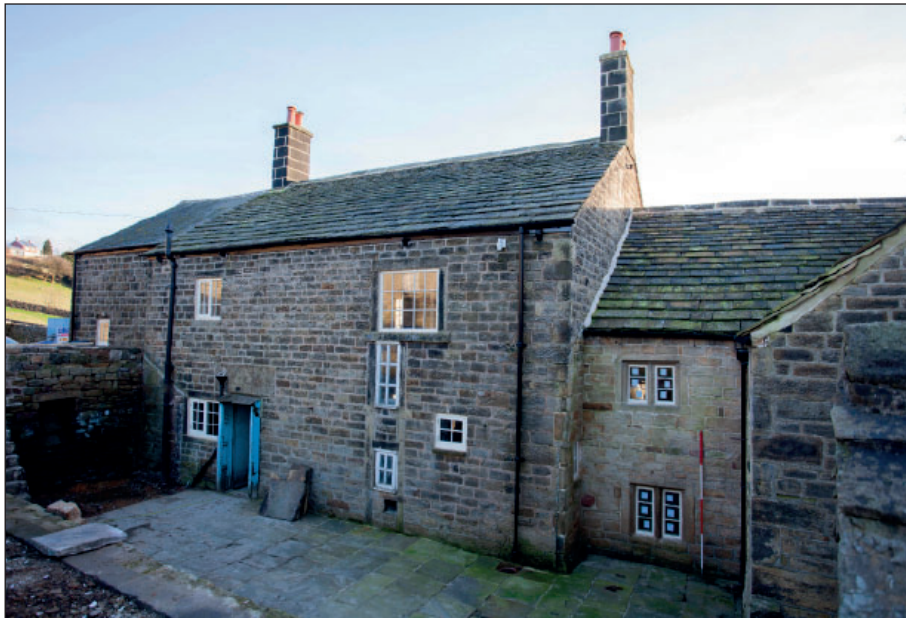
Plate 24: General view of the west elevation of the Farmhouse
