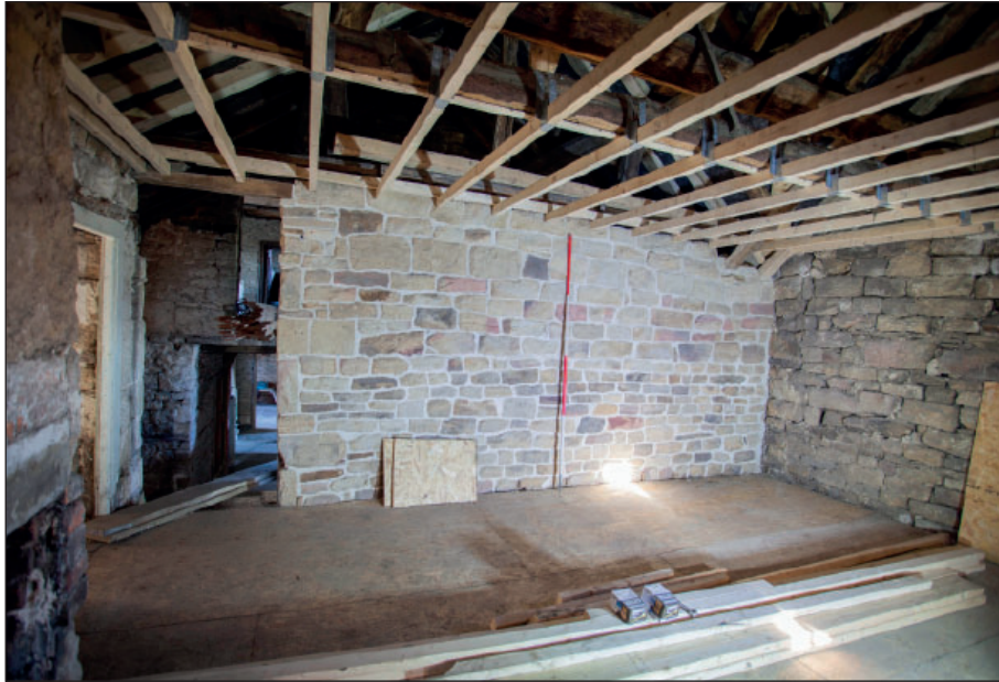
Plate 95: F1, general view of the north wall
