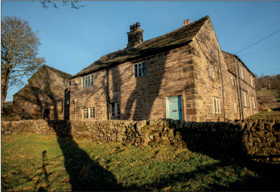
Plate 13: General view of the south and east elevations, looking north-west
