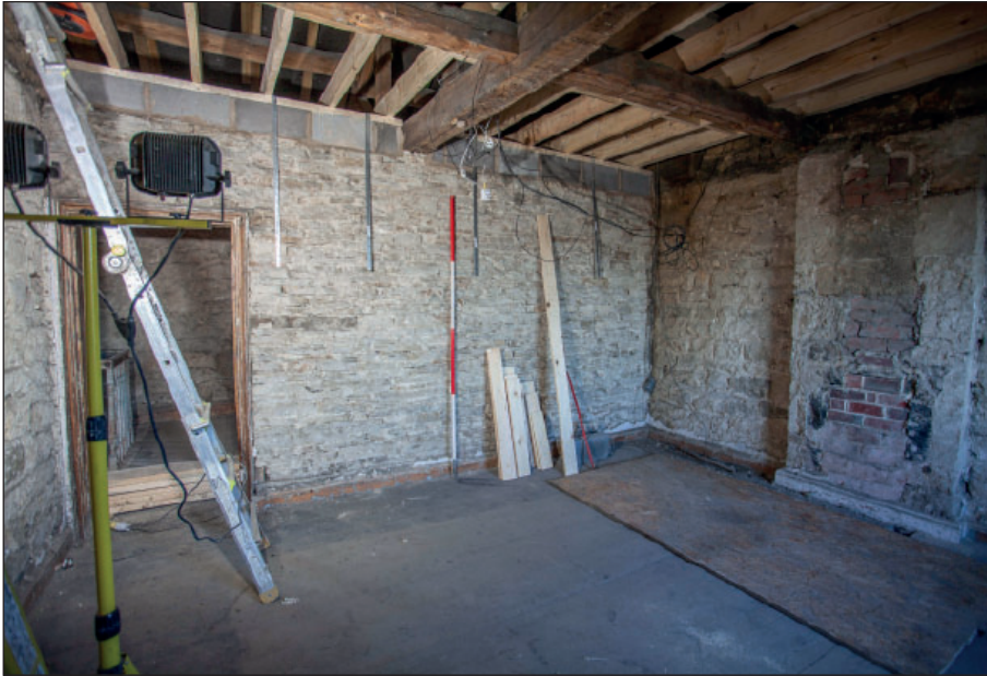
Plate 115: F5, looking north-west
