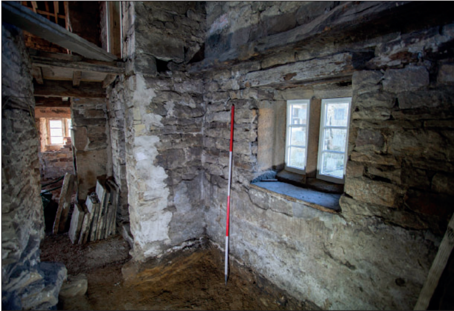
Plate 57: G3, girding beam against the west wall
