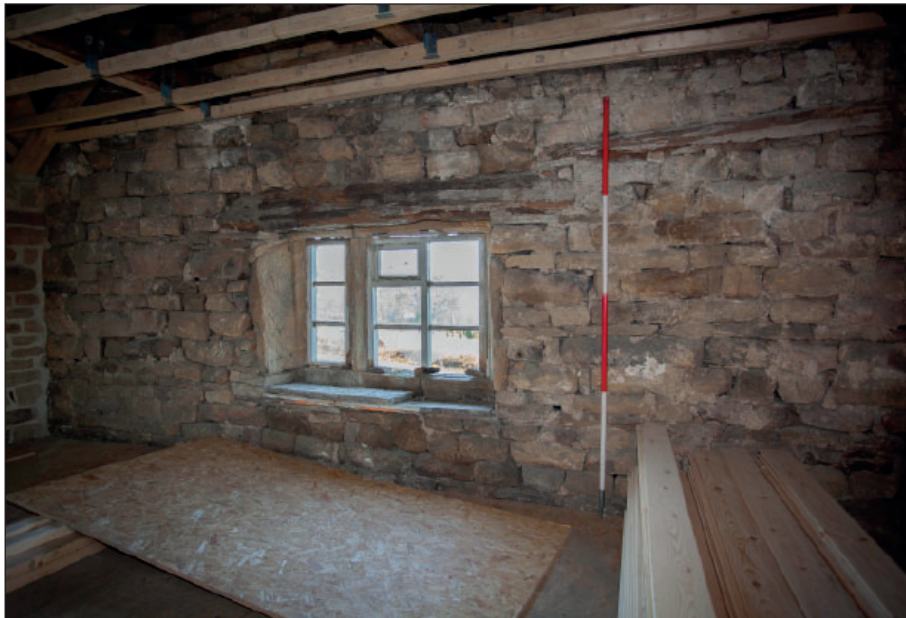
Plate 92: F1, detail of mullioned window within the east wall
