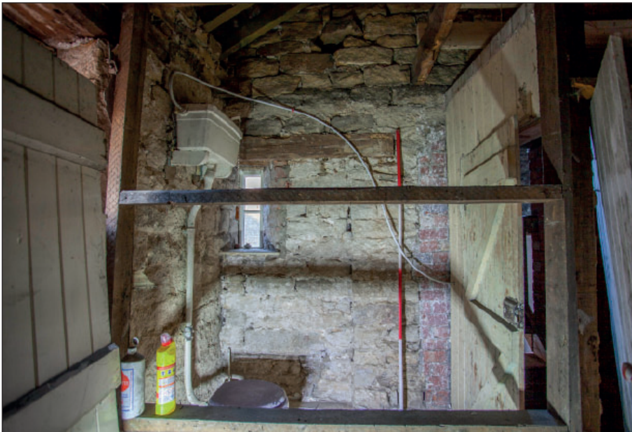
Plate 128: F9, north wall with blocked opening
