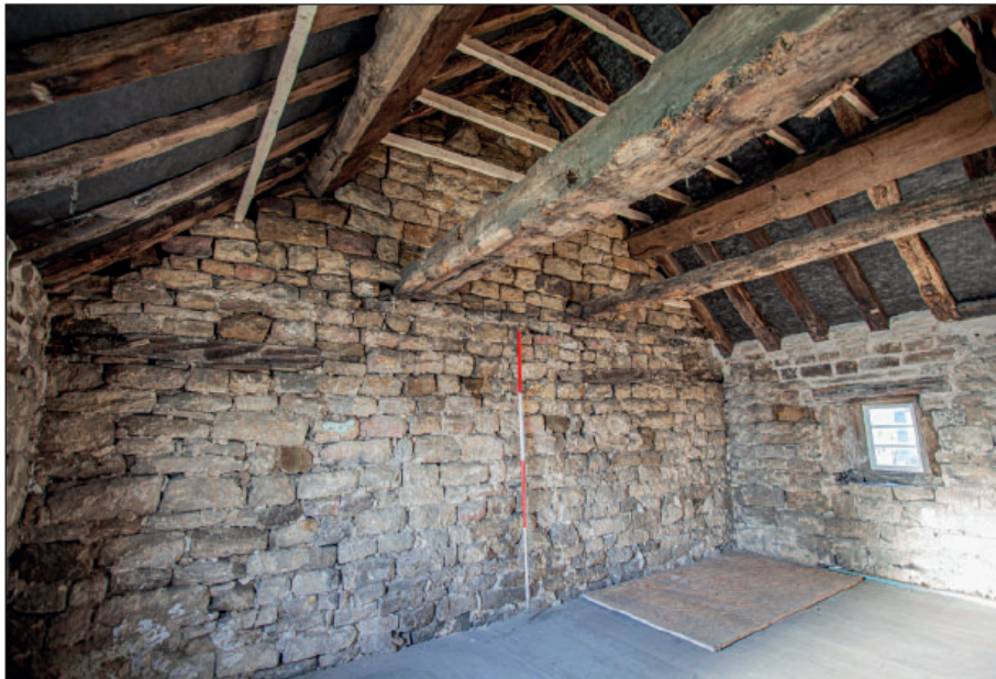
Plate 100: F2, west gable wall and roof structure
