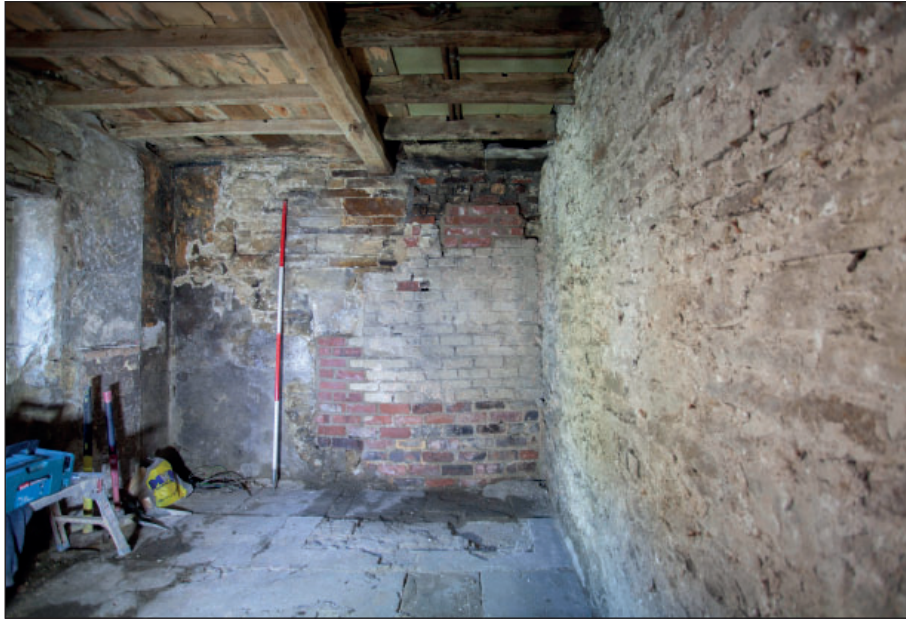
Plate 83: G9, north wall with later brickwork
