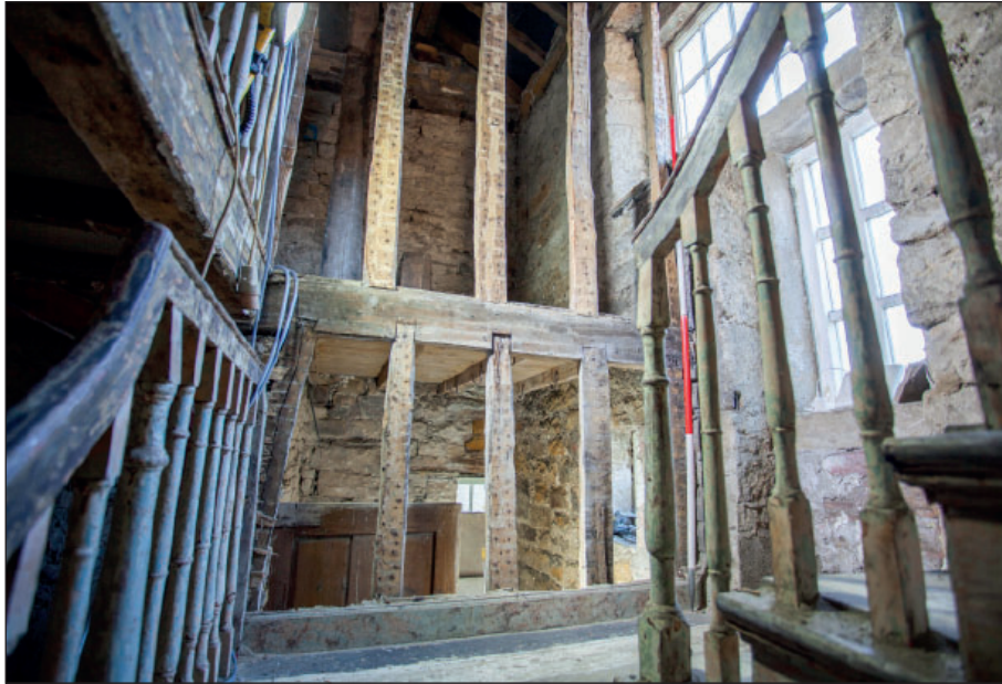
Plate 123: F7, detail of stud wall of staircase
