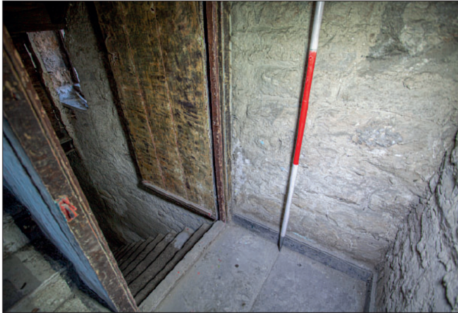
Plate 79: G8, staircase to cellar C2
