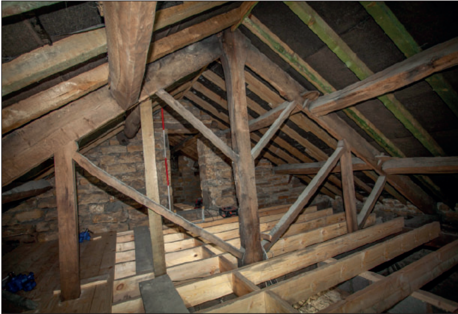
Plate 135: A2, upper face of truss with assembly carpenter marks 'II'
