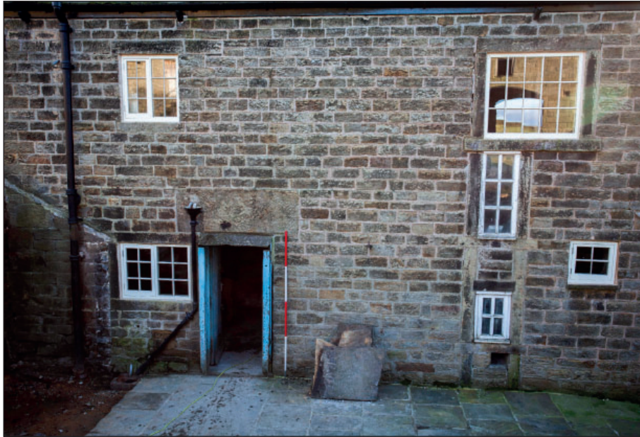
Plate 27: West elevation, detail of the Farmhouse rear façade
