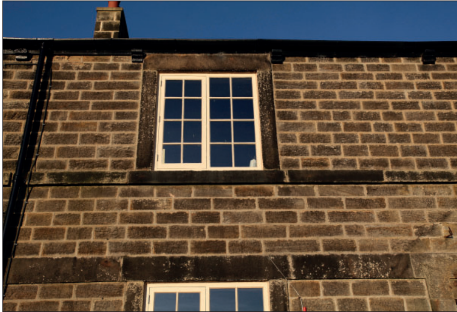
Plate 11: East elevation, detail of dressed string bands and window architrave
