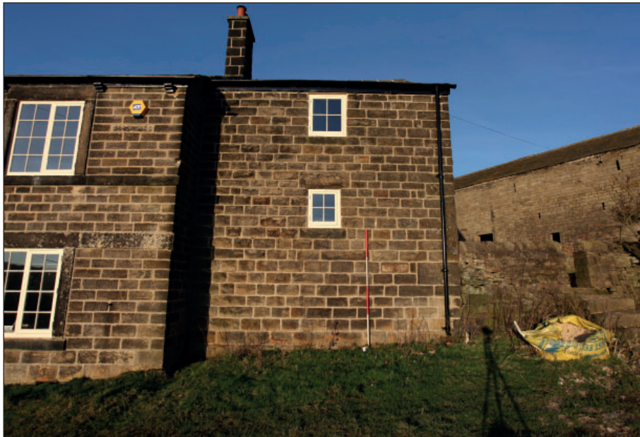
Plate 12: East elevation, northern extension
