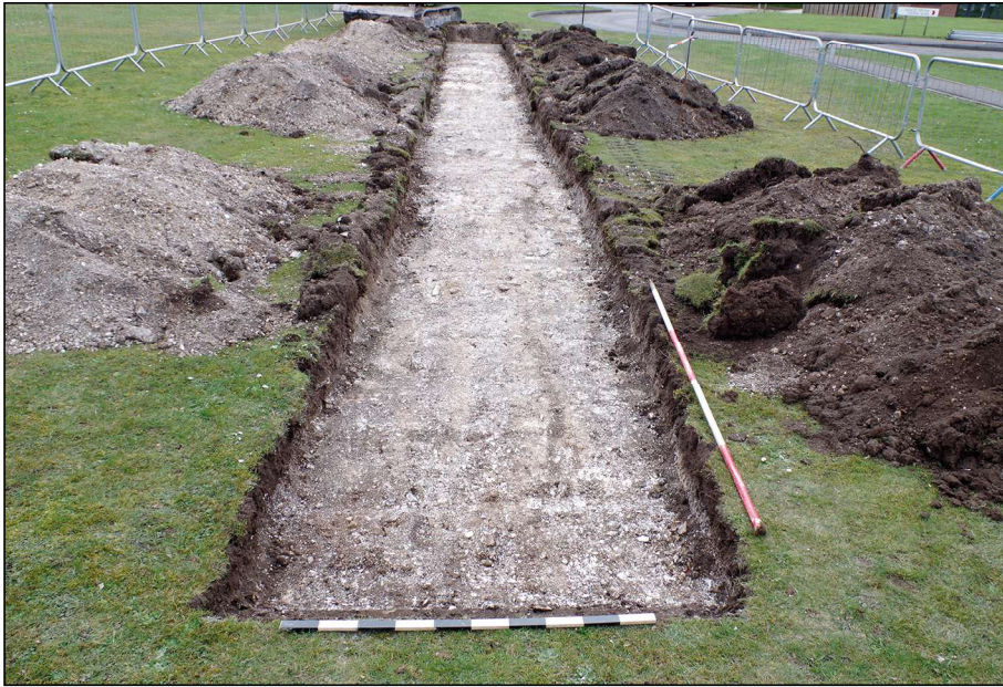
Plate 1: Trench 152 looking south-east
