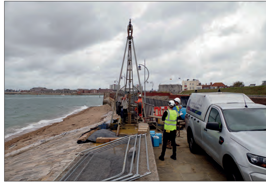
Plate 2: Location of Trench 2, View from the south-east
