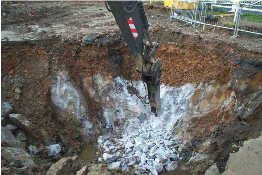
Plate 1: Groundworks for Receiving Hopper from the east
