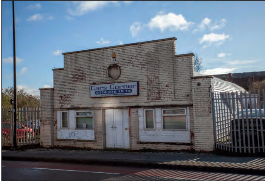
Plate 35: Building 3 - detail of front elevation
