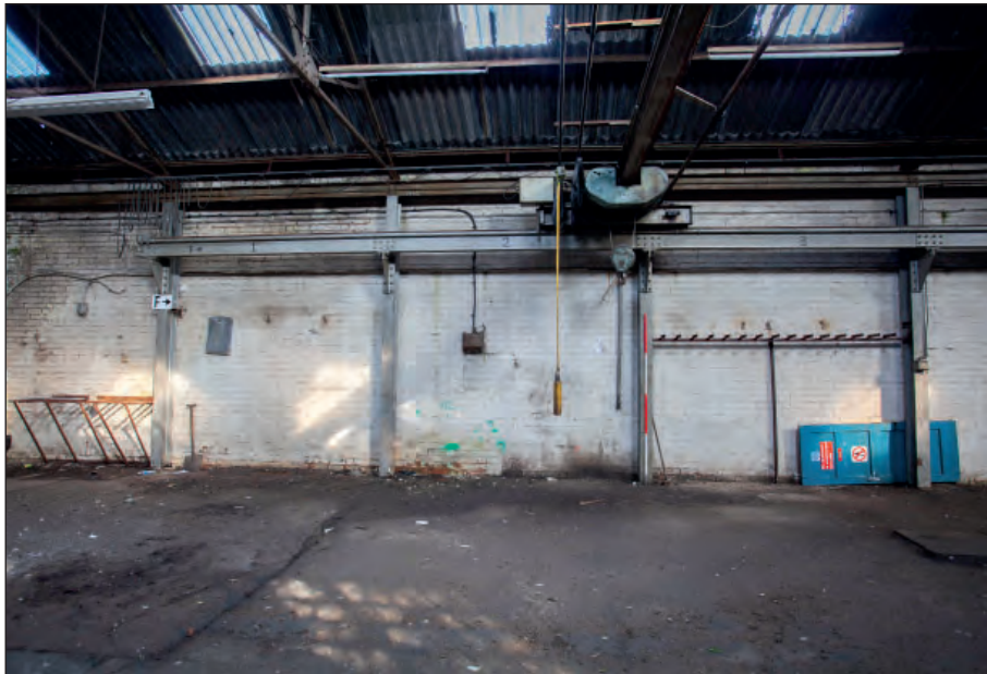
Plate 7: Building 1 - north-east wall and overhead travelling crane gantry
