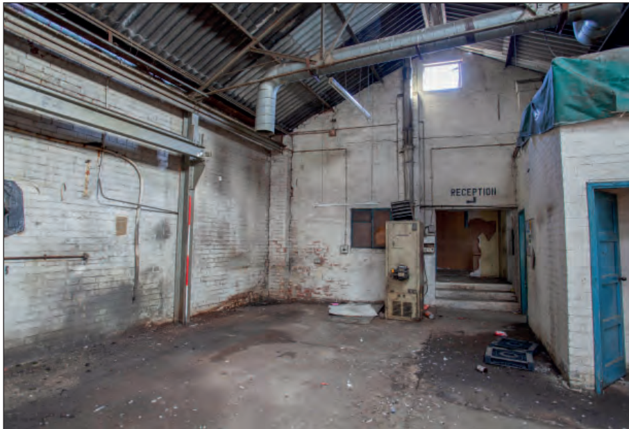
Plate 10: Building 1 - south-east end of warehouse
