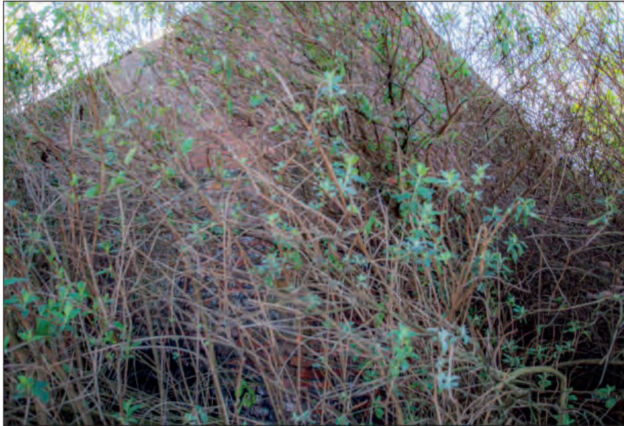
Plate 23: Building 2 - north-west gable wall with earlier lower brickwork
