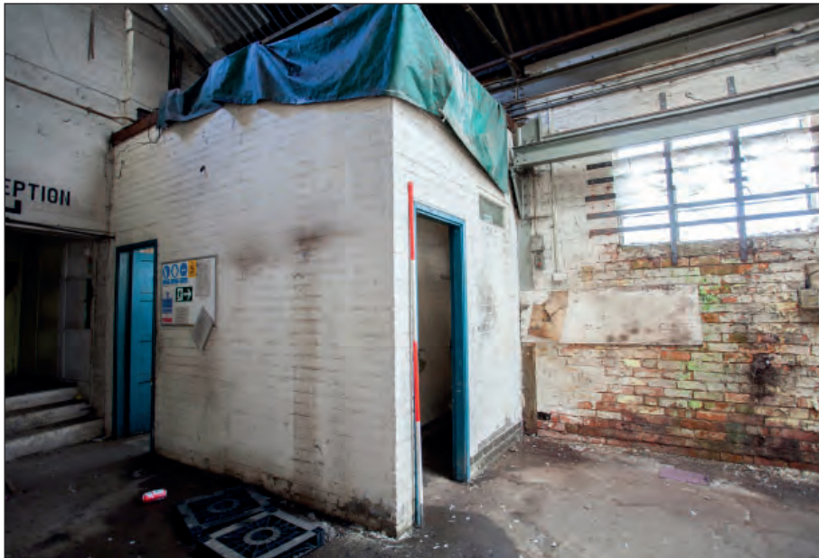
Plate 12: Building 1 - toilet and kitchen block
