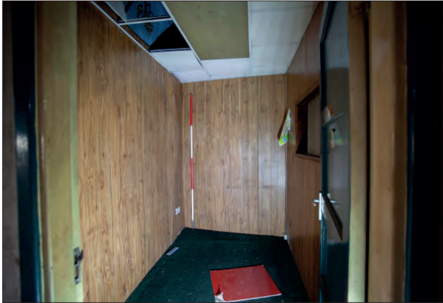
Plate 15: Building 1 - office 1 within the south-eastern range
