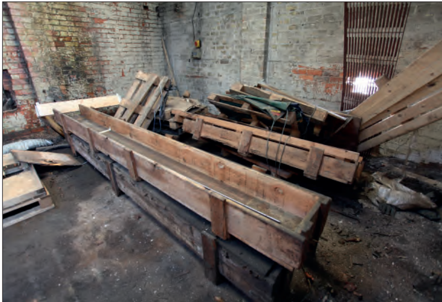
Plate 33: Building 2 - G2 detail of wooden boxes
