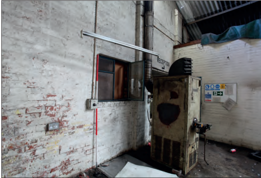
Plate 11: Building 1 - detail of former external window within the south-eastern range
