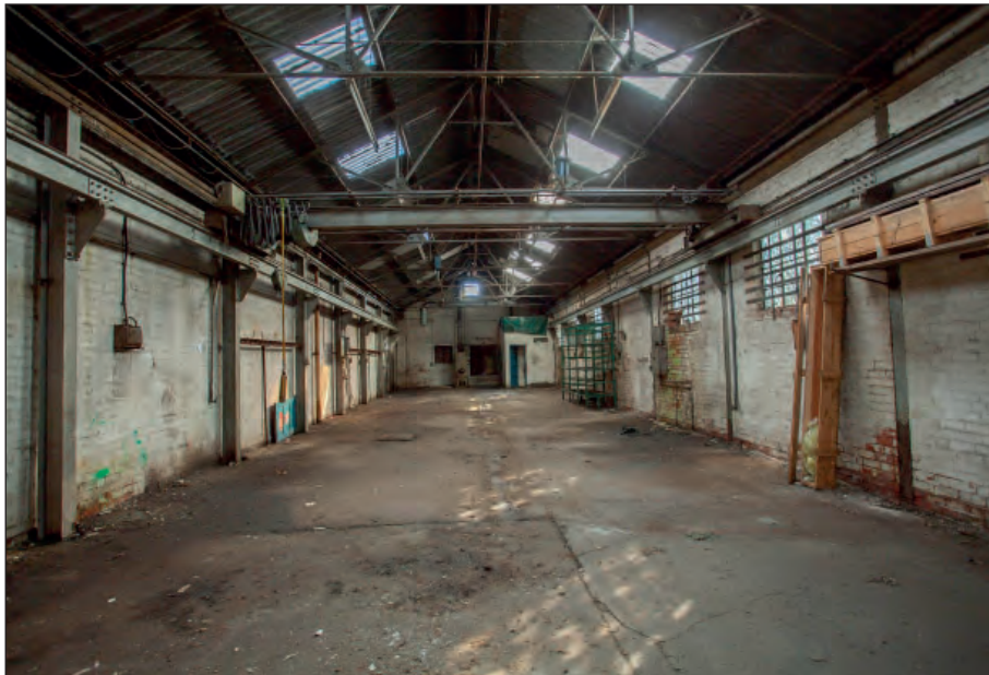
Plate 4: Building 1 - general internal view of warehouse
