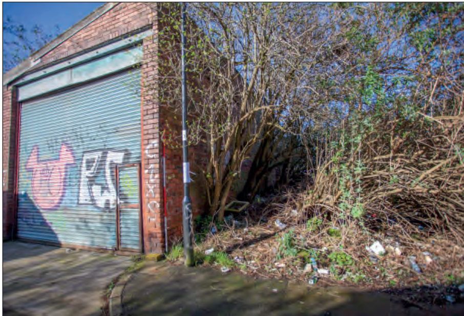
Plate 22: Building 2 - doorway with roller shutter and north-east elevation
