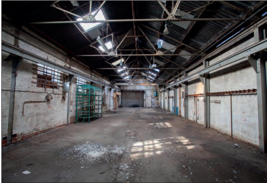
Plate 9: Building 1 - general view of warehouse, looking north-west
