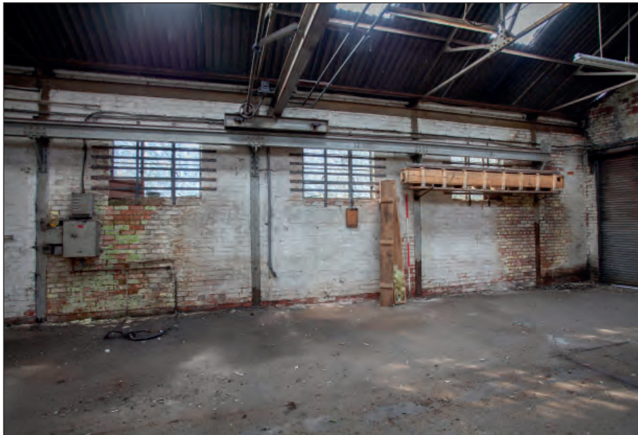
Plate 6: Building 1 - south-west wall with steel stanchions, brick infill and windows
