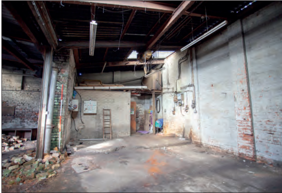
Plate 25: Building 2 - G1 with later office inserted to the north-west
