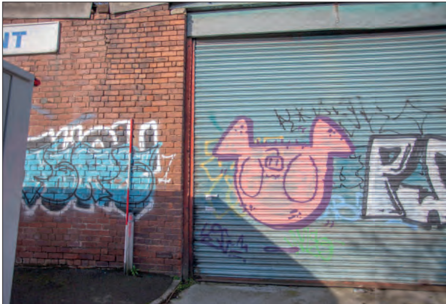
Plate 20: Building 2 - detail of construction joint
