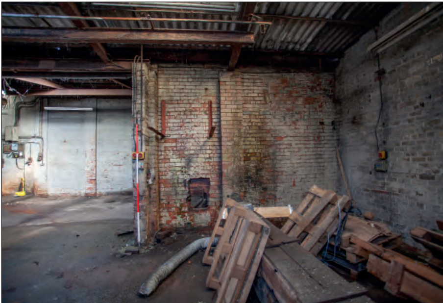
Plate 32: Building 2 - G2 wall brackets
