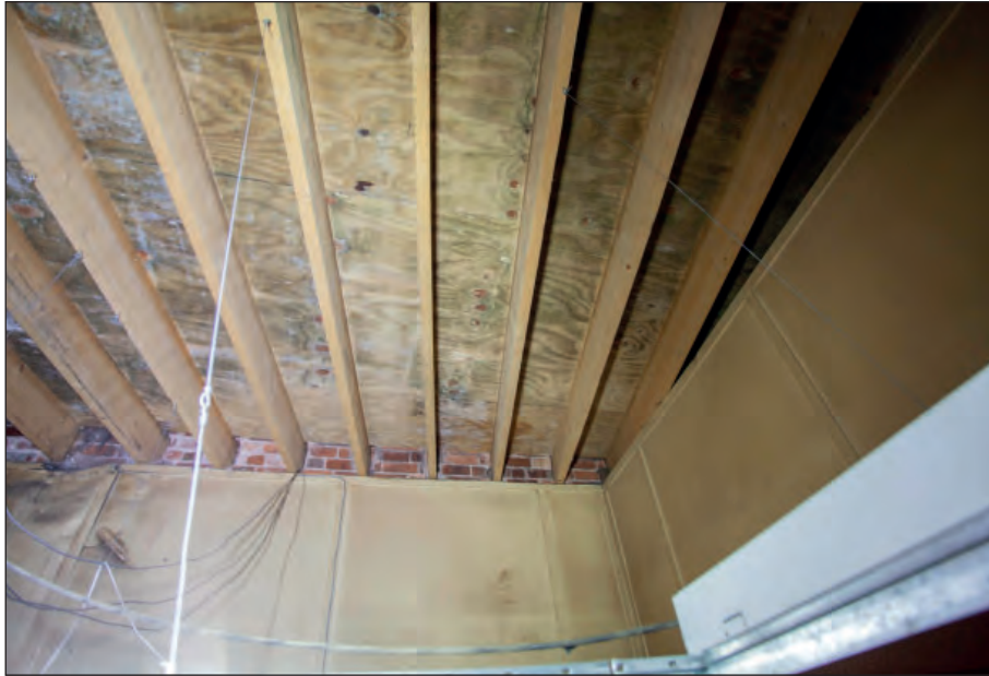
Plate 17: Building 1 - roof structure above false ceiling of office 2
