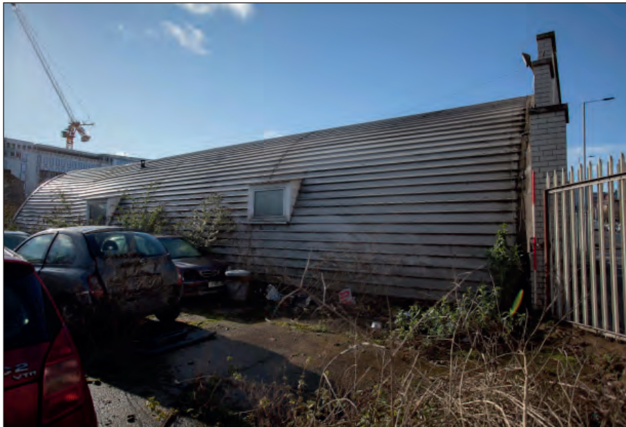
Plate 40: Building 3 - north-east elevation
