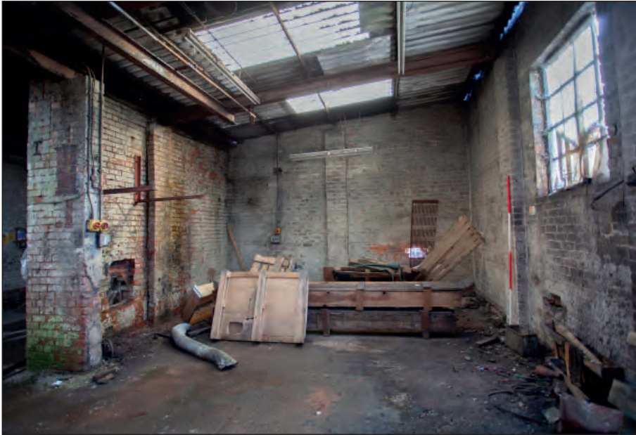
Plate 31: Building 2 - south-east end of G2
