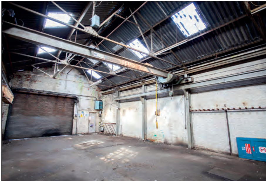
Plate 8: Building 1 - detail of crane gantry
