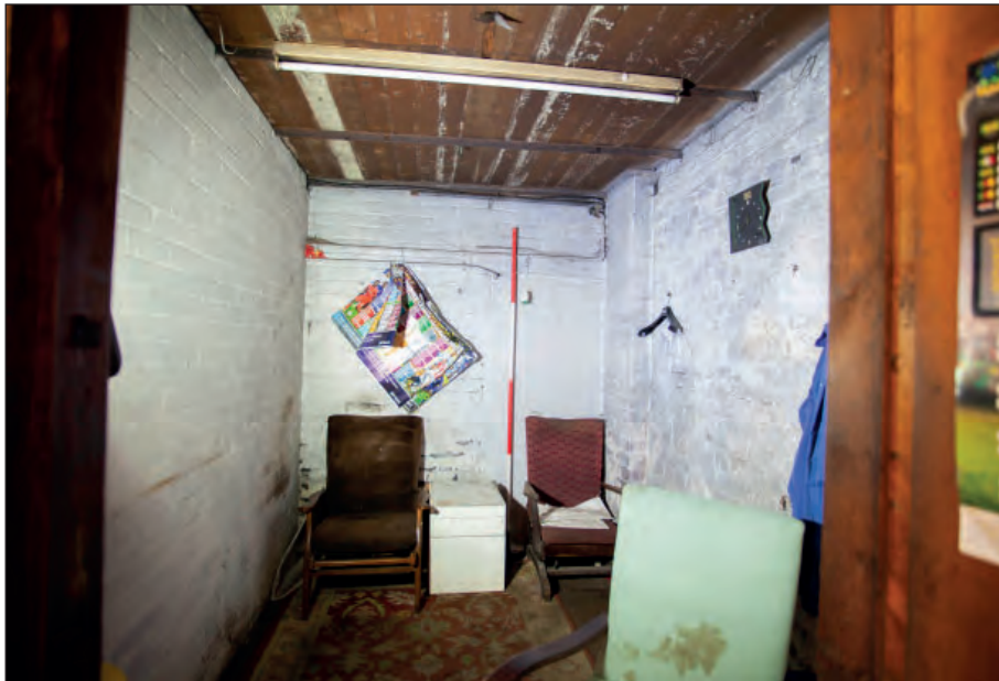
Plate 28: Building 2 - inside office with blocked doorway to the south-west
