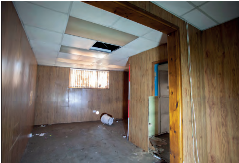
Plate 16: Building 1 - office 2 within the south-eastern range
