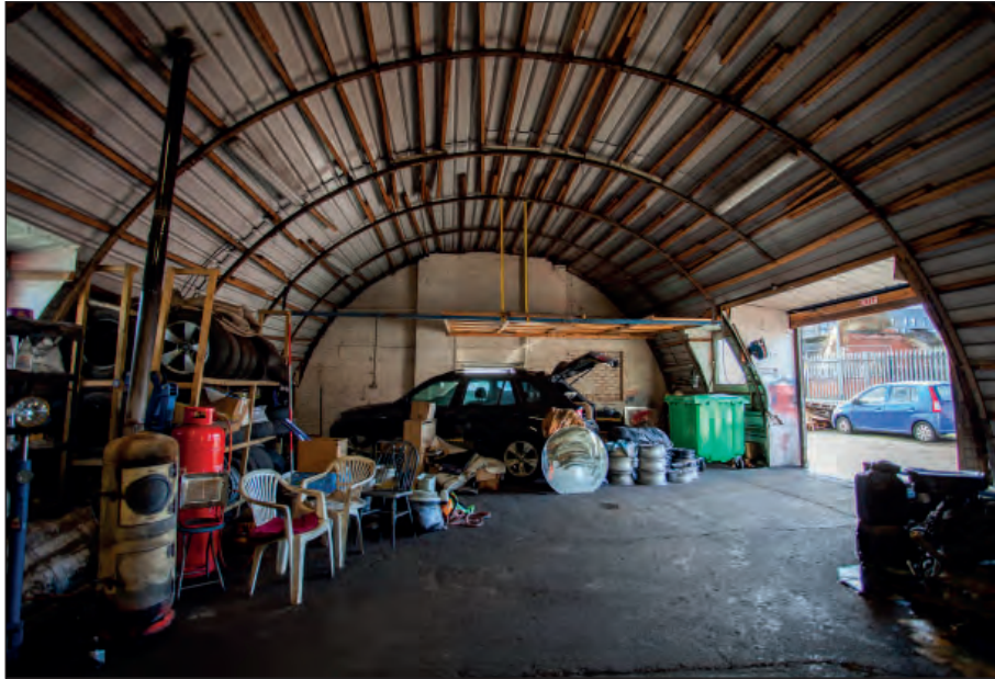
Plate 41: Building 3 - internal view of workshop, looking south-east
