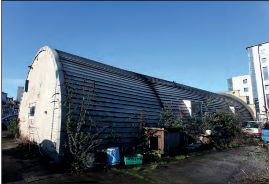
Plate 39: Building 3 - general view of the north-east elevation
