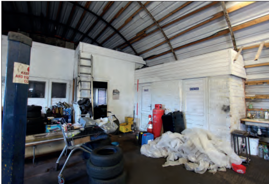
Plate 43: Building 3 - inserted toilets and office
