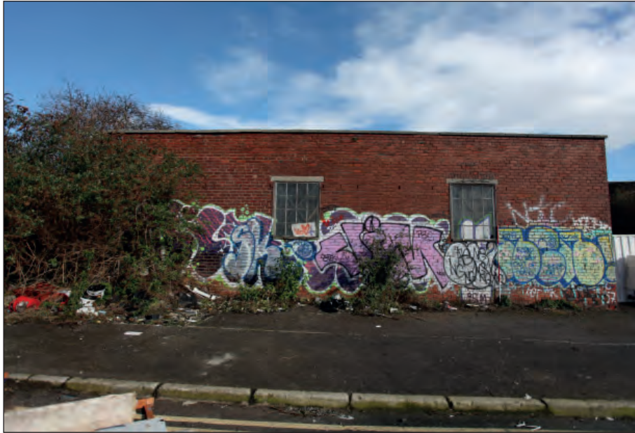
Plate 21: Building 2 - south-west elevation
