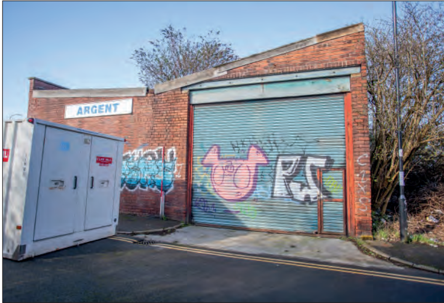
Plate 19: Building 2 - front elevation facing Matthew Street
