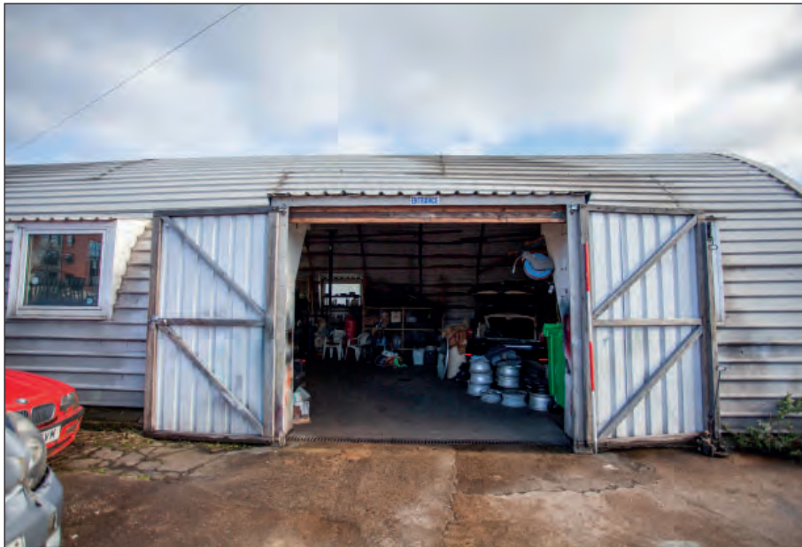
Plate 38: Building 3 - doorway within the south-west elevation
