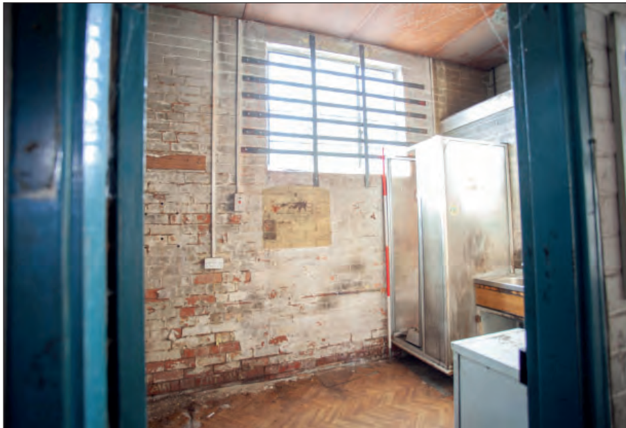
Plate 14: Building 1 - kitchen room
