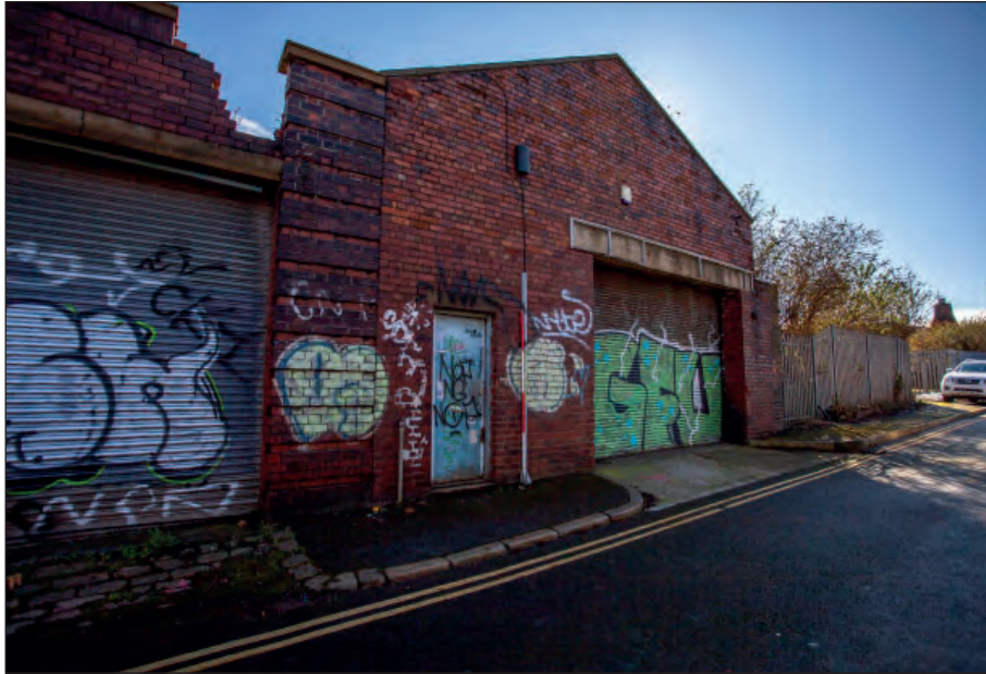
Plate 1: General view of Building 1, looking south
