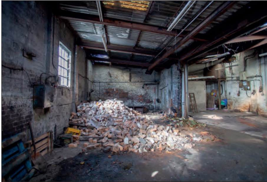
Plate 29: Building 2 - G2 with a pile of firebricks
