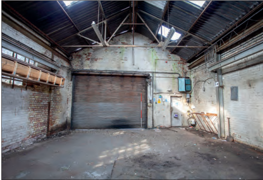
Plate 5: Building 1 - north-west end of warehouse
