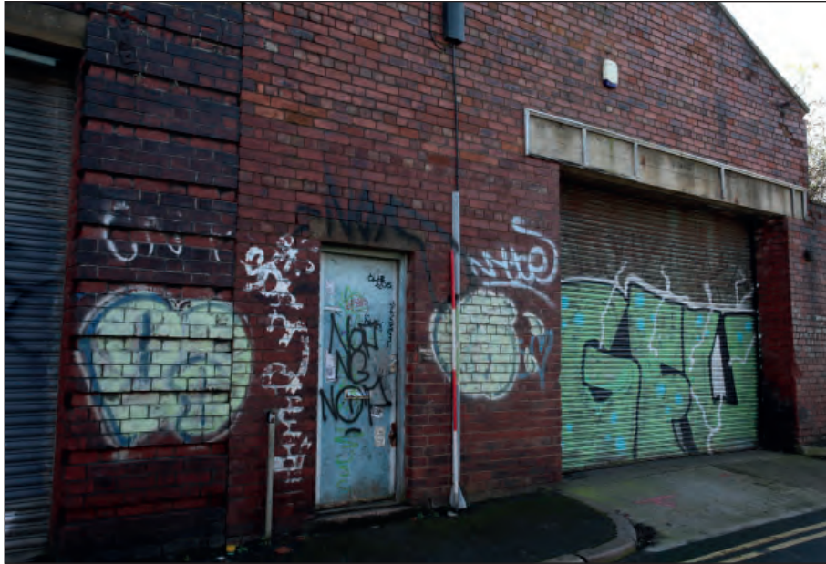
Plate 3: Building 1 - detail of external doorways
