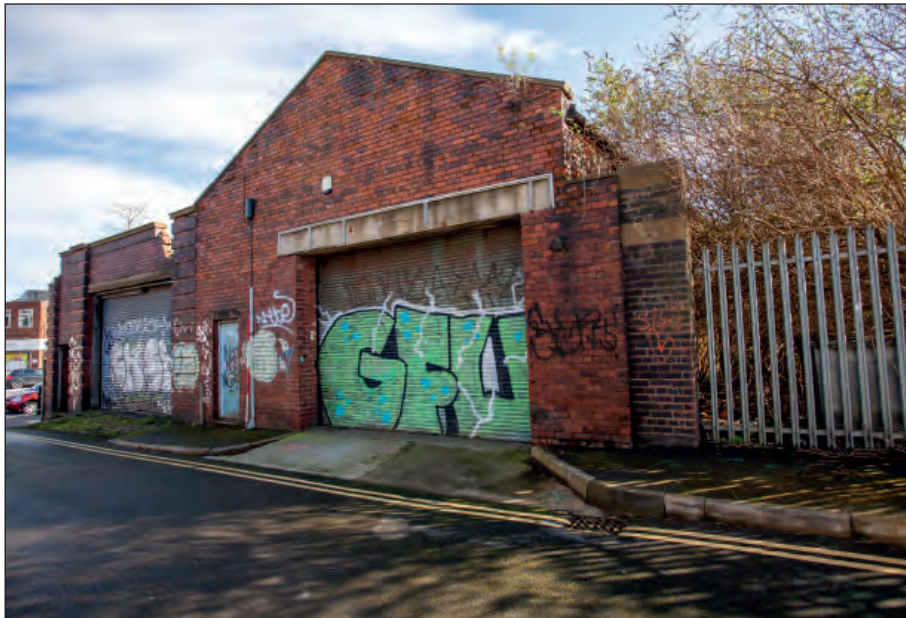
Plate 2: Front elevation of Building 1 adjacent to the former Shalesmoor Warehouse
