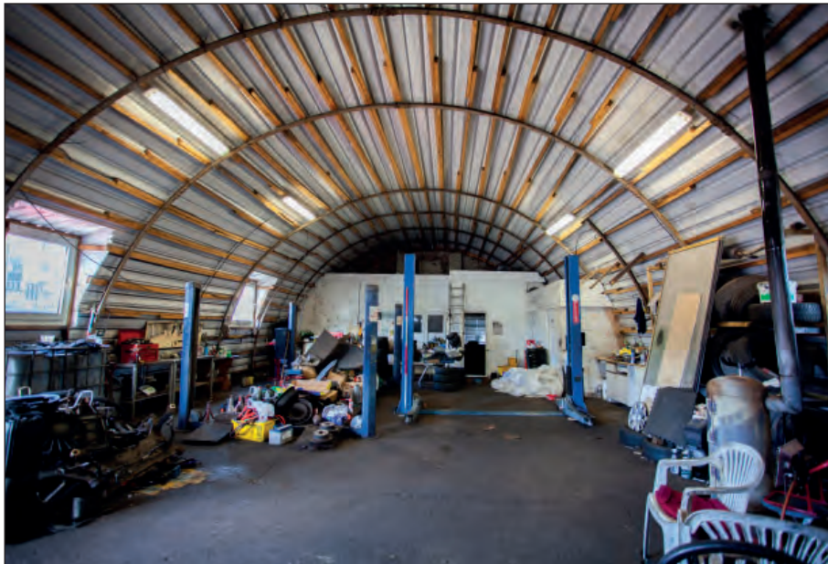
Plate 42: Building 3 - workshop, looking north-west
