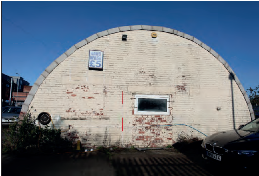
Plate 36: Building 3 - rear elevation
