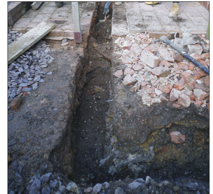
Plate 5: Working shot of foundation trench excavations, photographed from the south-west
