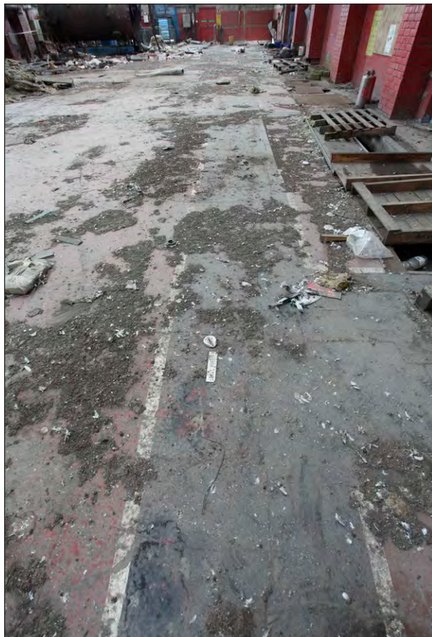
Plate 14: Powerhouse, principal room, demarcated walkway, facing southeast
