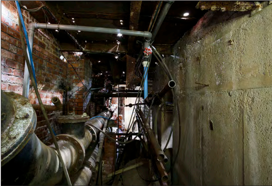
Plate 27: Powerhouse, example of pipe duct, facing southeast
