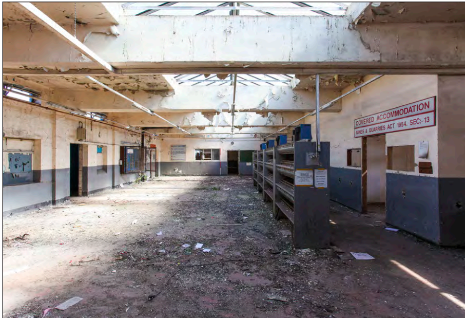
Plate 67: Lamp Room, first floor, overview of main room, facing northeast
