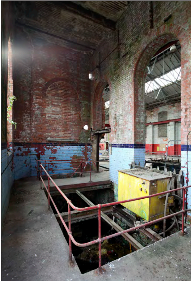
Plate 3: Powerhouse, lobby overview, facing south
