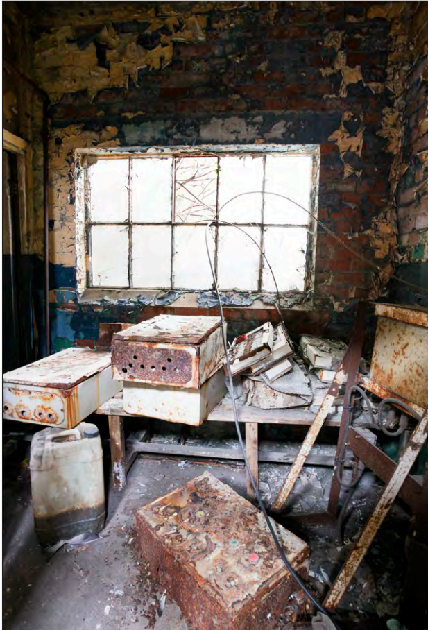
Plate 19: Powerhouse, storage room overview, facing southeast
