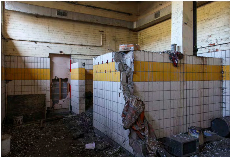
Plate 52: Pithead Baths, ground floor , shower room within northeast section, facing east
