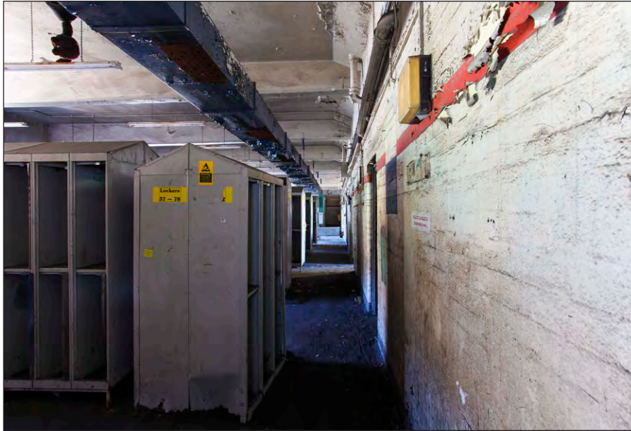
Plate 41: Pithead Baths, ground floo , clean locker room, facing northeast
