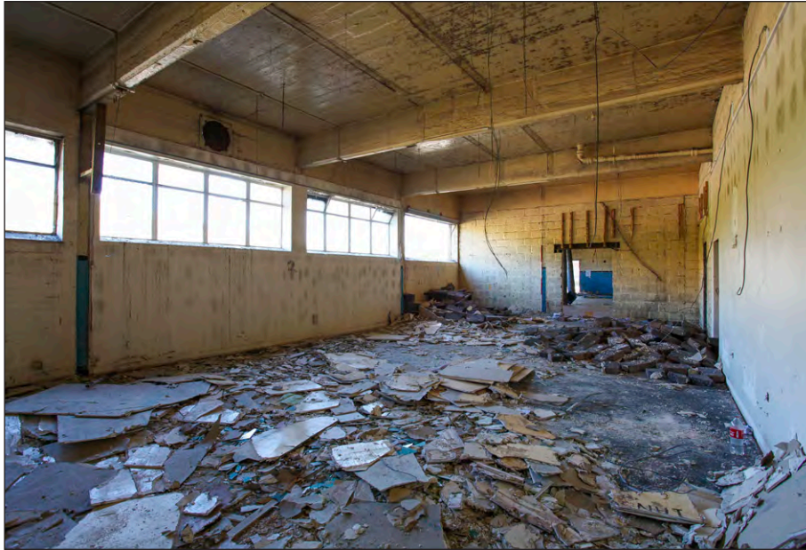
Plate 35: Pithead Baths, first floor, converted clean locker room, facing north
