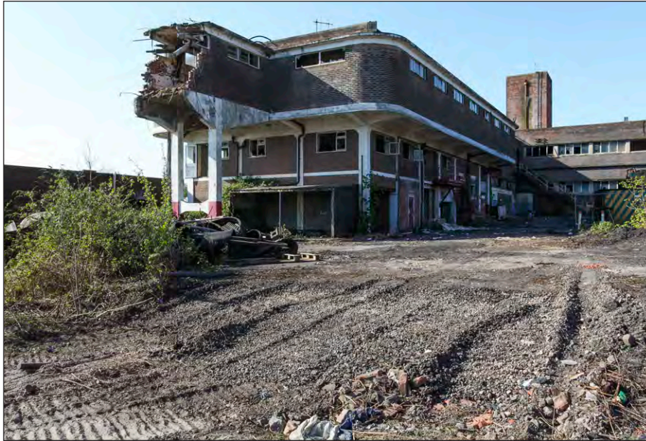
Plate 57: Lamp Room, northeast and northwest elevations
