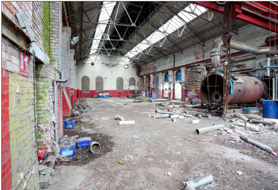
Plate 6: Powerhouse, principal room overview, facing north
