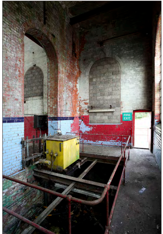
Plate 4: Powerhouse, lobby overview, facing west
