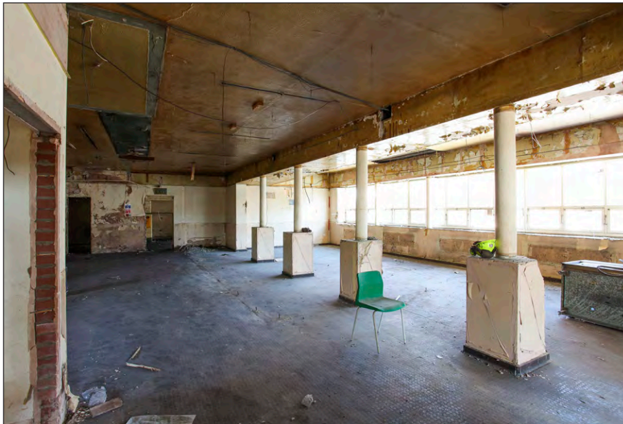
Plate 74: Canteen, overview, facing east
