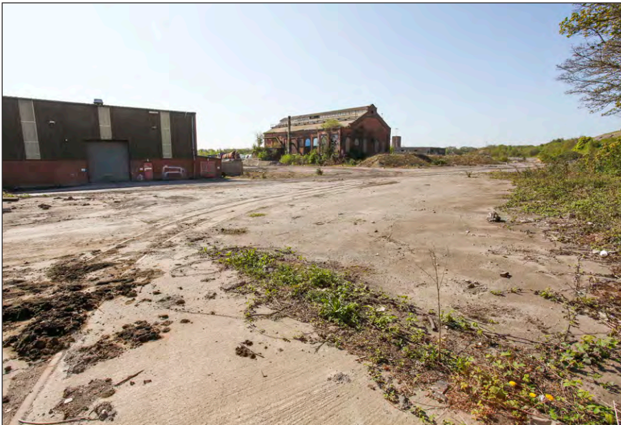
Plate 84: Railway sidings running southwest from the Loco Shed
