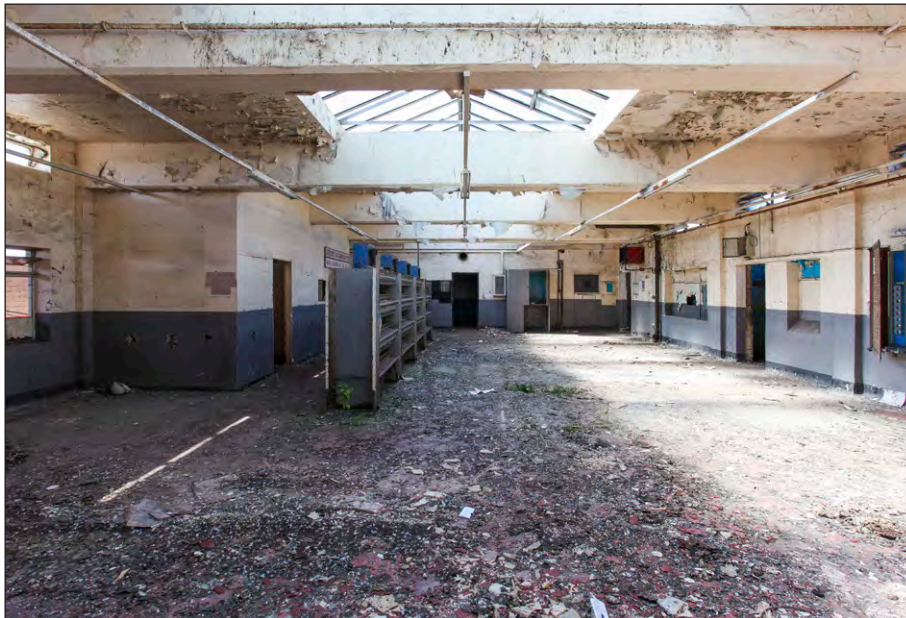
Plate 68: Lamp Room, first floor, overview of main room, facing southwest
