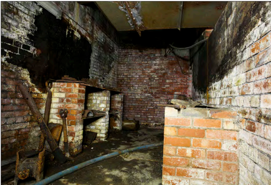
Plate 28: Powerhouse, cellar storage room, facing southeast
