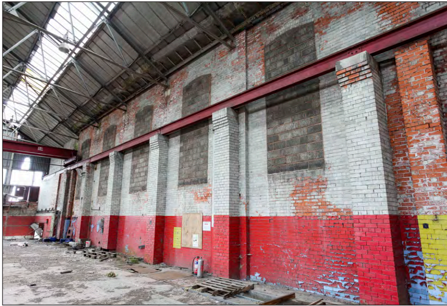
Plate 11: Powerhouse, principal room, brick pilasters and traveling train girder
