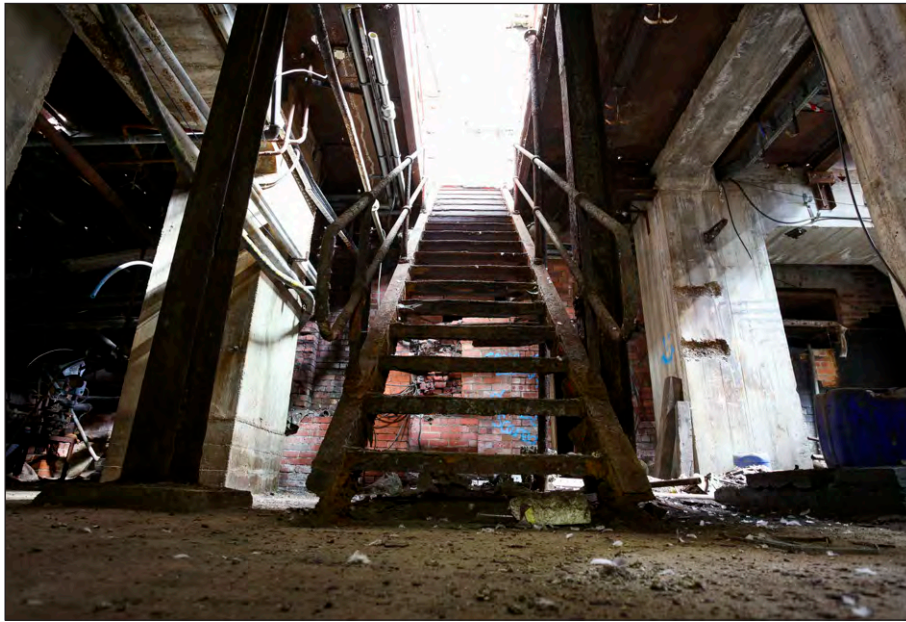
Plate 23: Powerhouse, cellar stairs to principal room, facing southeast
