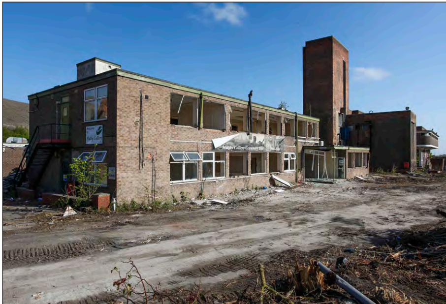
Plate 76: Main Office Building, southwest and southeast elevations
