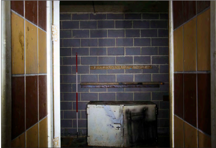
Plate 39: Pithead Baths, first floor, inserted stores within former showers, facing southwest
