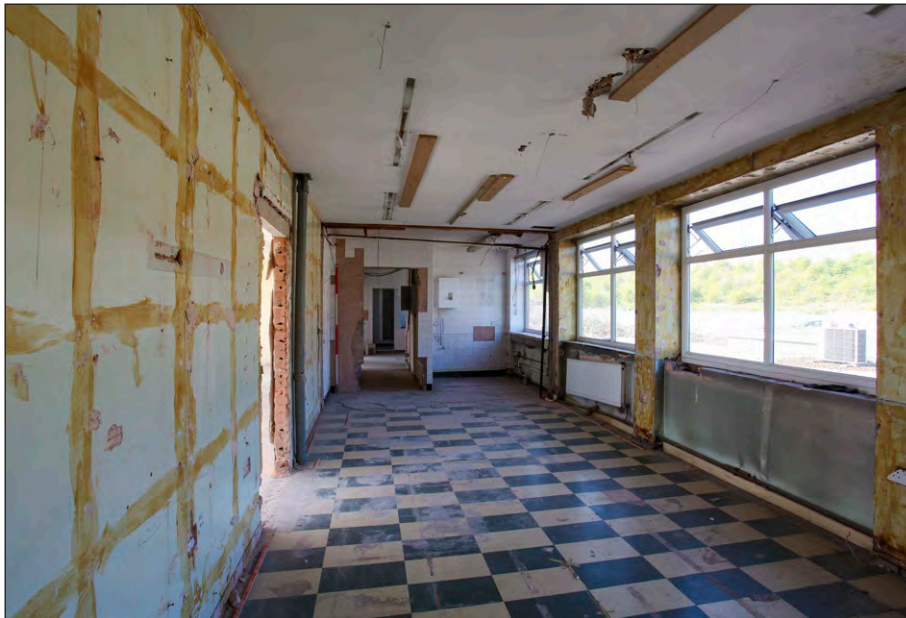
Plate 78: Main Office Building, example first floor room, facing south
