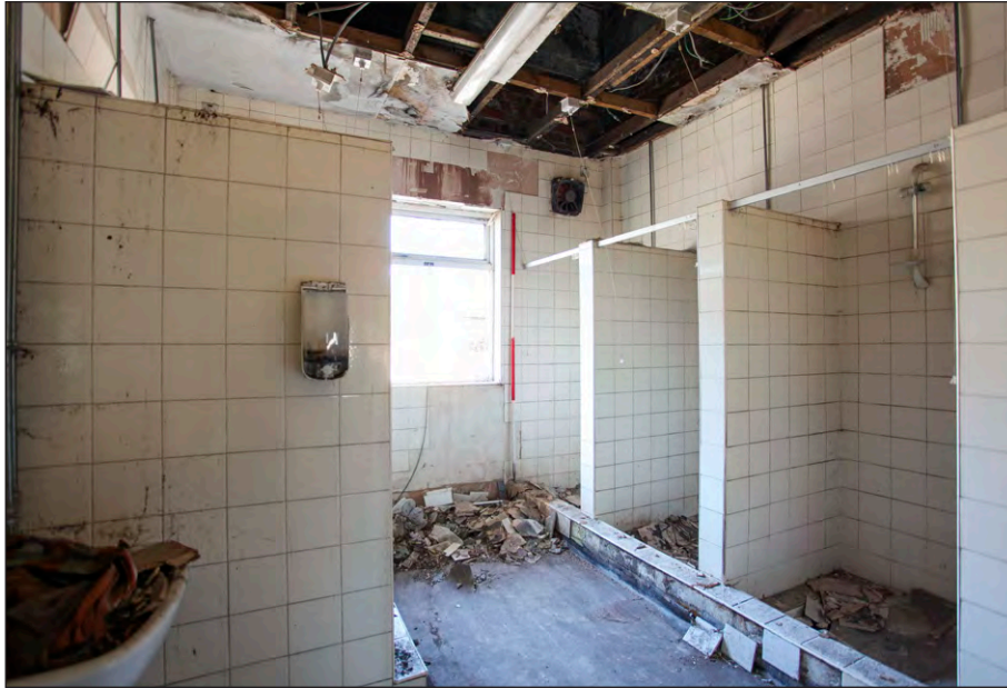
Plate 61: Lamp Room, modern showers, facing north
