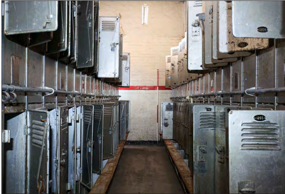
Plate 43: Pithead Baths, ground floor , original lockers in clean locker room, facing northwest
