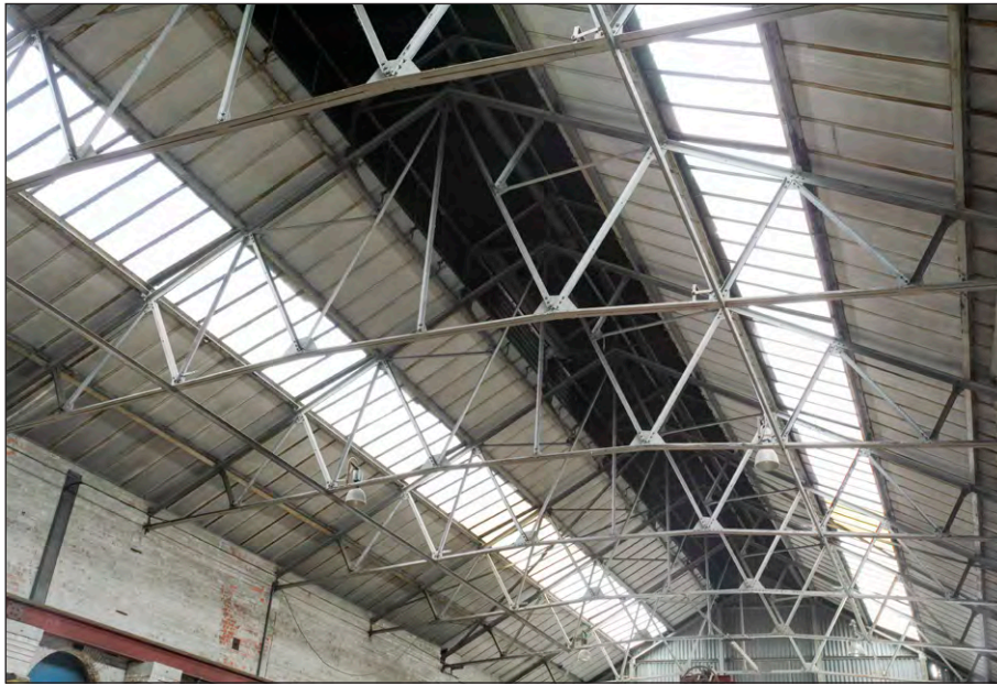
Plate 17: Powerhouse, principal room, roof detail
