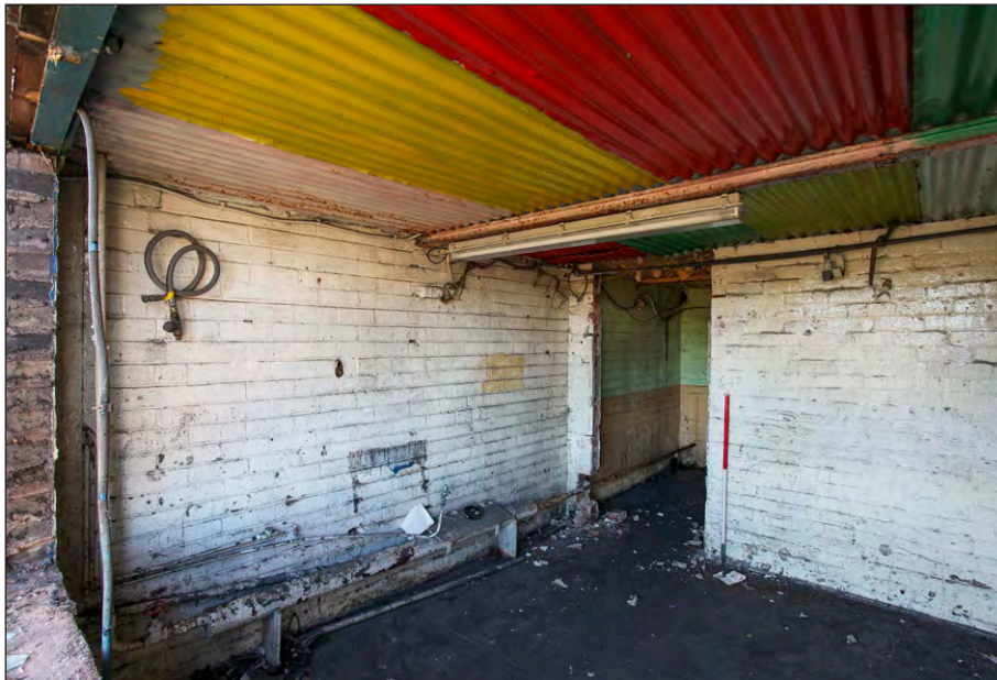
Plate 60: Lamp Room, ground floo , store, facing west
