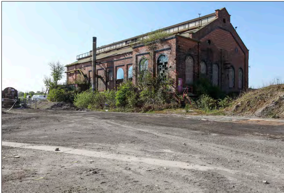
Plate 2: Powerhouse, northeast and northwest elevations
