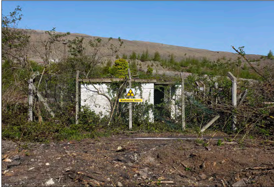
Plate 81: Radioactive Store, southeast elevation
