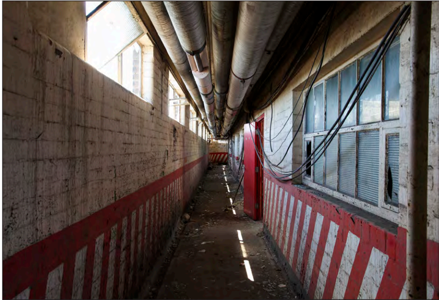
Plate 69: Lamp Room, first floor, east corridor of Lamp Room, facing southwest
