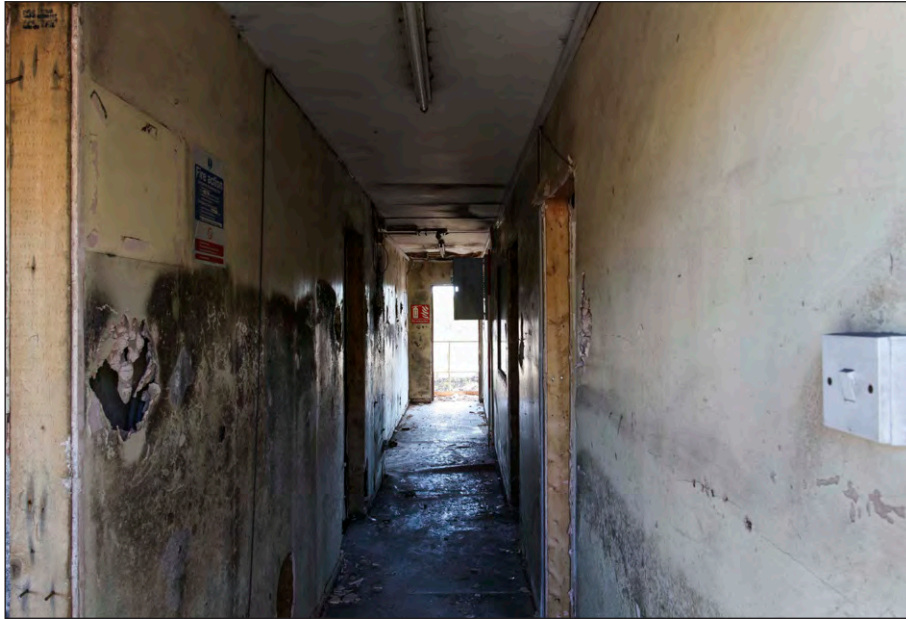
Plate 63: Lamp Room, mezzanine floor corrido , facing southeast
