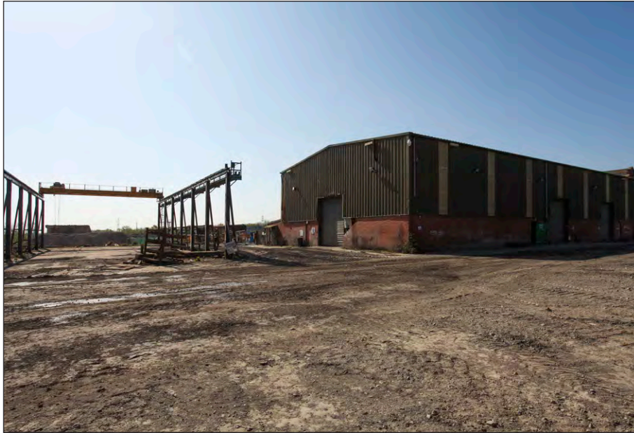
Plate 89: Former Workshop, northwest and northeast elevations
