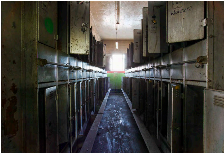
Plate 44: Pithead Baths, ground floor , original lockers in dirty locker room, facing northeast
