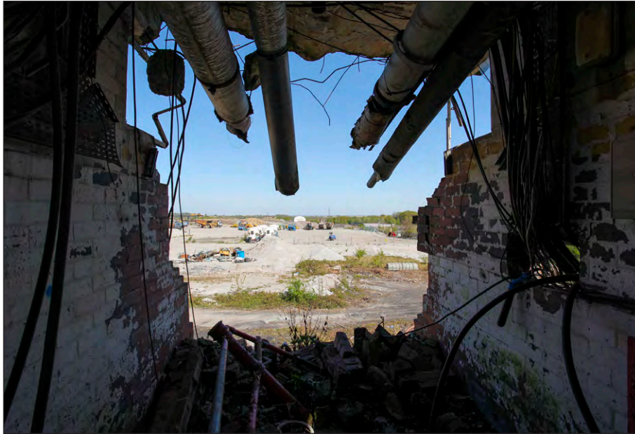
Plate 65: Lamp Room, first floor, truncated walkway, facing northeast
