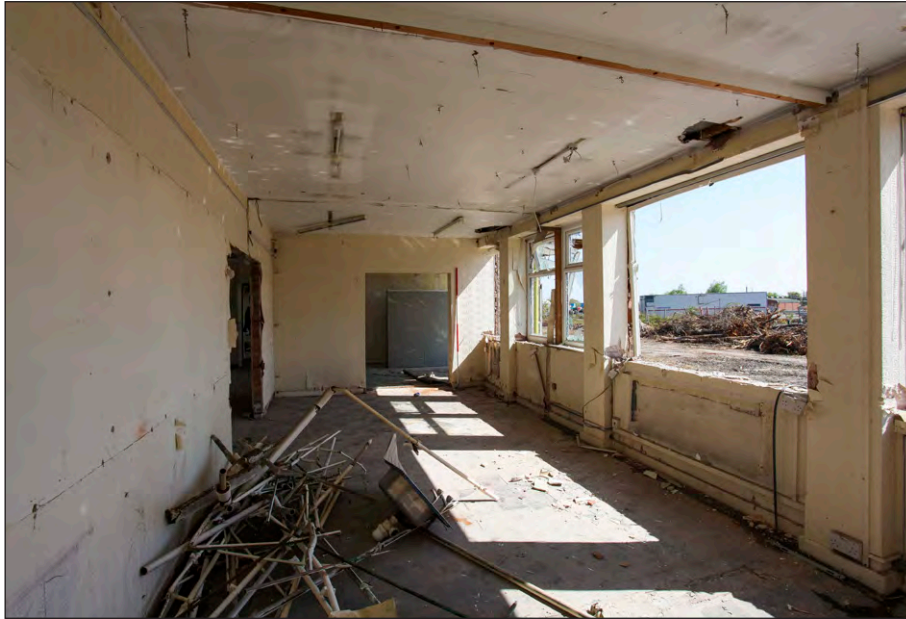
Plate 77: Main Office Building, example ground floor room, facing north
