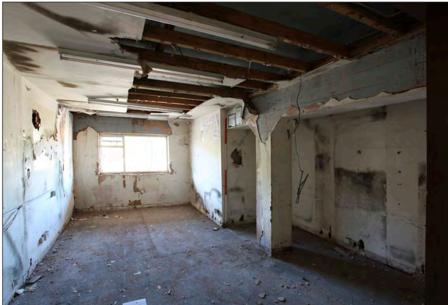
Plate 64: Lamp Room, mezzanine floo , room, facing northwest
