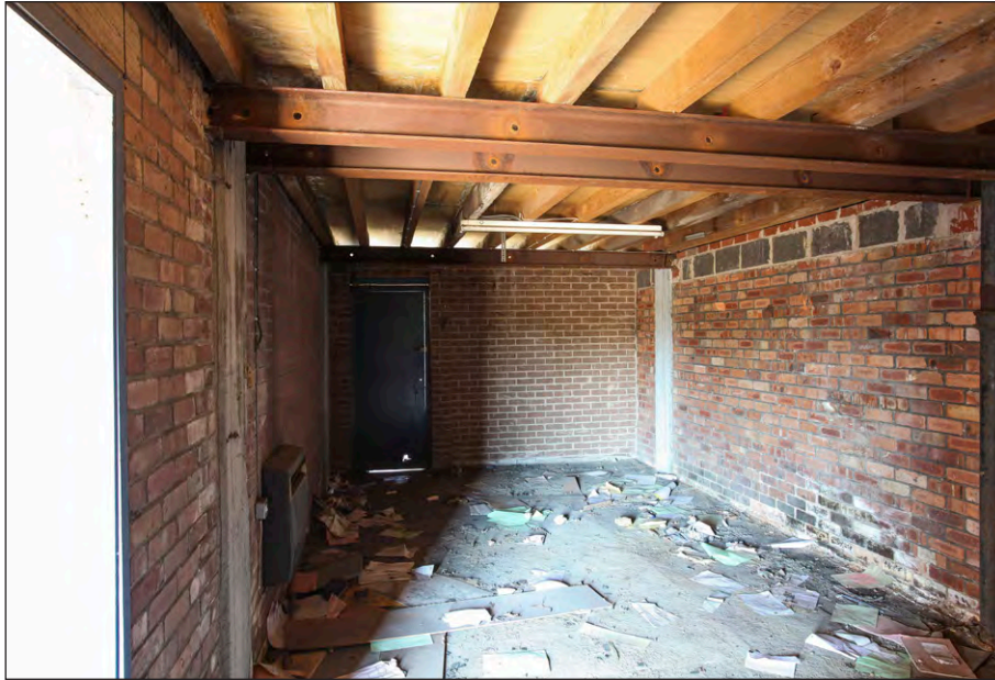
Plate 59: Lamp Room, ground floo , rescue room, facing northwest
