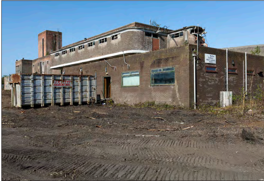
Plate 79: Control Room, northeast and southeast elevations
