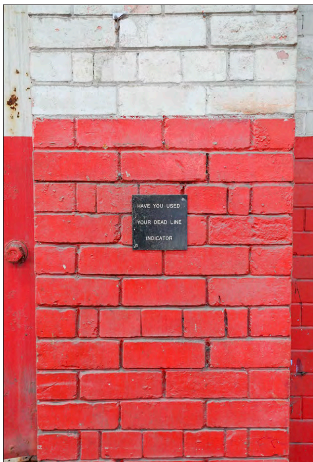
Plate 15: Powerhouse, principal room, signage
