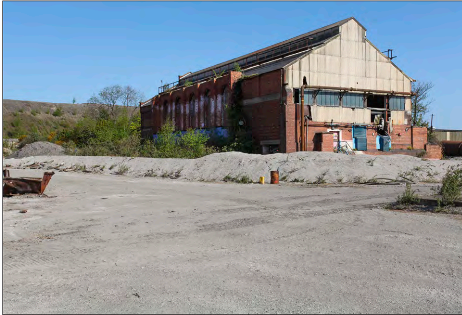
Plate 1: Powerhouse, southeast and southwest elevations
