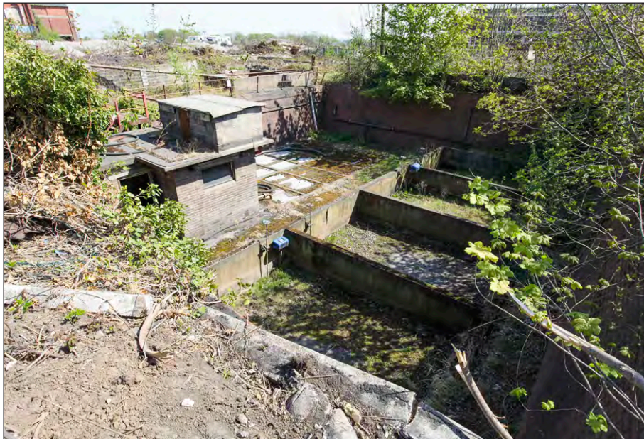
Plate 82: Sewage Plant overview, facing east
