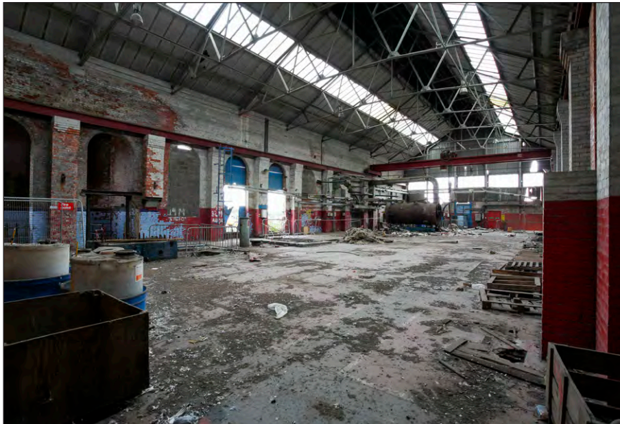
Plate 5: Powerhouse, principal room overview, facing south
