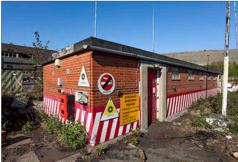
Plate 80: Explosives Store, northeast and southeast elevations
