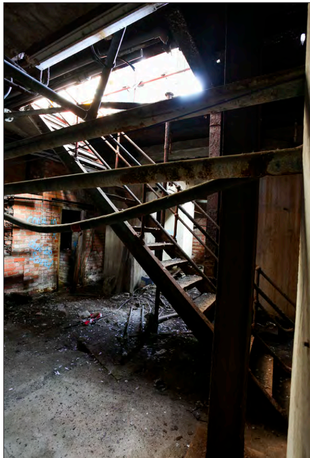
Plate 24: Powerhouse, cellar stairs to principal room, facing east
