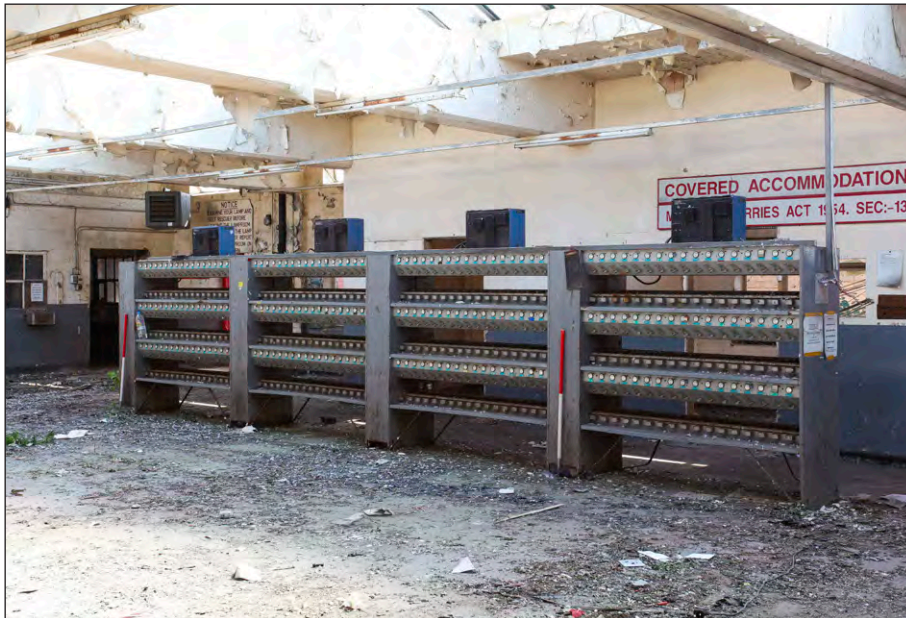
Plate 70: Lamp Room, first floor, lamp stand, facing east
