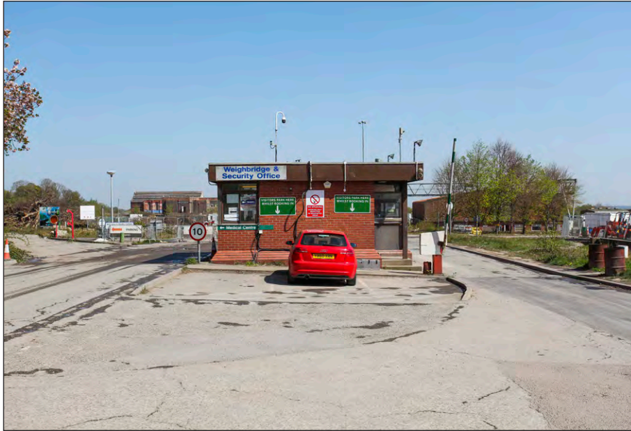
Plate 87: Gatehouse, southwest elevation
