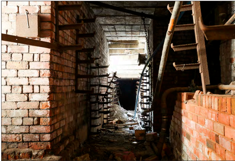
Plate 29: Powerhouse, pipework and tunnel leading southwest from the powerhouse cellar
