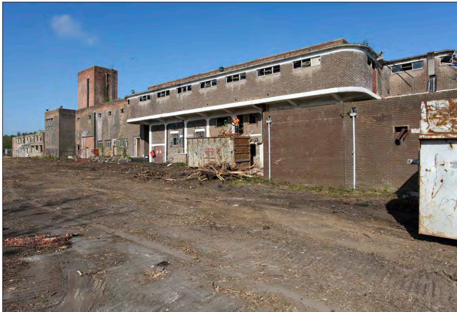
Plate 58: Lamp Room, northeast and southeast elevations
