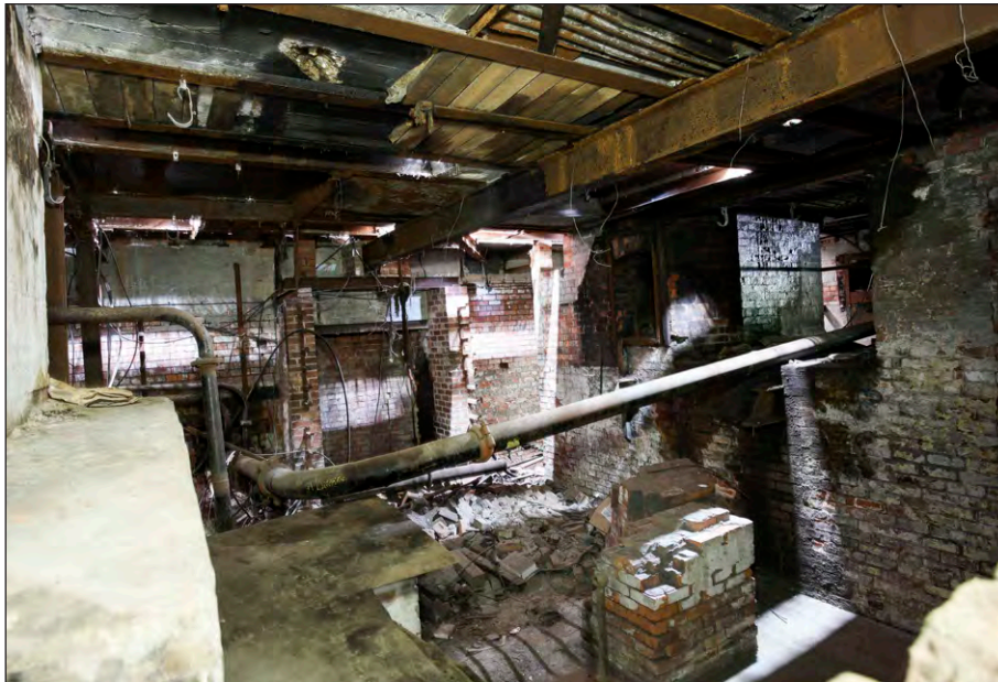
Plate 25: Powerhouse, example of cellar room, facing west
