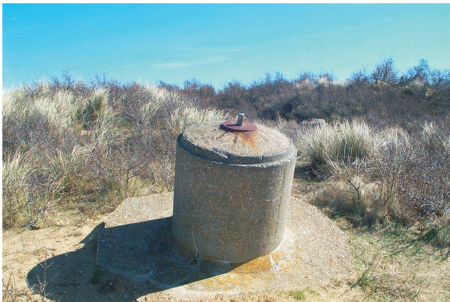
Plate 4. Two WWII spigot mortar bases on the sand dunes at Holme-next-the-Sea, illustrating how even recent sites can become intertidal through coastal erosion
