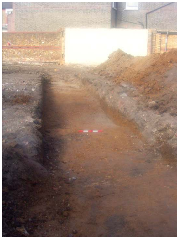
Plate 2: Trench from south
