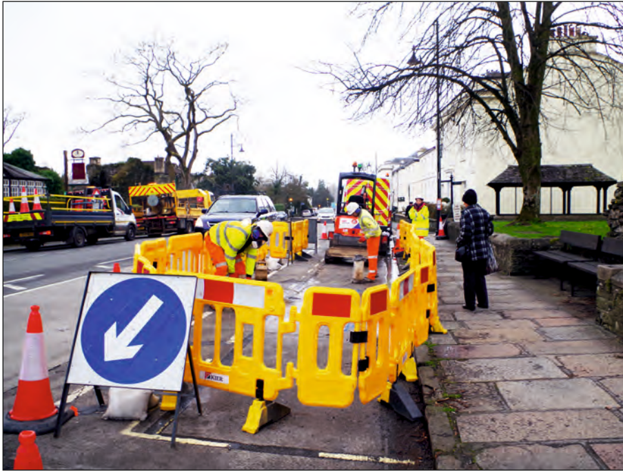
Plate 1: Location working shot of excavation
