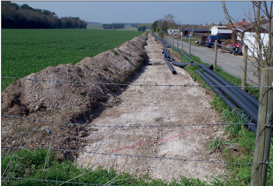
Plate 2: Cable easement viewed from the west showing undisturbed chalk geology
