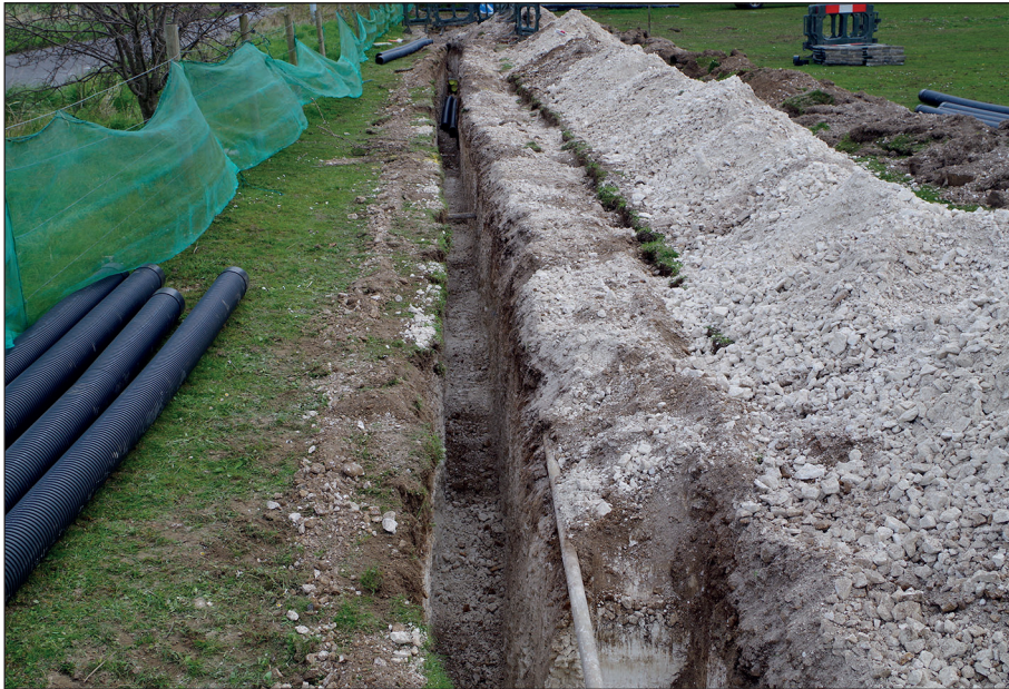
Plate 1: Cable easement and trench viewed from the east
