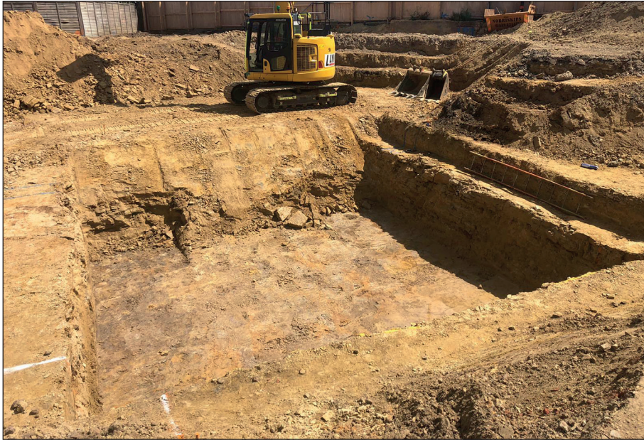
Plate 1: Excavated area, viewed from the southwest
