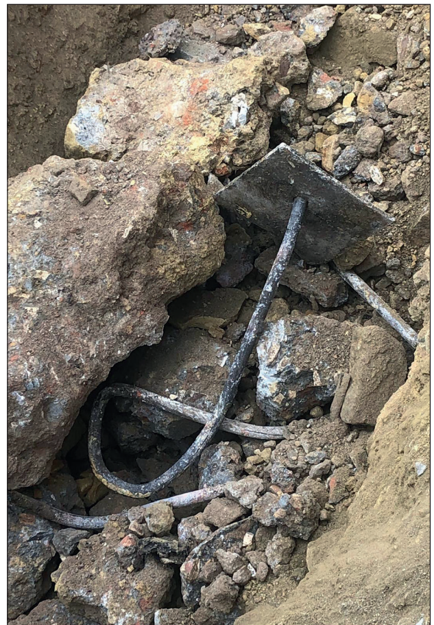
Plate 6: Metal supports within concrete post
