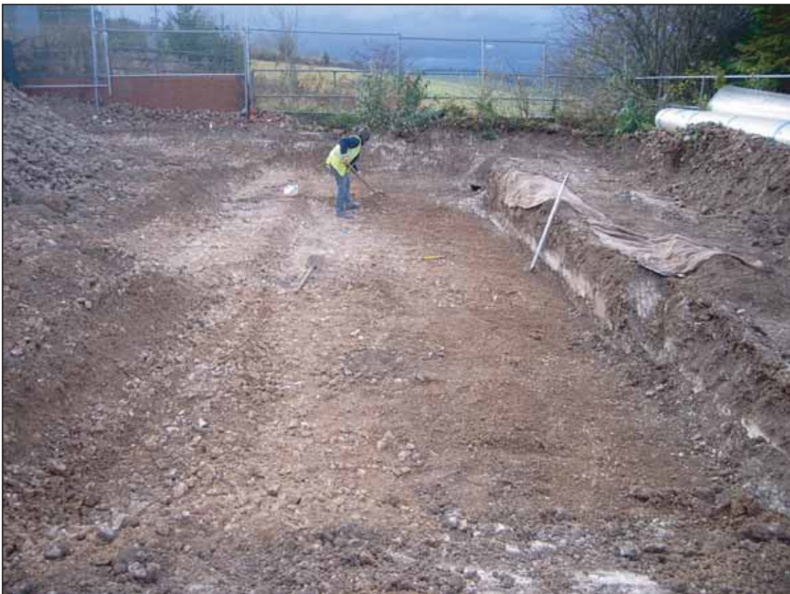
Plate 2: Area 2 viewed from the north-north-east
