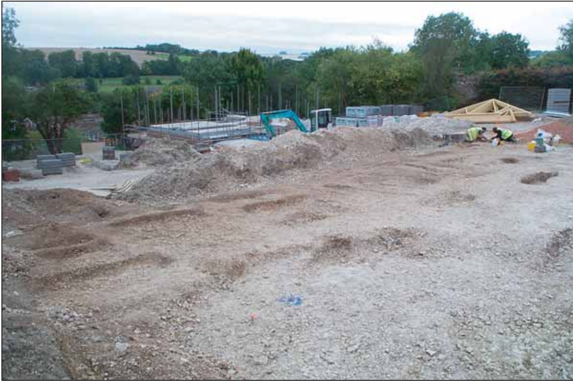
Plate 1: Area 1 viewed from the south-east
