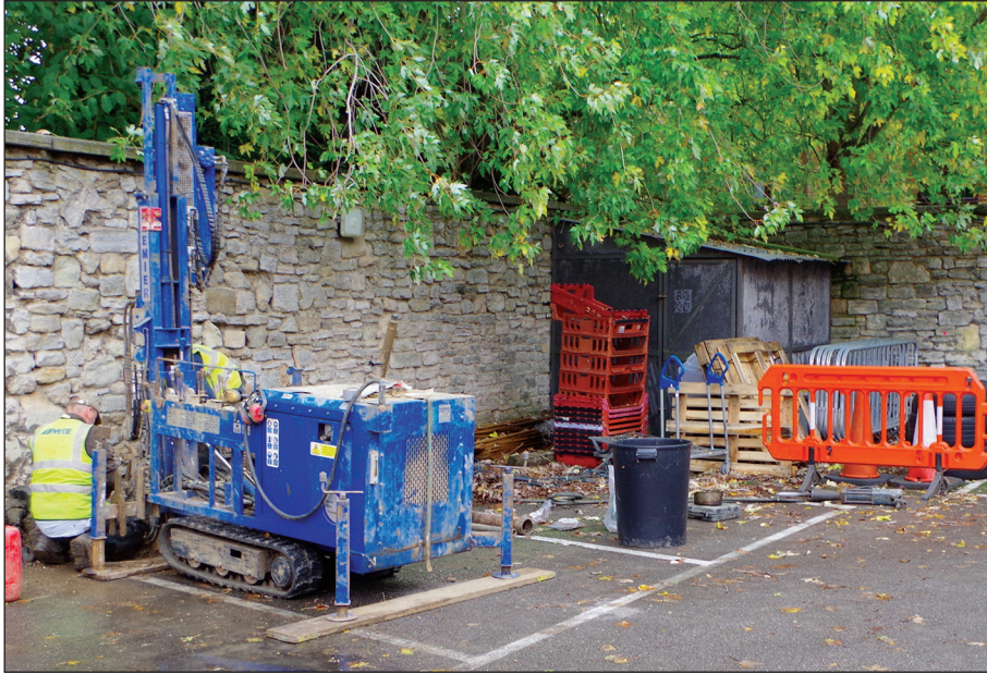
Plate 5: Borehole working shot, view from the north-west.
