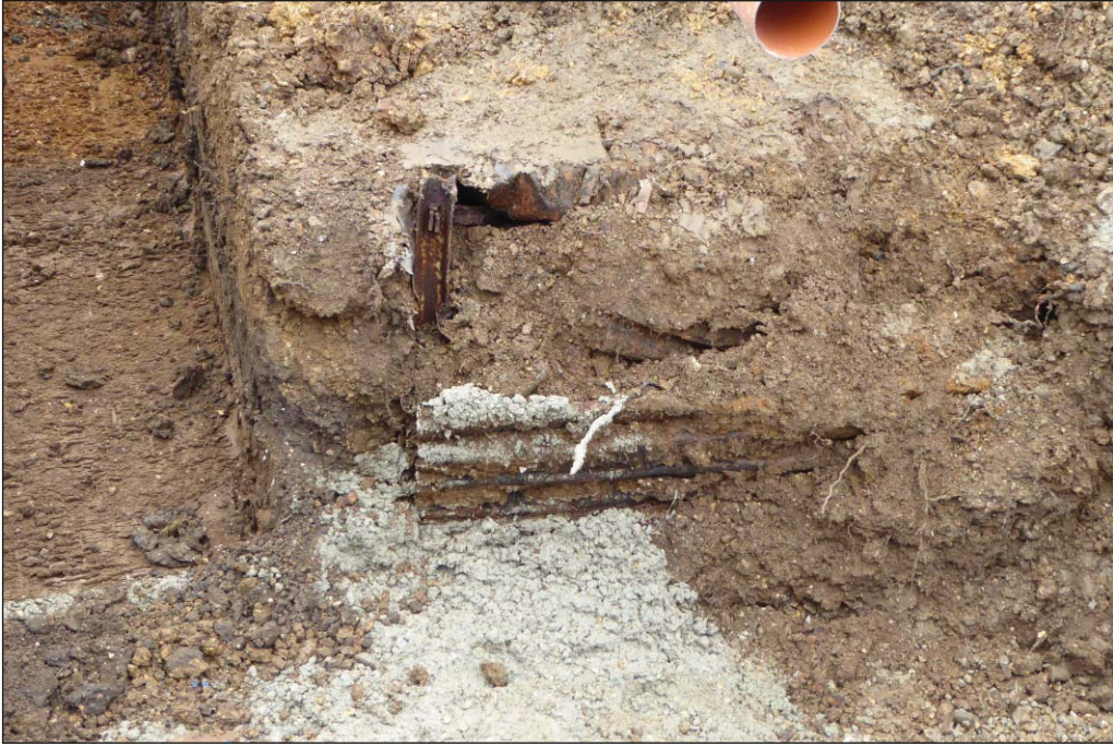
Plate 3: Detail of south-east facing elevation of corrugated iron Anderson shelter lining 1205 (no scale)
