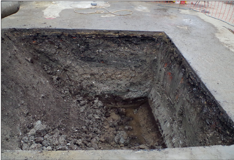
Plate 3: South-east corner of Trench 2, view from the south-east.
