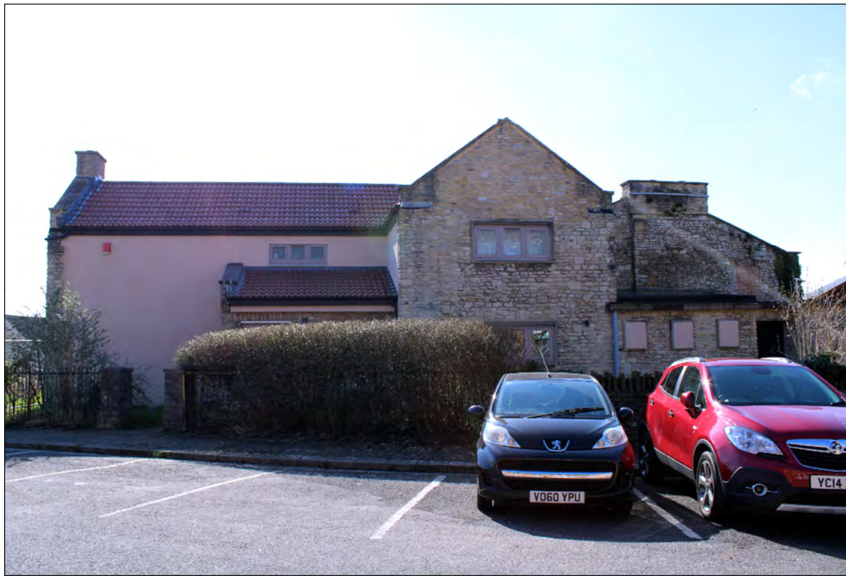
Plate 5) The Cairn, view from the north
