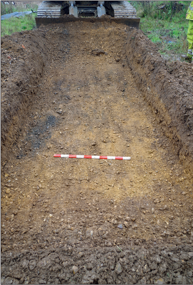
Plate 1: View of pipeline section from the southeast
