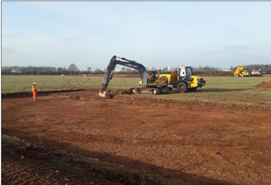
Plate 15: Machine stripping Middle Bronze Age enclosure in Area 4, view from south-east
