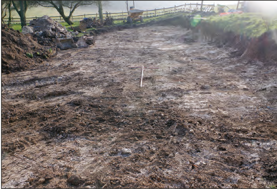
Plate 1: Excavation area, view from north. 2.0 m and 1.0 m scales
