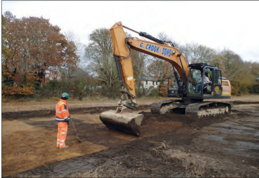
Figure 6: Excavation of Area 1
