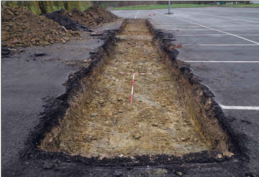
Plate 9: Trench 5 (view from the south)
