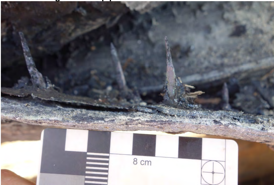
Lead sheathing profile and a thin layer of copper sheathing in between the lead and the timber.
