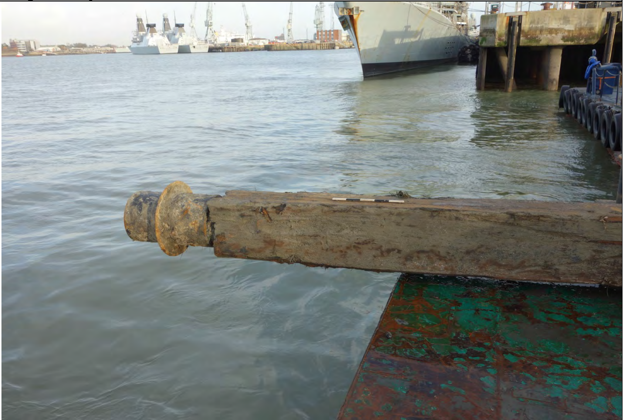
Head of pile with cylindrical flanged steel fitting
