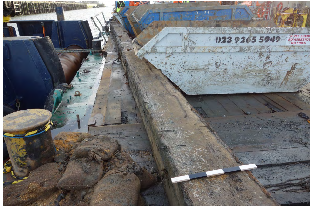
Looking along pile towards heel
