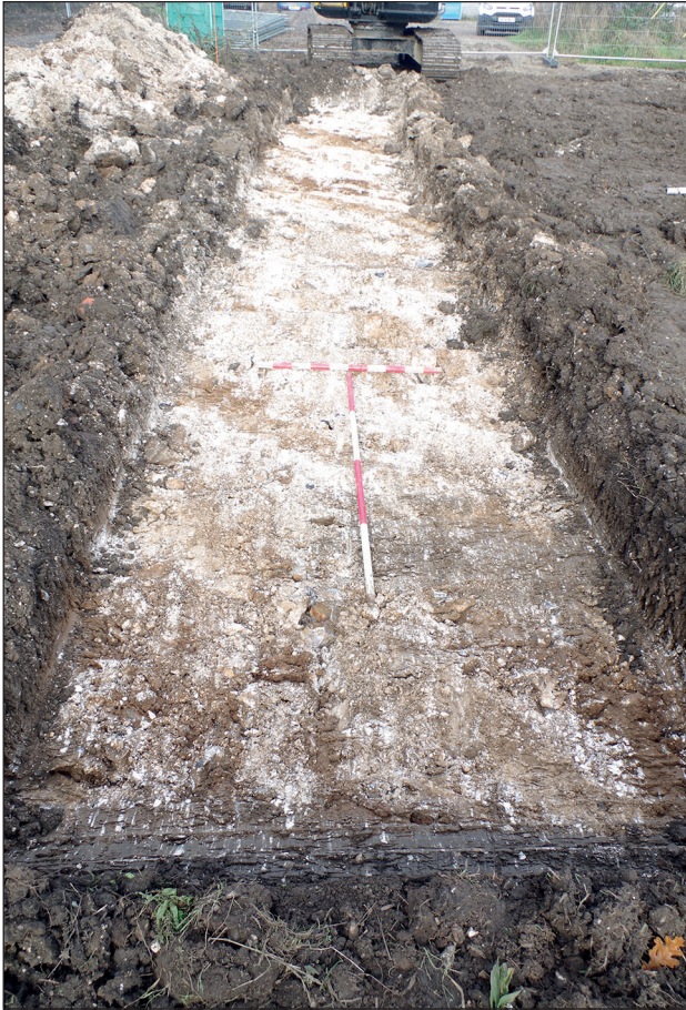
Plate 1: Trench 1 from the south
