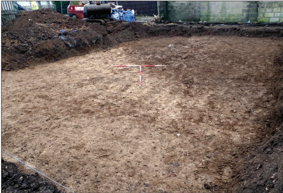
Plate 1: Main SMS area, viewed from the north-west
