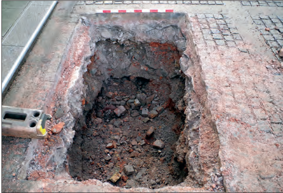
Plate 7: TP7, looking south. 1 m scale.
