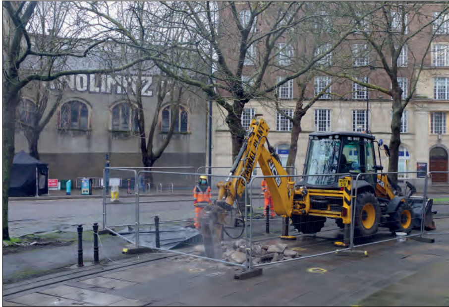
Plate 3: Excavation of TP15, looking north towards Wine Street.
