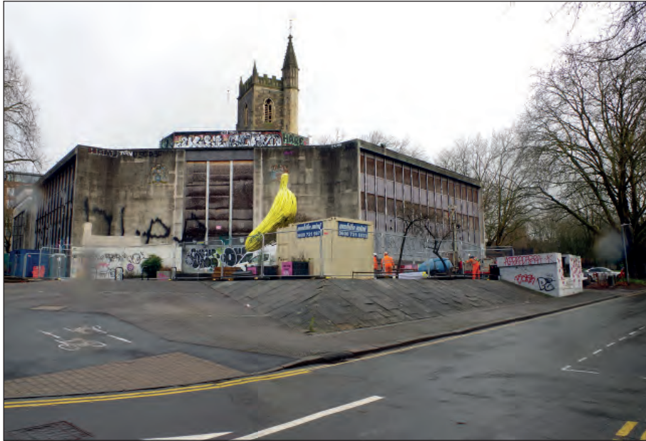
Plate 1: General view of Norwich Union House from the south-west
