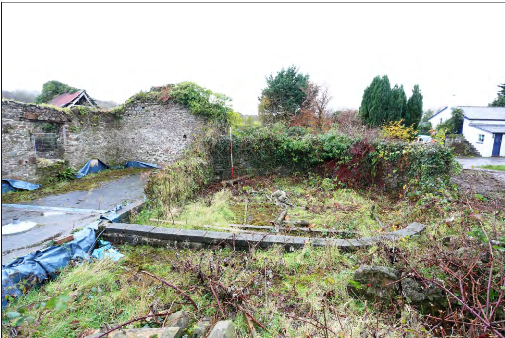
Plate 60: Former farm range building 8 viewed from east showing remains of horse-gin house
