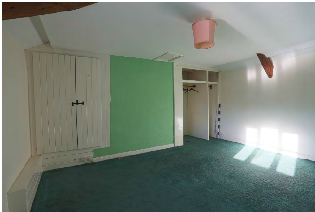
Plate 34: Steart Farmhouse first floor room F4 showing west central chimney
