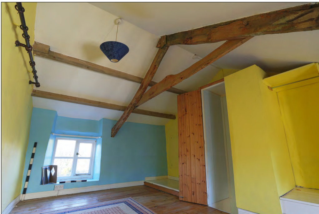
Plate 38: Steart Farmhouse south-west wing first floor room F5 showing roof truss
