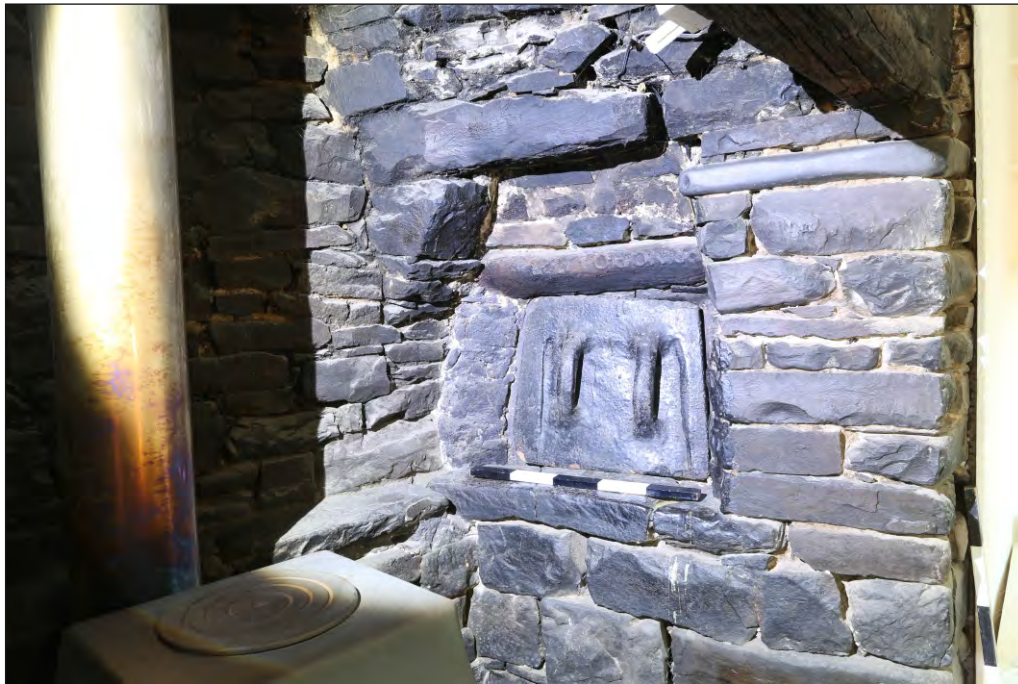
Plate 17: Steart Farmhouse room G4 north cloam oven with cast iron door in-situ
