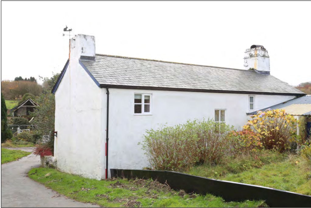
Plate 3: Steart Farmhouse north elevation
