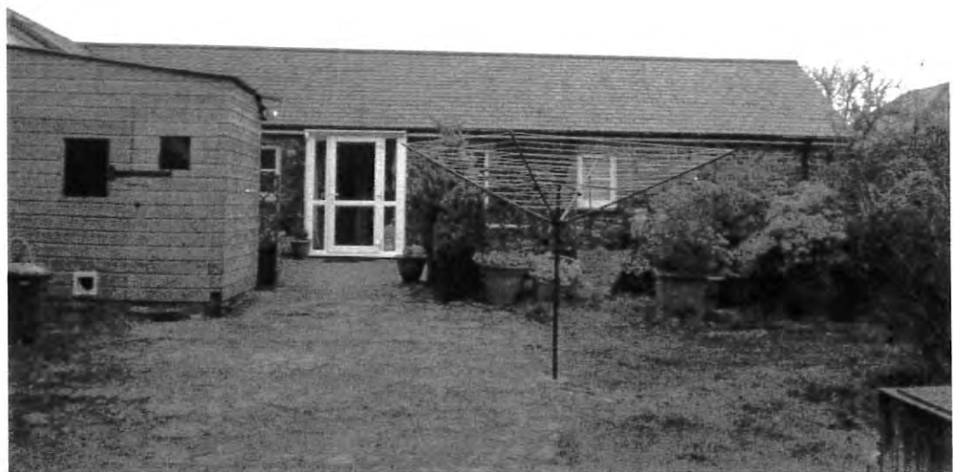
Figure 45a. East elevation of building 04 The Old Shippen retaining original openings and all brickwork dressings. West
