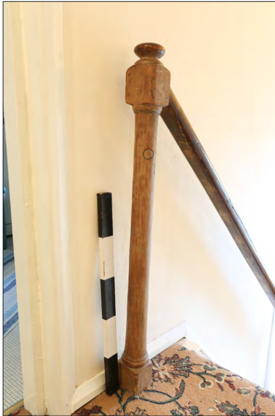
Plate 31: Steart Farmhouse stair post and hand rail
