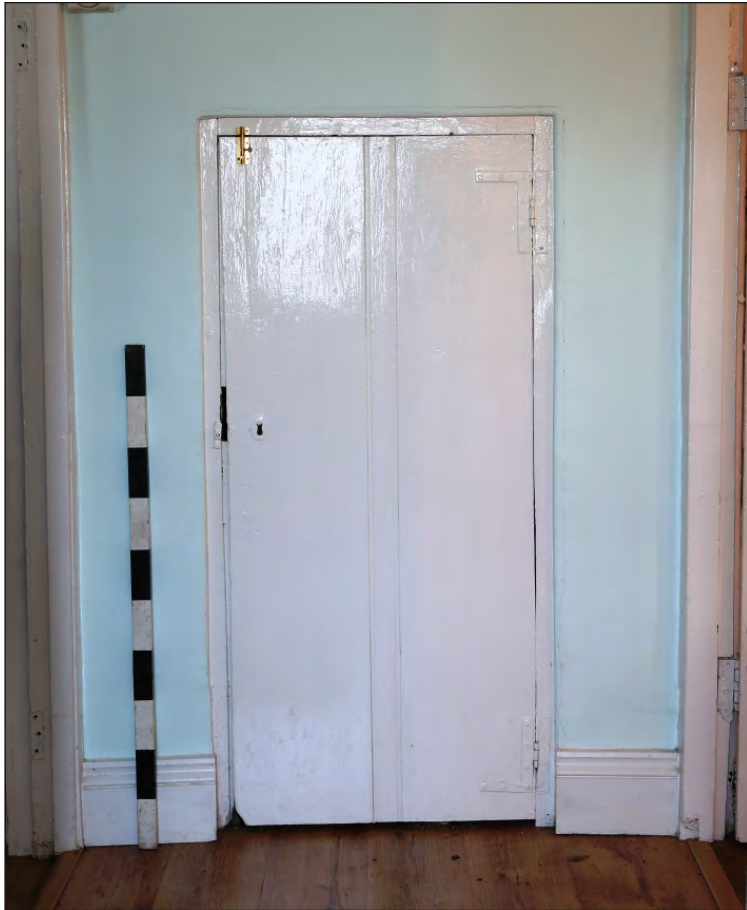
Plate 9: Steart Farmhouse 18th century plank and batten door fitted with 'L' hinges
