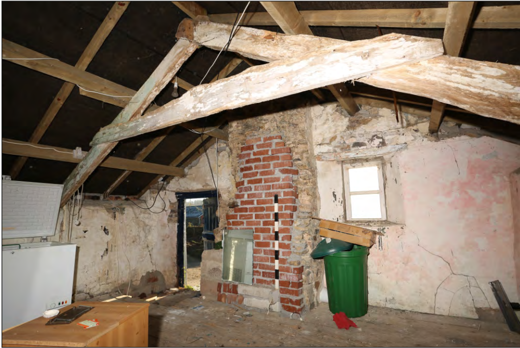
Plate 39: Steart Farmhouse south-west wing first floor room F6 showing roof truss, chimney and window
