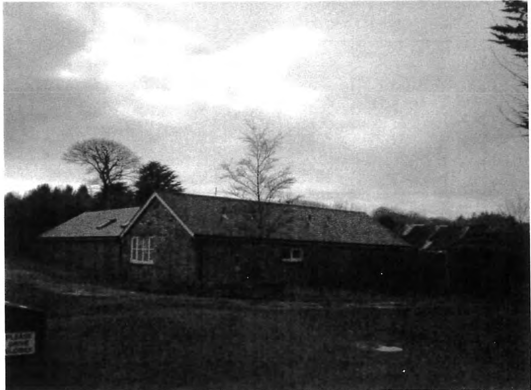
Figure 43a. The Old Shippen east elevation, see also figure 48 and 48a below, and 08 north elevation retaining the window shown in figure 47.
