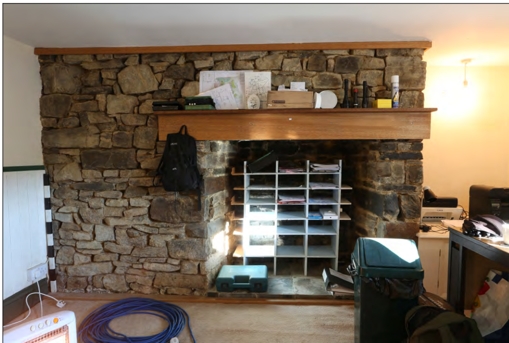
Plate 12: Steart Farmhouse room G3 stone chimney
