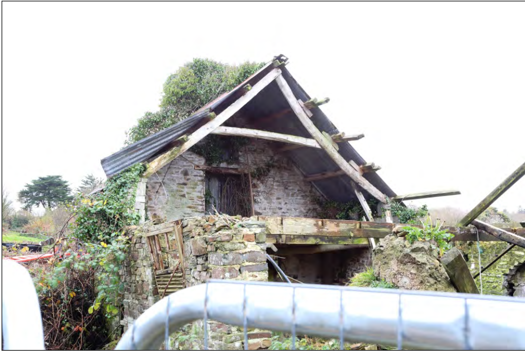
Plate 65: Former barn building 2 surviving roof truss at south end
