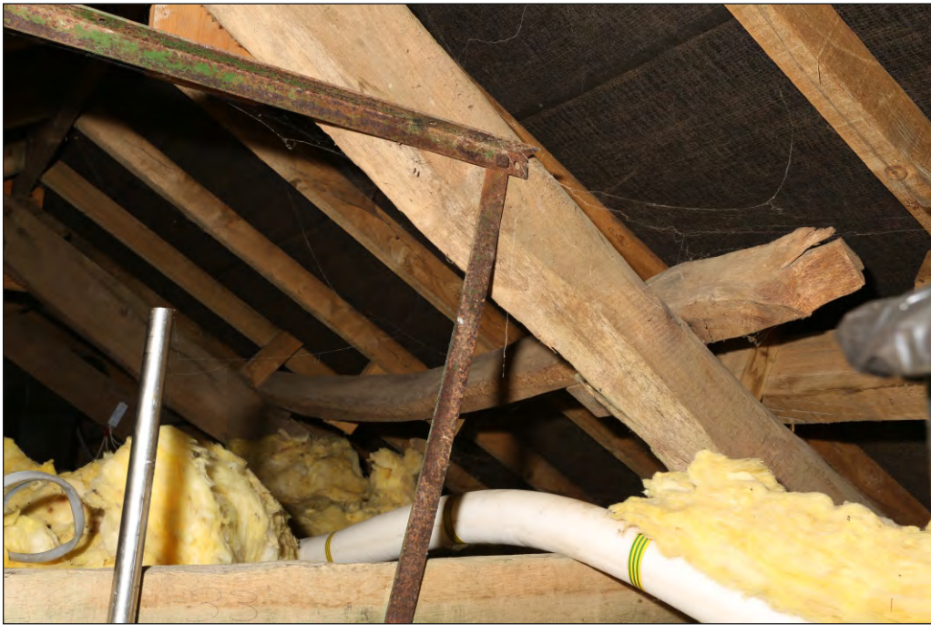
Plate 37: Steart Farmhouse example of thatch purlin between trusses
