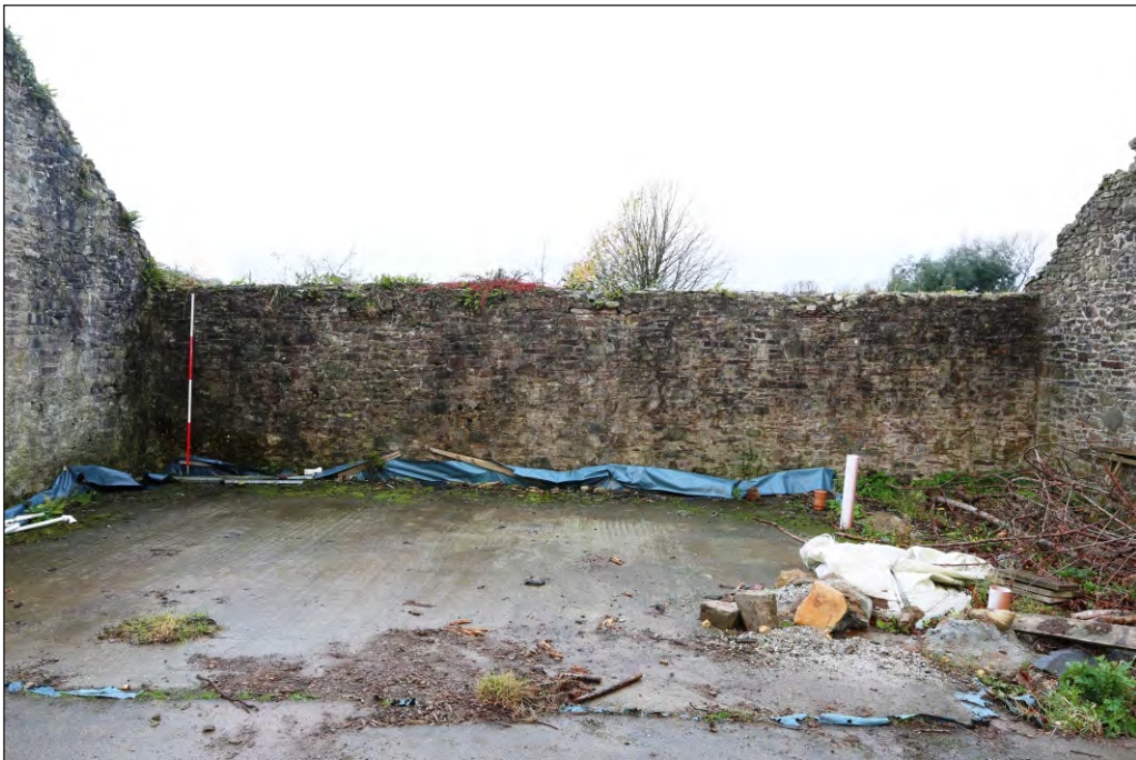
Plate 42: Open fronted cart shed Building 3, interior view of west wall showing timber roof truss pads set in wall fabric
