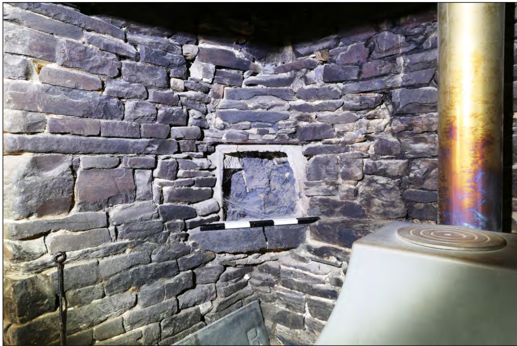
Plate 16: Steart Farmhouse room G4 remains of south cloam oven
