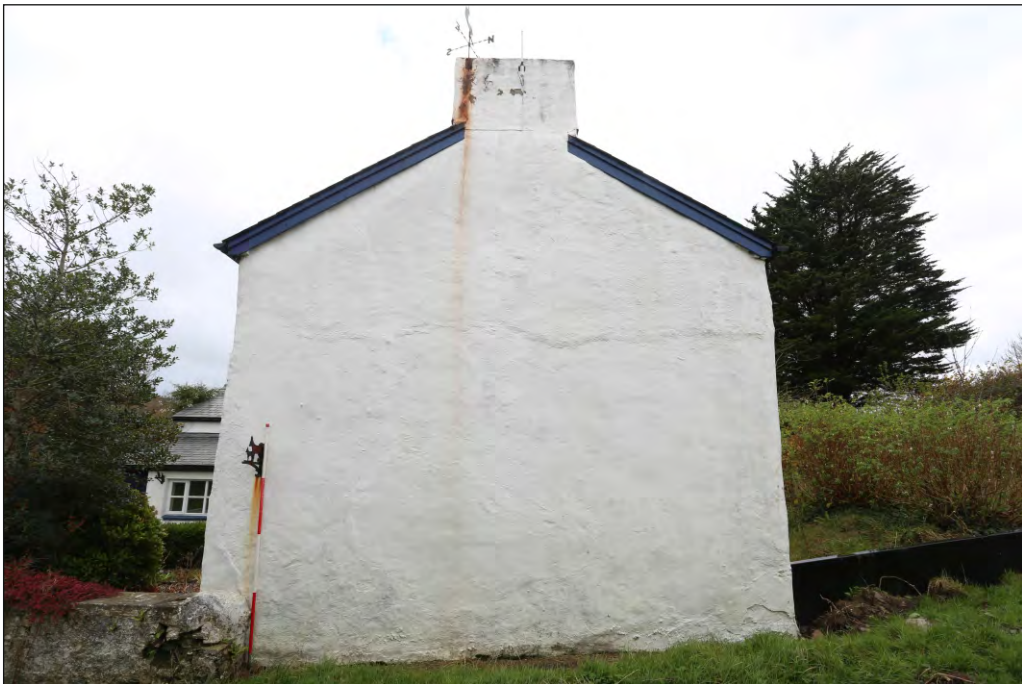
Plate 2: Steart Farmhouse east elevation
