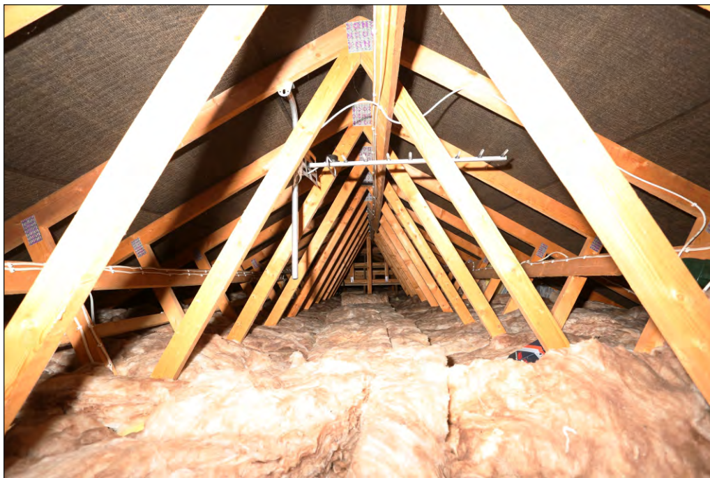
Plate 56: Former farm range building 4, modern roof trusses
