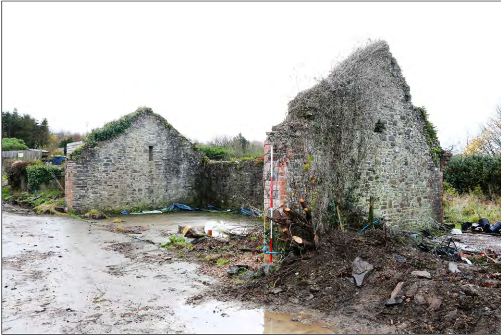
Plate 41: Open fronted cart shed Building 3, viewed from north-east
