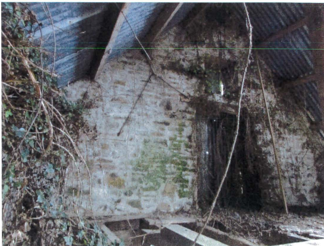
Figure 10: The first floor loading door viewed from the north.
