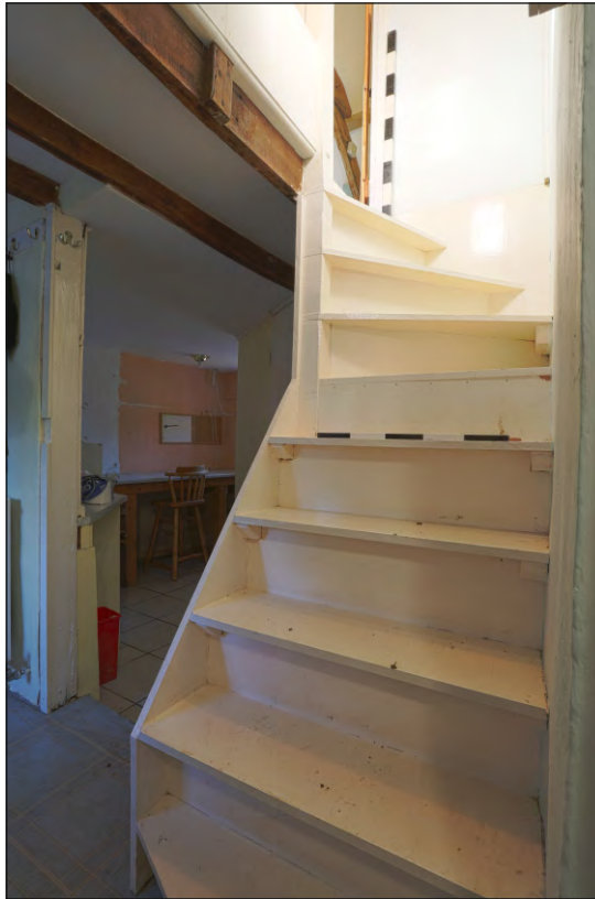
Plate 29: Steart Farmhouse south-west modern stairs to first floor room
