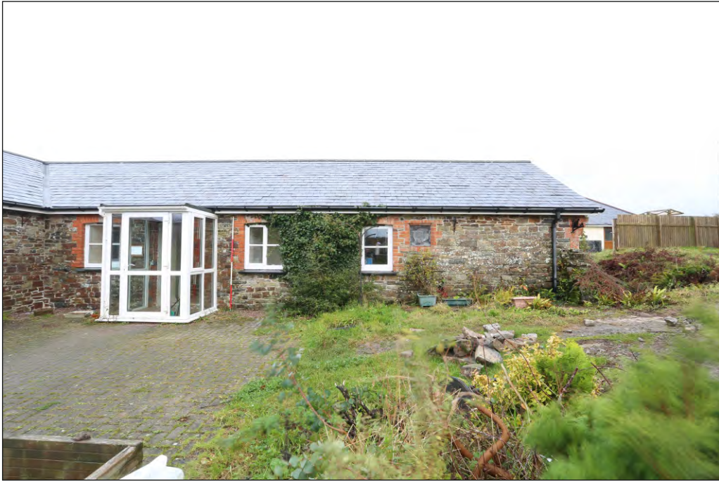
Plate 47: Former farm range building 4, west elevation of south range
