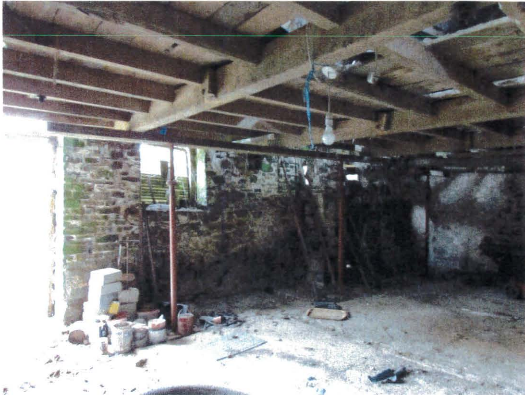
Figure 4: The ground floor viewed from the north-east.
