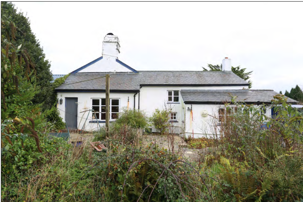
Plate 4: Steart Farmhouse west elevation
