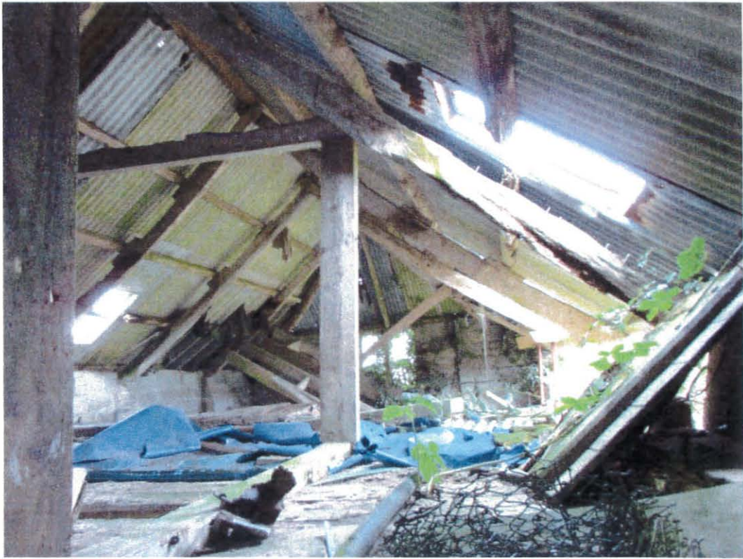
Figure 3: The first floor and roof structure viewed from the south.
