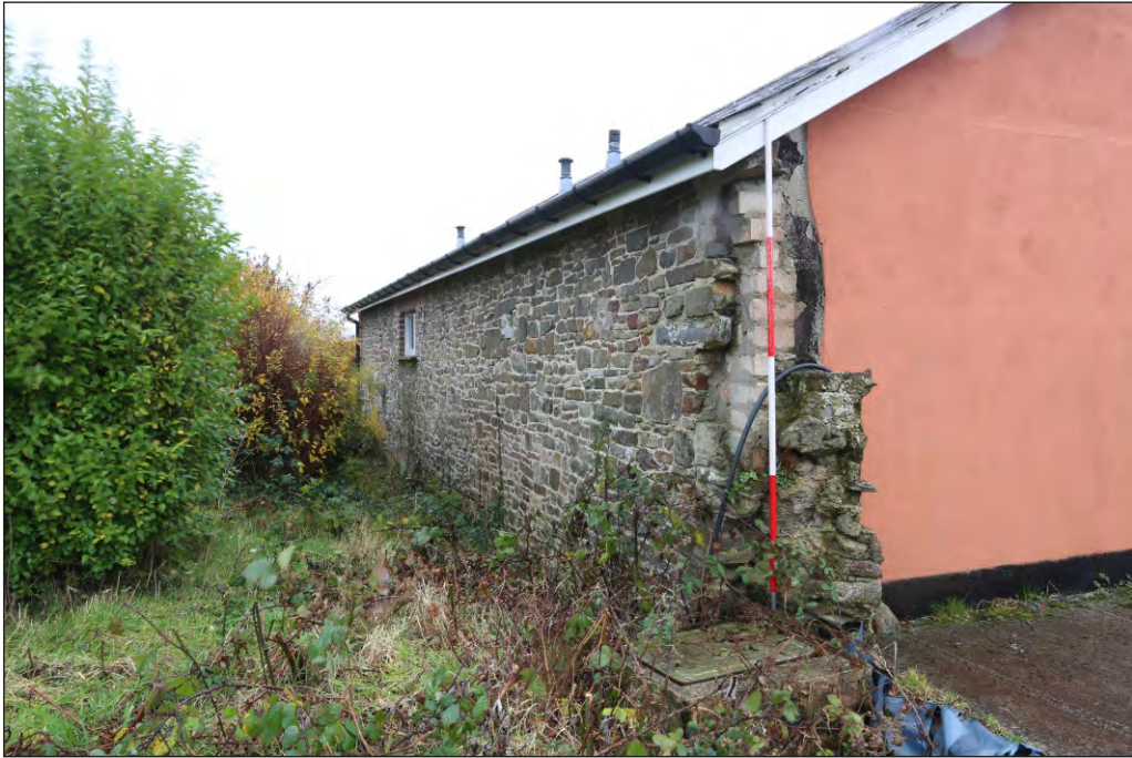
Plate 53: Former farm range building 4 oblique view of north elevation
