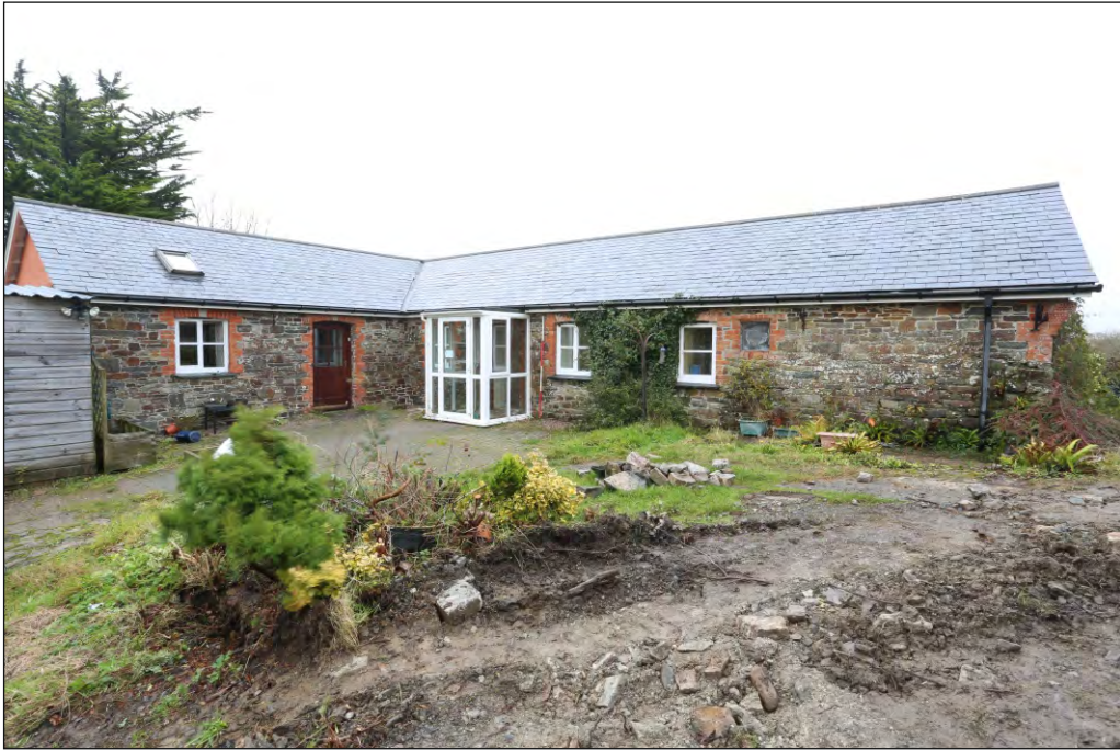
Plate 45: Former farm range building 4, east-west and north-south ranges viewed from south-west
