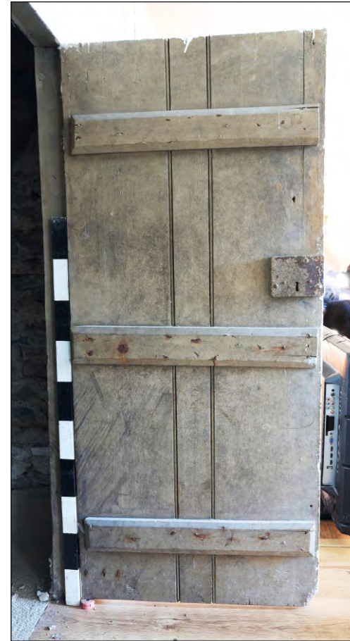
Plate 10: Steart Farmhouse 18th century plank and batten door with metal lock case
