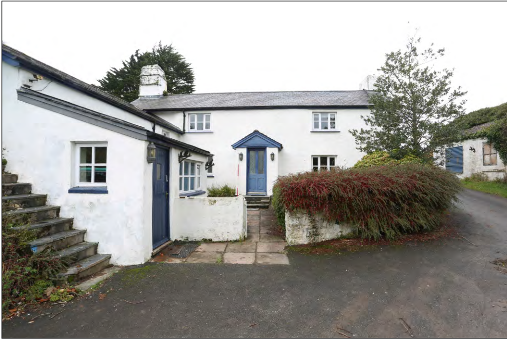
Plate 1: Steart Farmhouse south elevation
