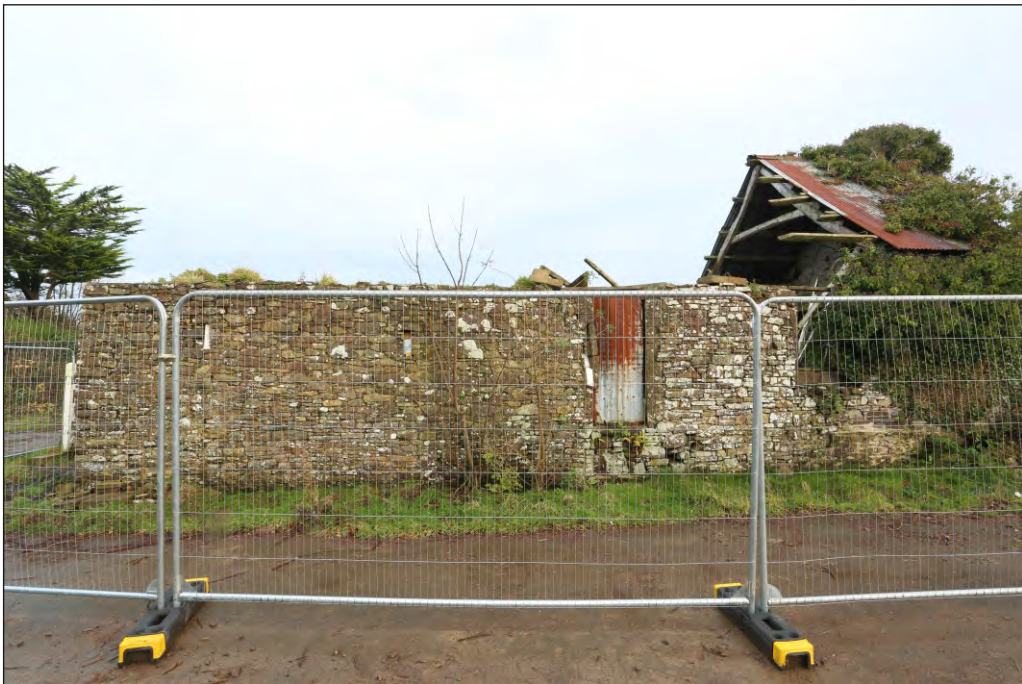
Plate 64: Former barn building 2 west facing stone wall
