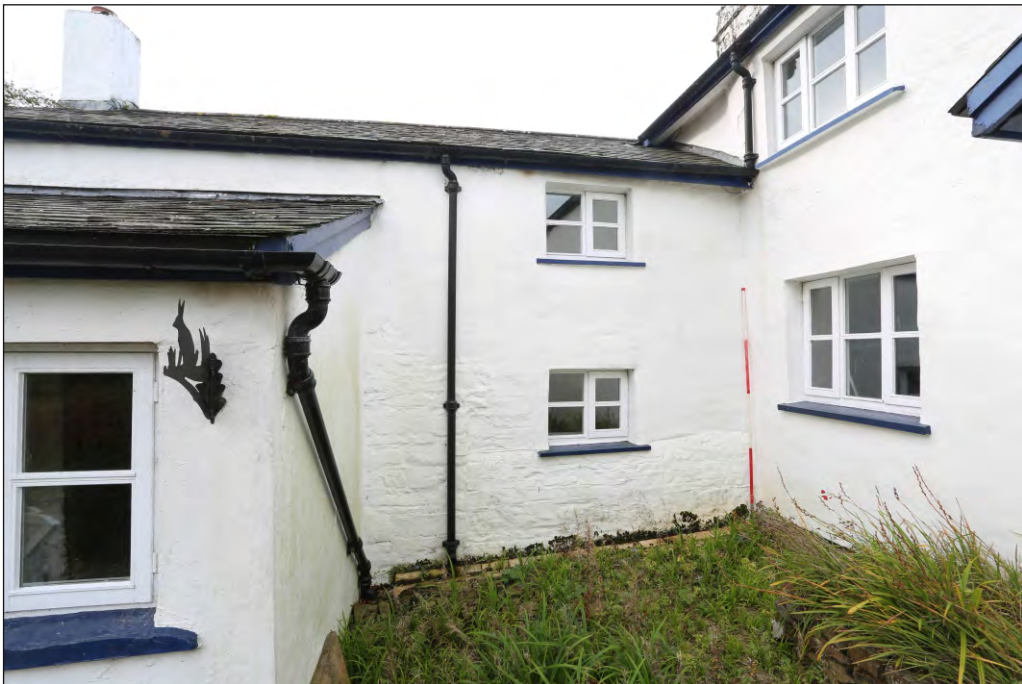
Plate 6: Steart Farmhouse east side of south-west extension showing change in build
