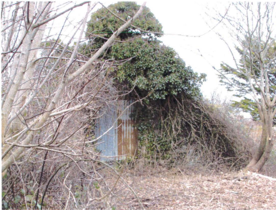
Figure 6: View from the south showing the first floor loading door.
