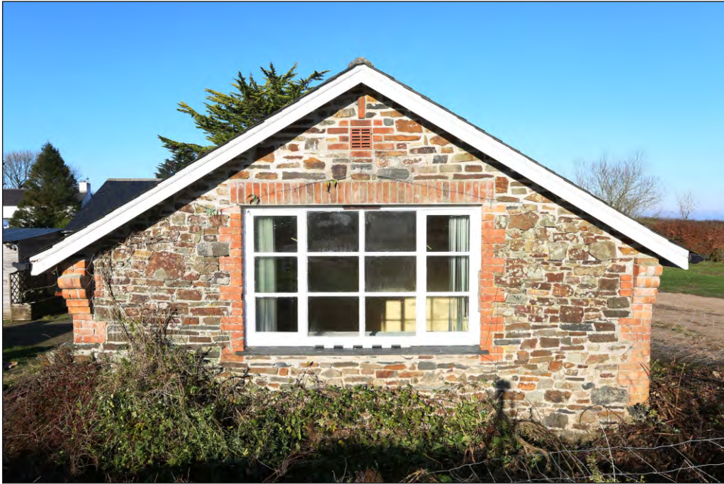
Plate 49: Former farm range building 4 south gable end window
