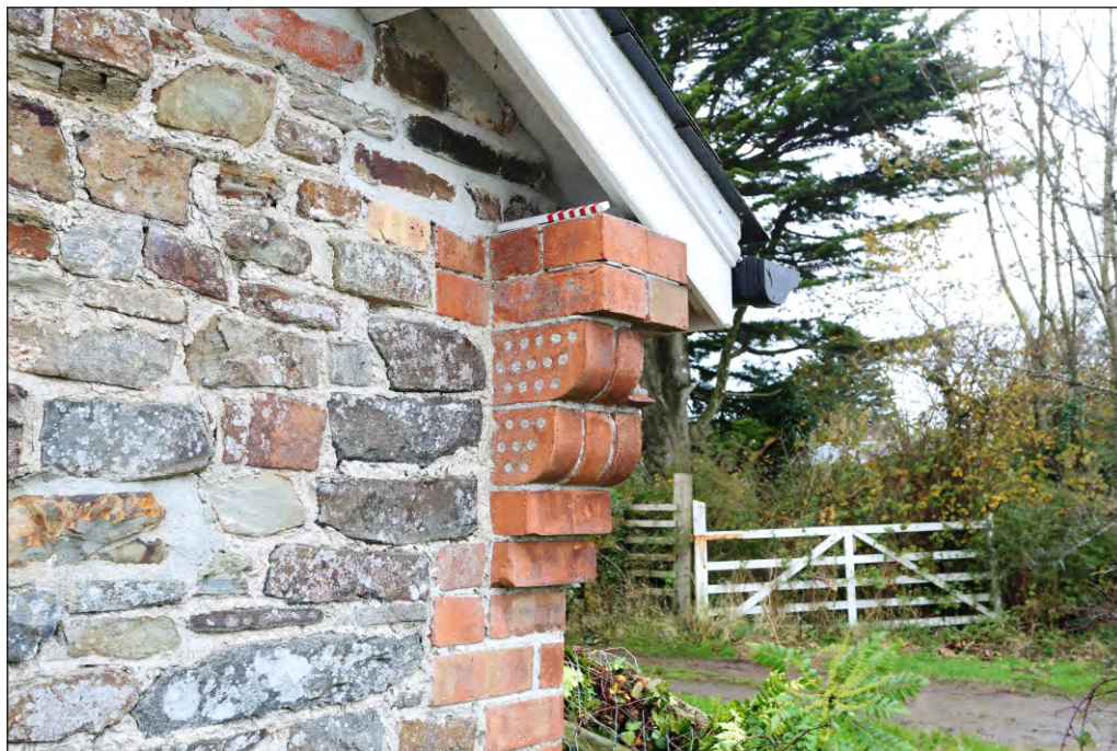
Plate 52: Former farm range building 4 good surviving example of Rolle's brick corbel
