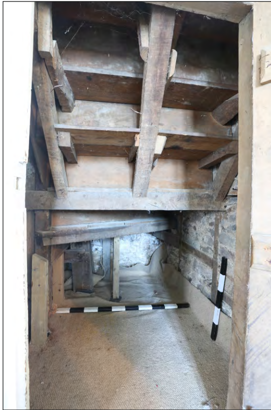
Plate 11: Steart farmhouse 18th century wooden stair framing in under stair cupboard
