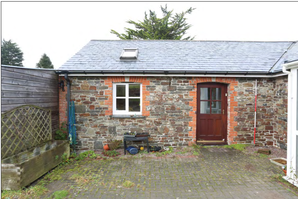
Plate 46: Former farm range building 4, south elevation of east-west range
