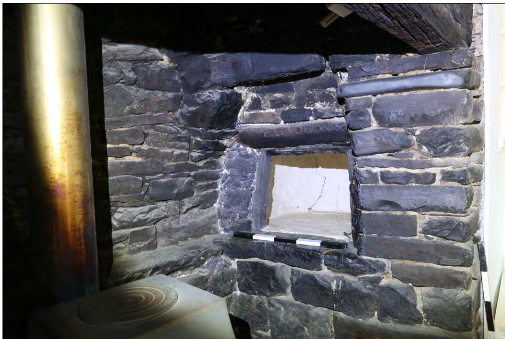
Plate 18: Steart Farmhouse room G4 north cloam oven with cast iron door removed
