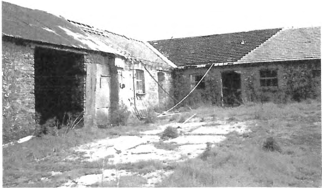
Figure 41. 1995 photograph. Inner angle of Buildings 04 and 08 creating the NE corner of the yard, building 04 shows Rolle brickwork, building 08 does not.
