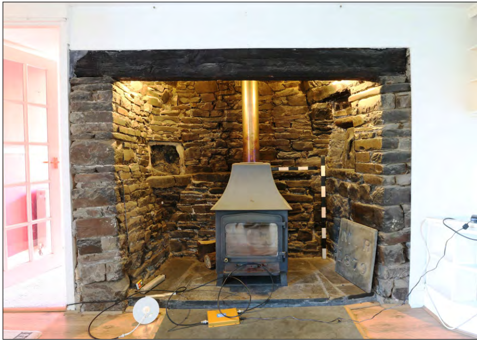
Plate 15: Steart Farmhouse room G4 inglenook fireplace
