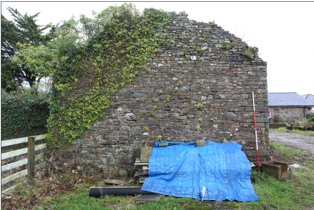
Plate 58: Former farm range building 8, west elevation
