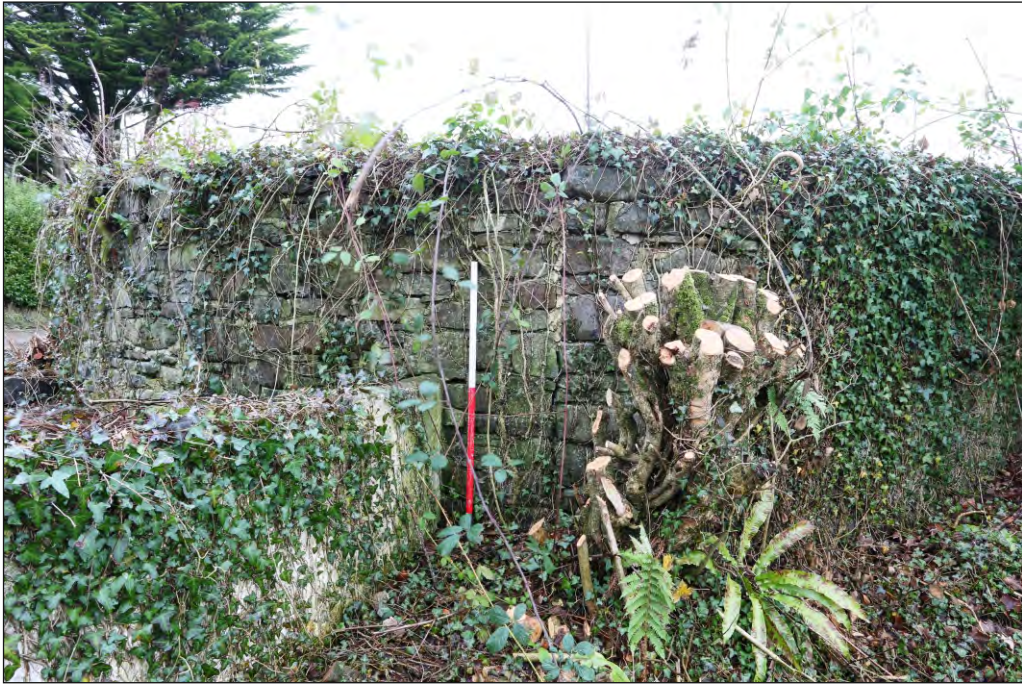
Plate 61: Former farm range building 8 evidence of blocked door entrance to horse-gin house
