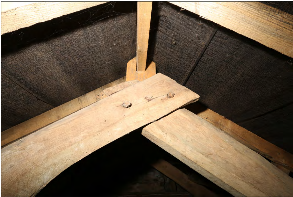
Plate 36: Steart Farmhouse typical roof truss apex joint
