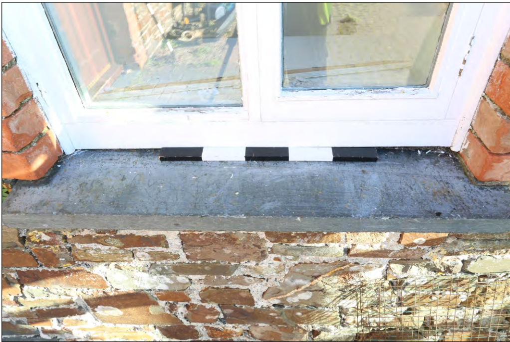
Plate 48: Former farm range building 4, detail of apotropaic marks on window sill
