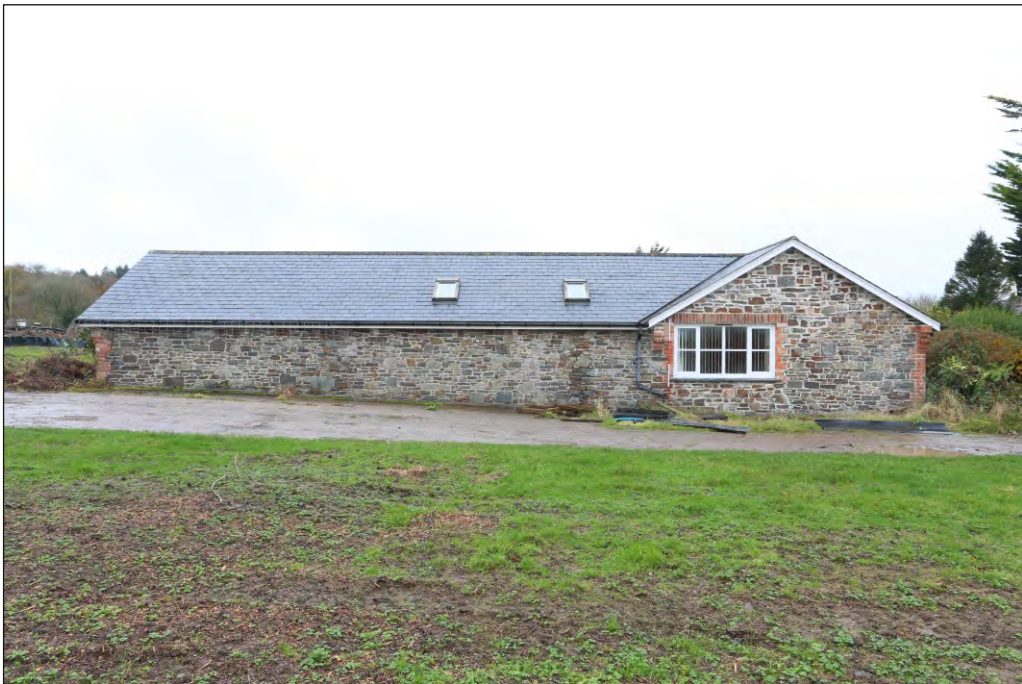
Plate 50: Former farm range building 4 east facing elevation
