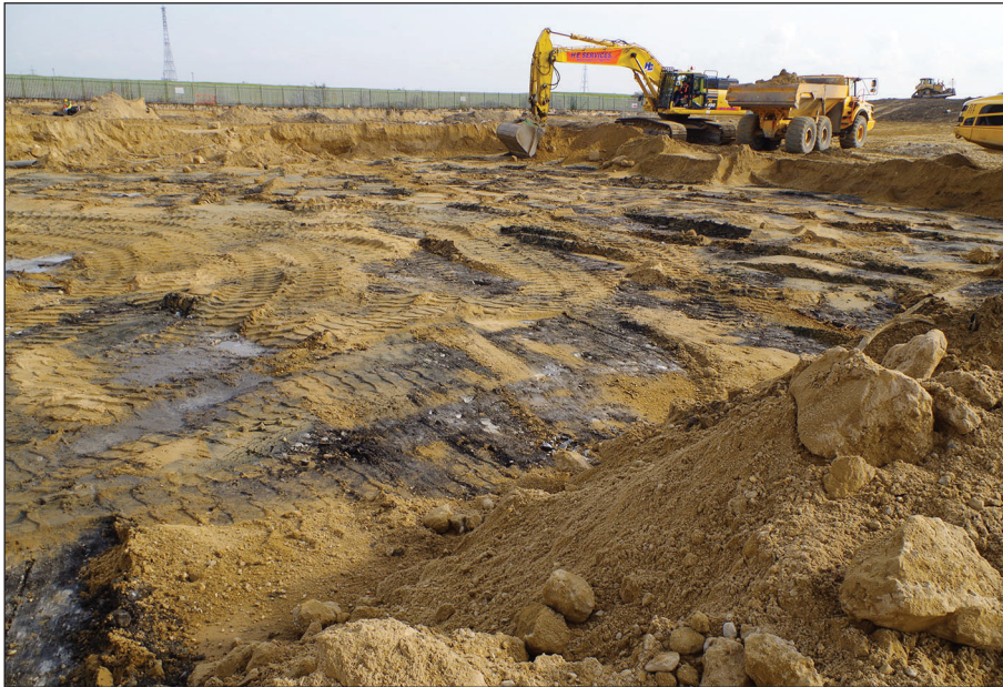
Plate 1: Unit 1 under excavation, viewed from the southwest
