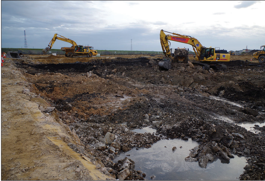
Plate 3: Unit under excavation, viewed from the north
