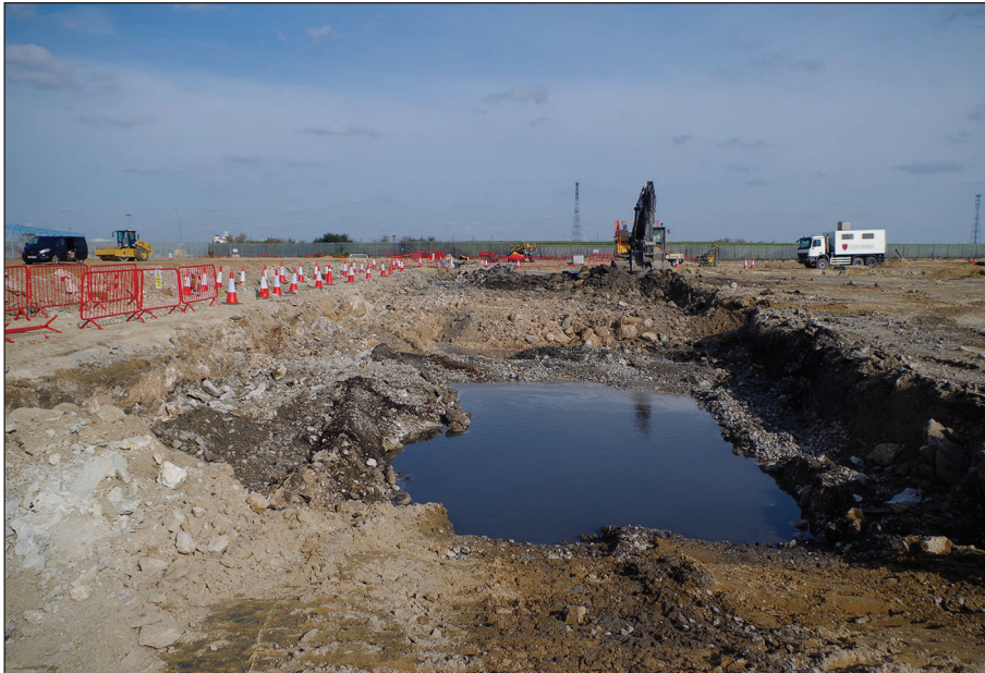
Plate 2: Unit under excavation, viewed from the west
