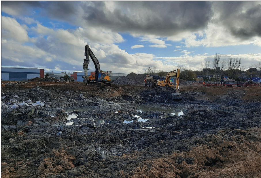
Plate 4: Attenuation area under excavation, viewed from the west
