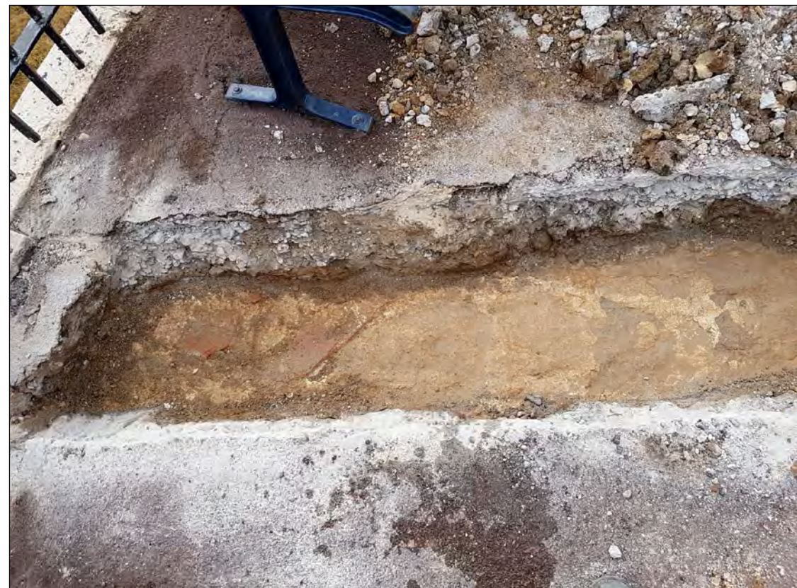
Plate 7) Northeastern end of TPRH105A, mortar surface
