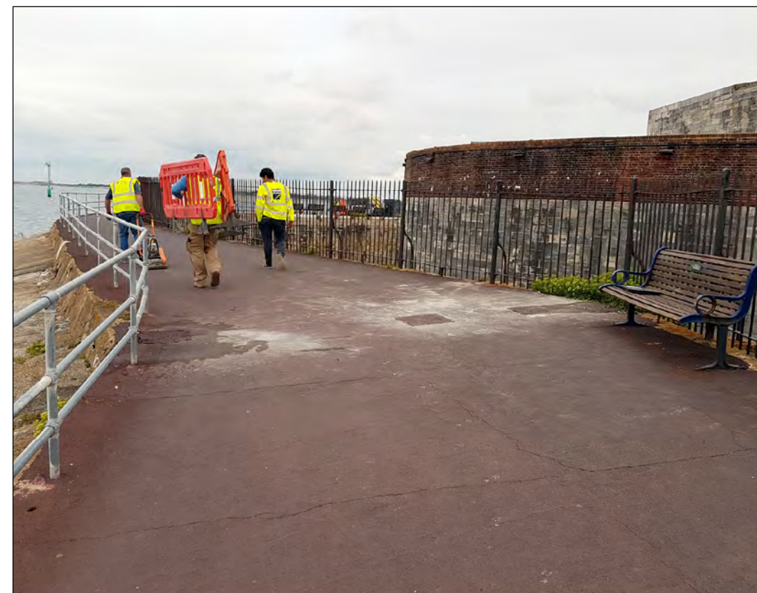
Plate 12) Locations of the separate sections of TP105B after reinstatement
