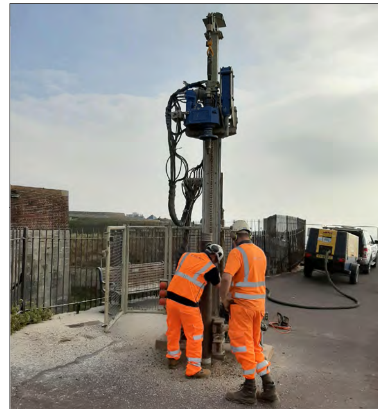
Plate 16) Working shot, excavating RH4, view from the north-east
