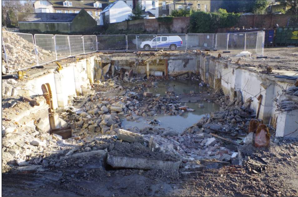
Plate 7: Watching brief area, viewed from the south west
