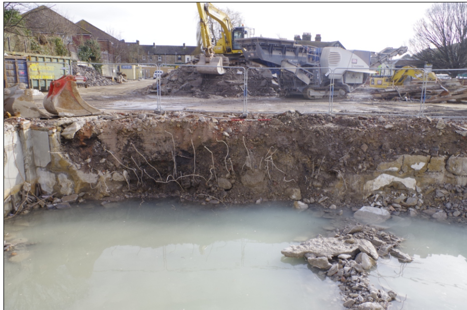
Plate 8: Basement partially demolished, viewed from the north west
