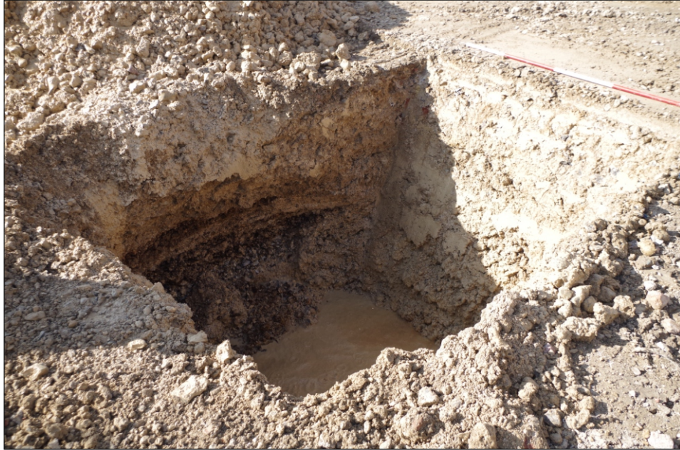
Plate 1: Test Pit 3, viewed from the east
