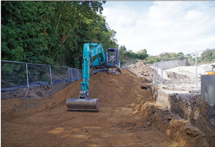
Plate 3: Tank Strip – Start of strip
