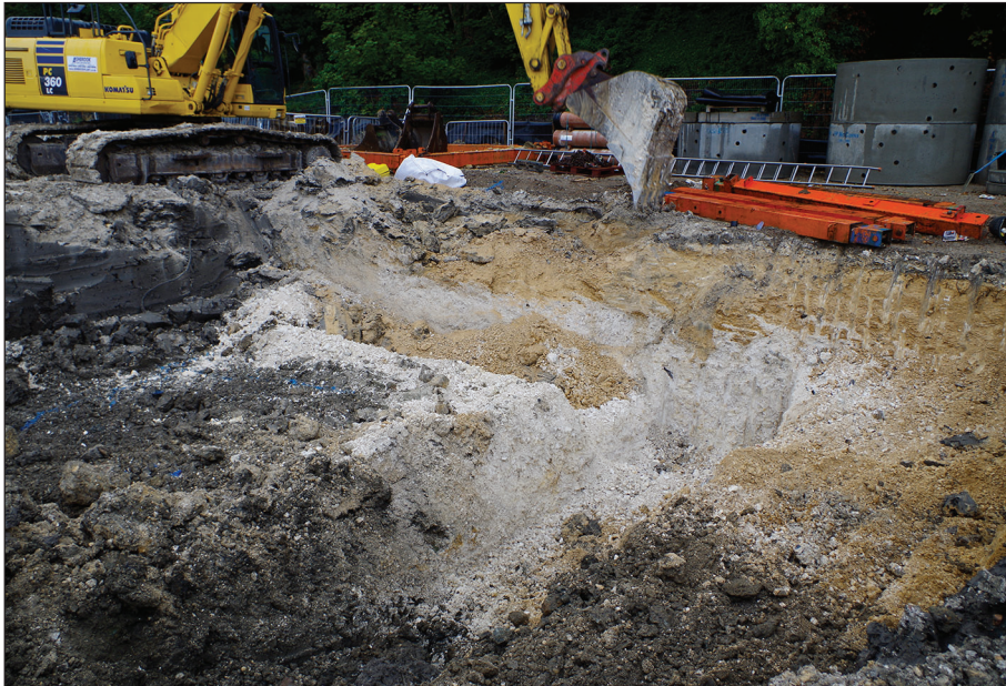
Plate 10: Soakaway 2 – Made Ground
