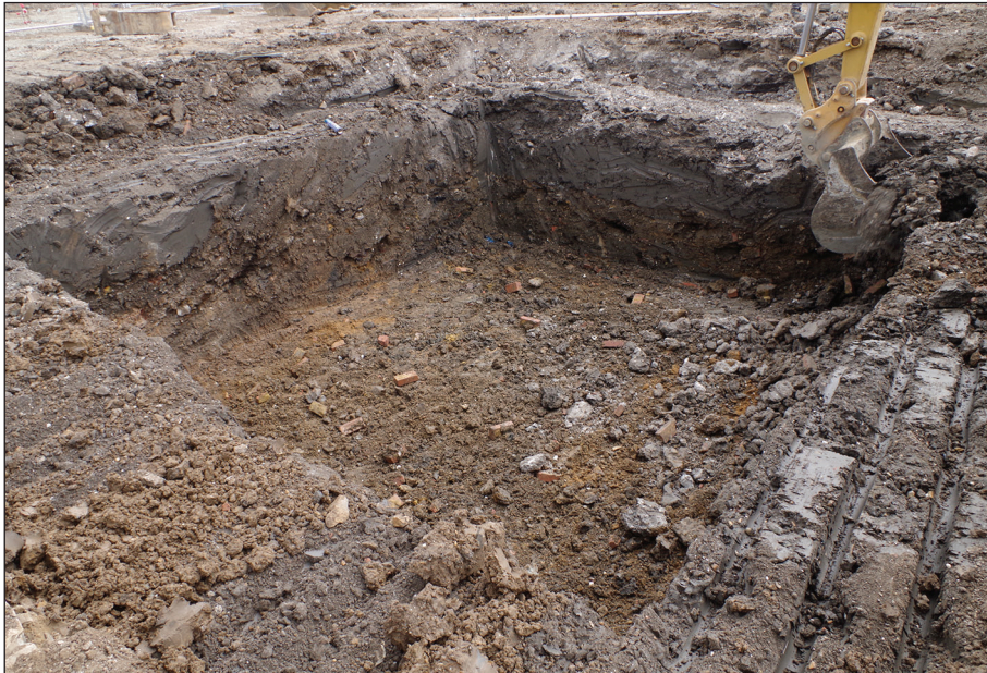
Plate 6: Soakaway 1 – Initial Strip
