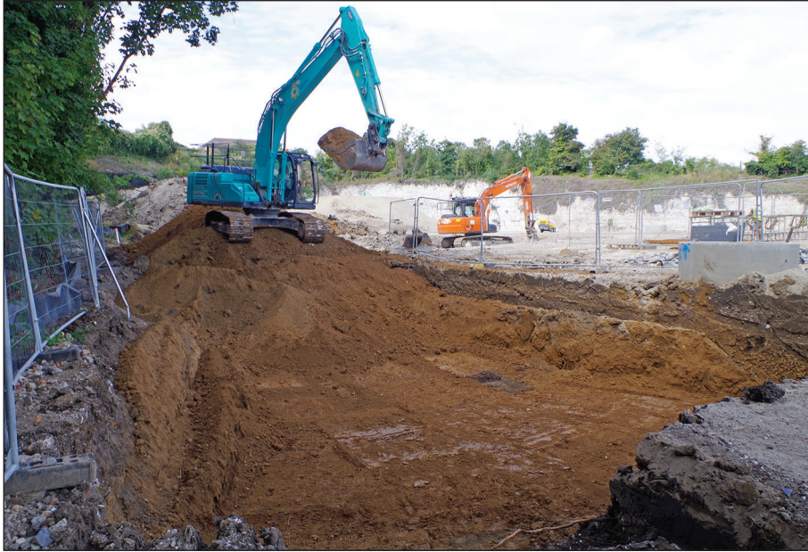
Plate 5: Tank Strip – Near completed strip
