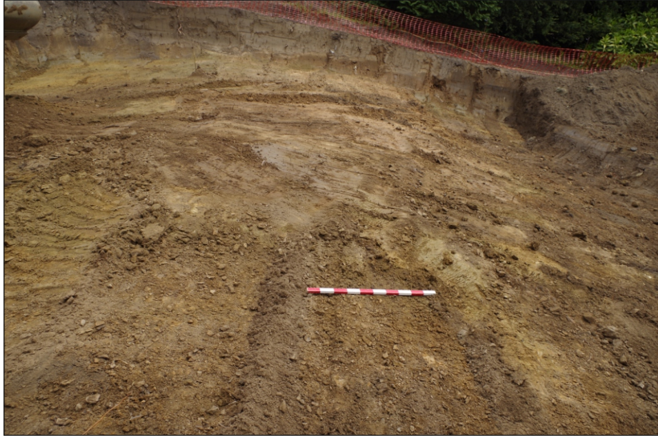
Plate 3: Ground reduction within a garage footprint, viewed from the south west
