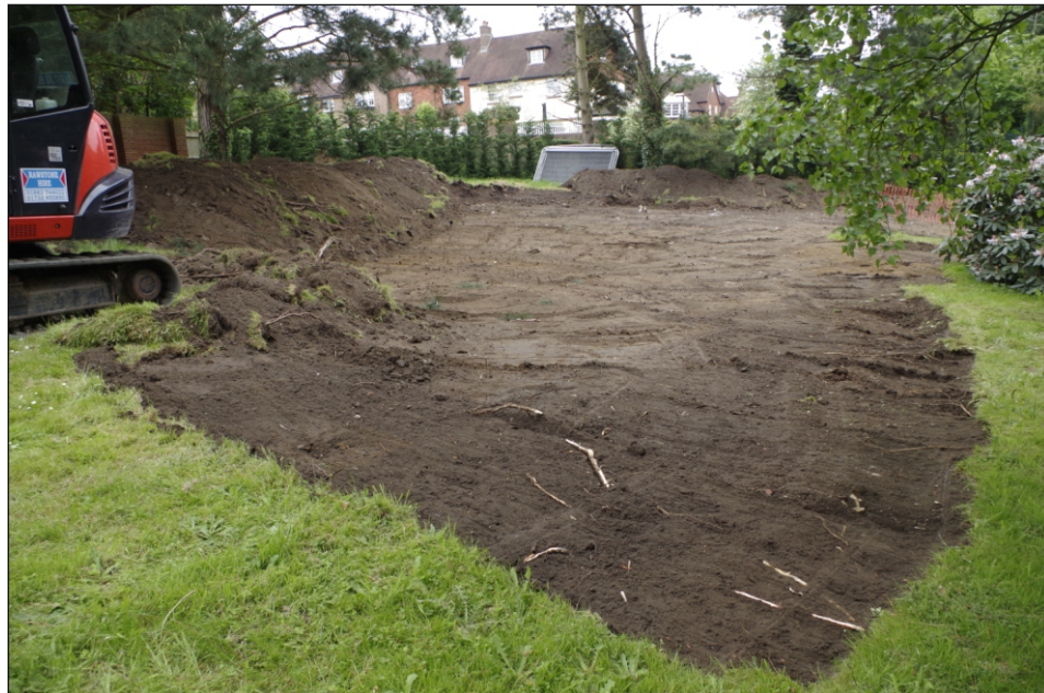
Plate 2: Topsoil reduction for a spoil heap, viewed from the west
