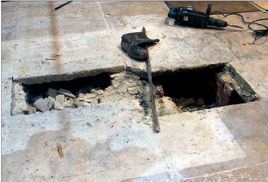
Plate 14: Lifting of flooring slabs within the church
