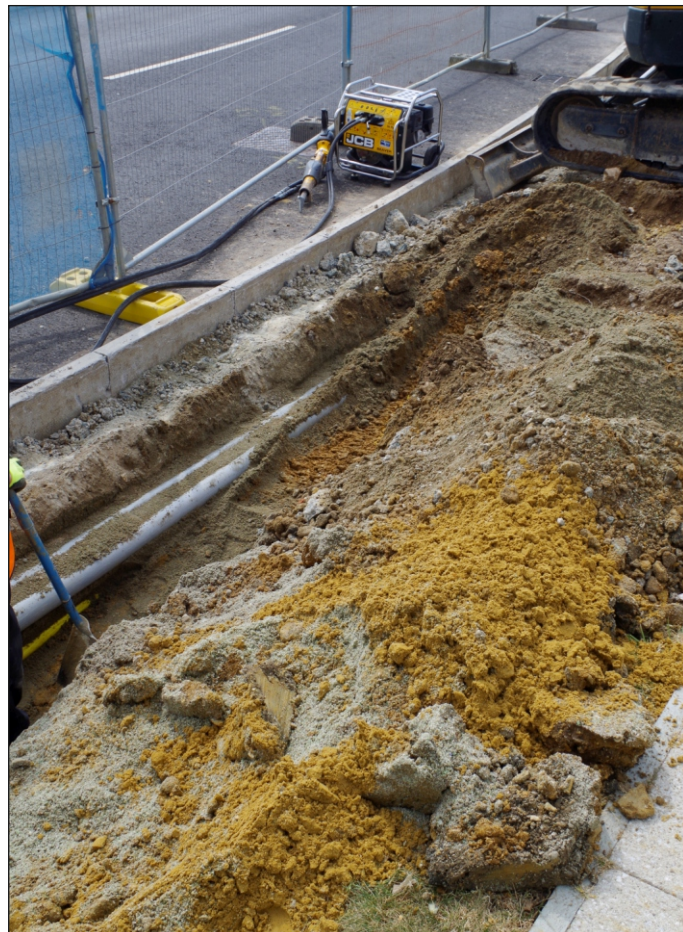
Plate 6: Excavation of Zone 2, looking south east
