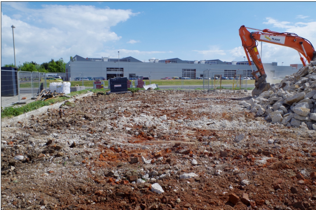
Plate 8: Excavation of Zone 3, looking south
