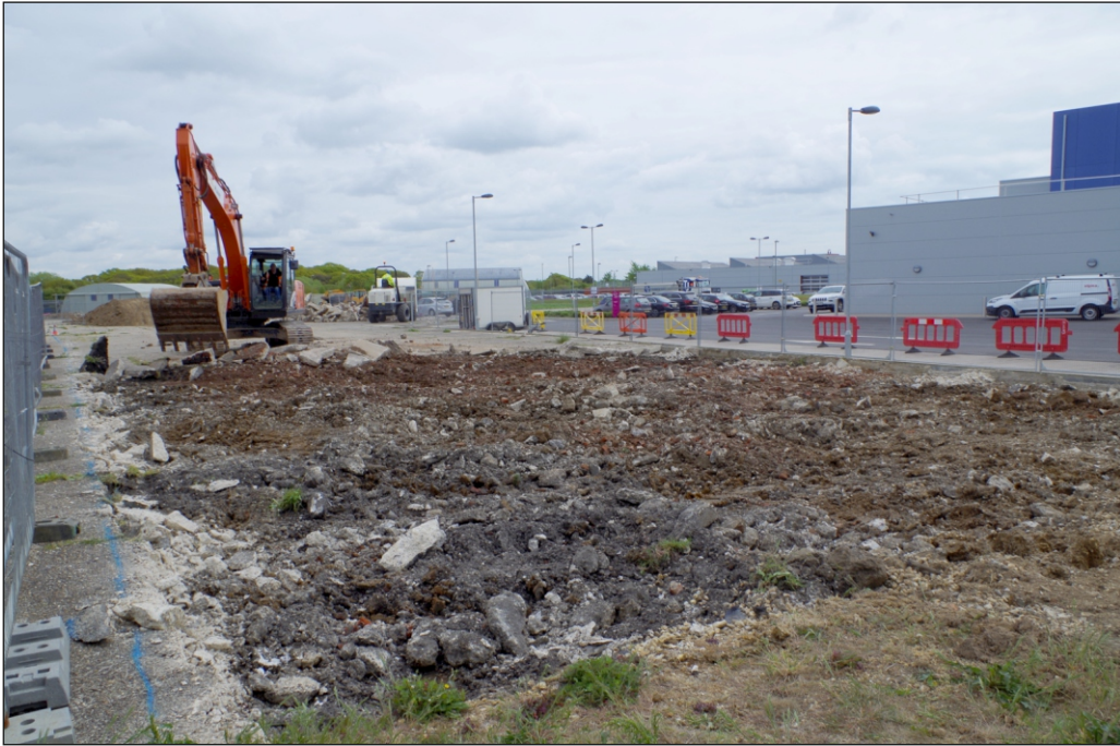
Plate 9: Excavation of Zone 4, looking east
