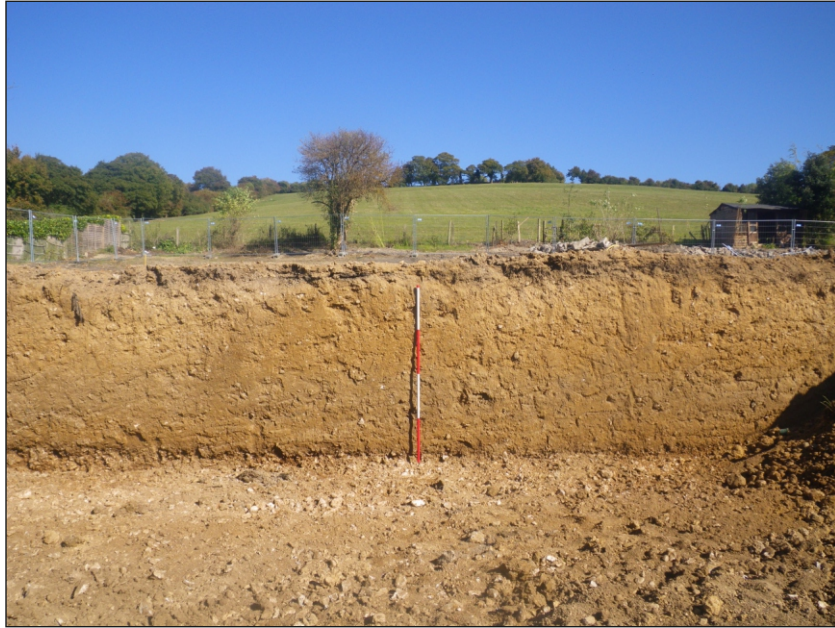
Plate 3: Southwest facing section of bank excavation
