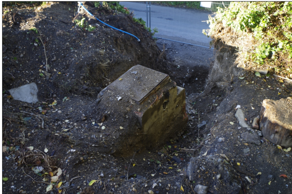
Plate 2: View of existing manhole within the site
