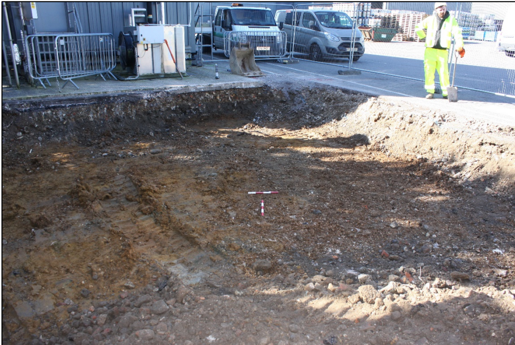
Plate 4: View of the top of the natural sandy clay and flint gravel across the excavation area. (Scale 0.5 m and 0.4 m)
