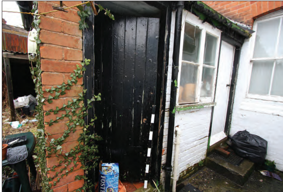
Plate 52: 16 Chesil Street: rear extension (2009)
