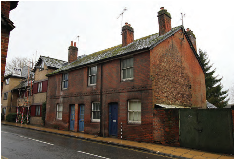
Plate 36: 16-20 Chesil Street: front elevation showing scar of former building at 16a Chesil Street (2009)
