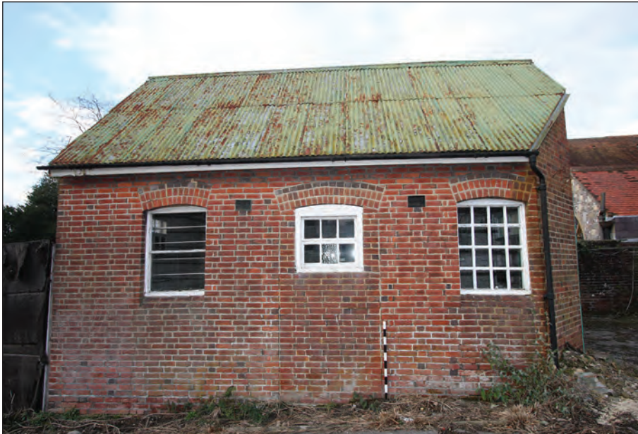
Plate 28: Rear workshop: south wall showing blocked central doorway (2009)
