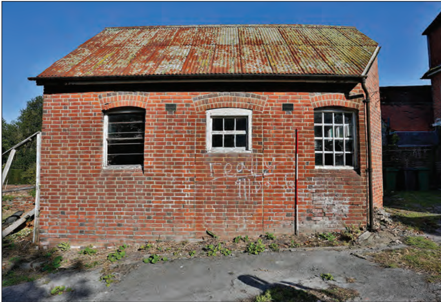
Plate 29: Rear workshop: south wall showing blocked central doorway (2019)
