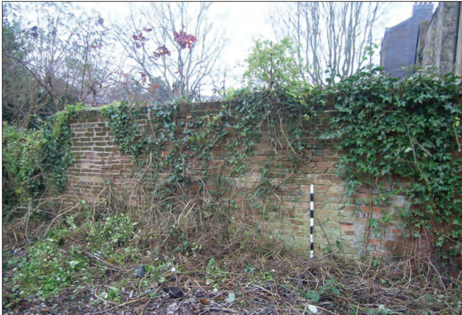
Plate 72: Wall 1 viewed from the south-east 2
