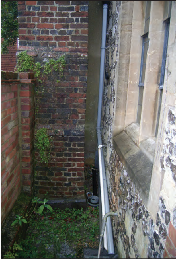
Plate 7: External space to the west of the former Vestry (2012)
