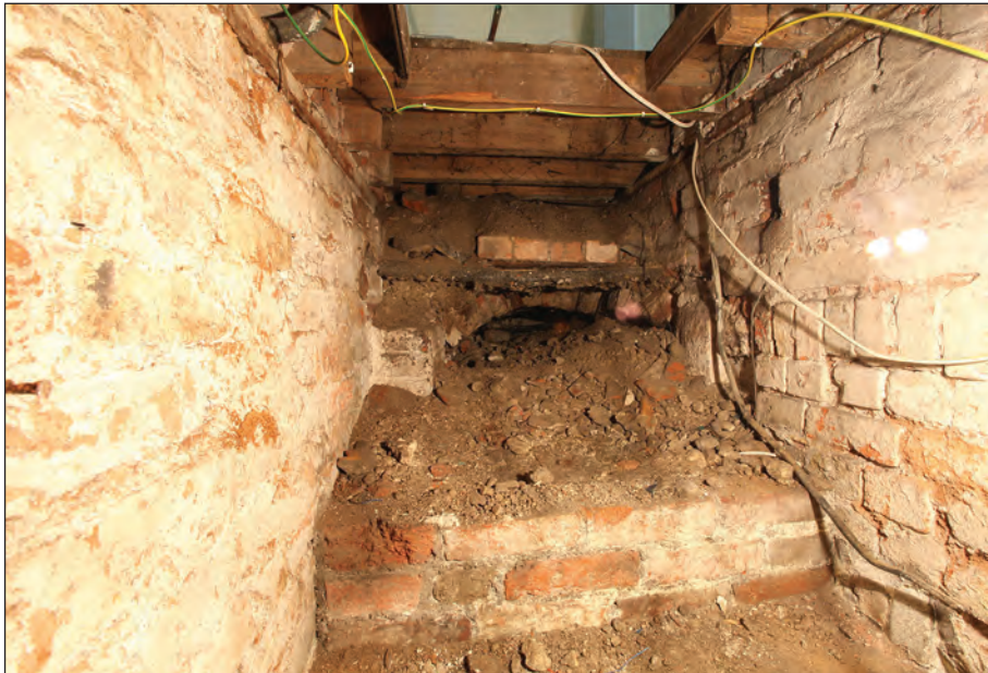
Plate 66: Top of the staircase with blocked passageway beyond
