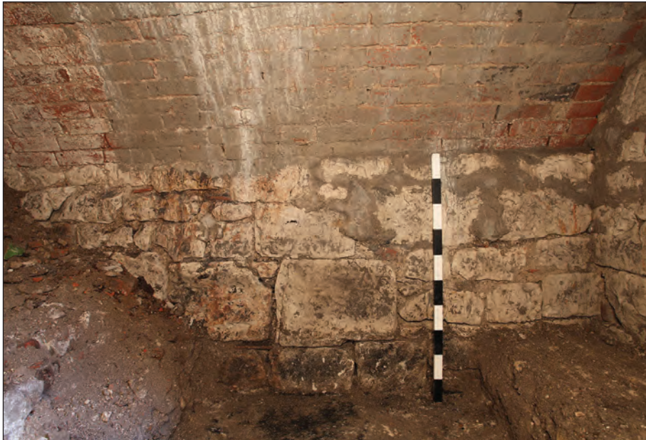
Plate 60: Exposed south wall of rear chamber
