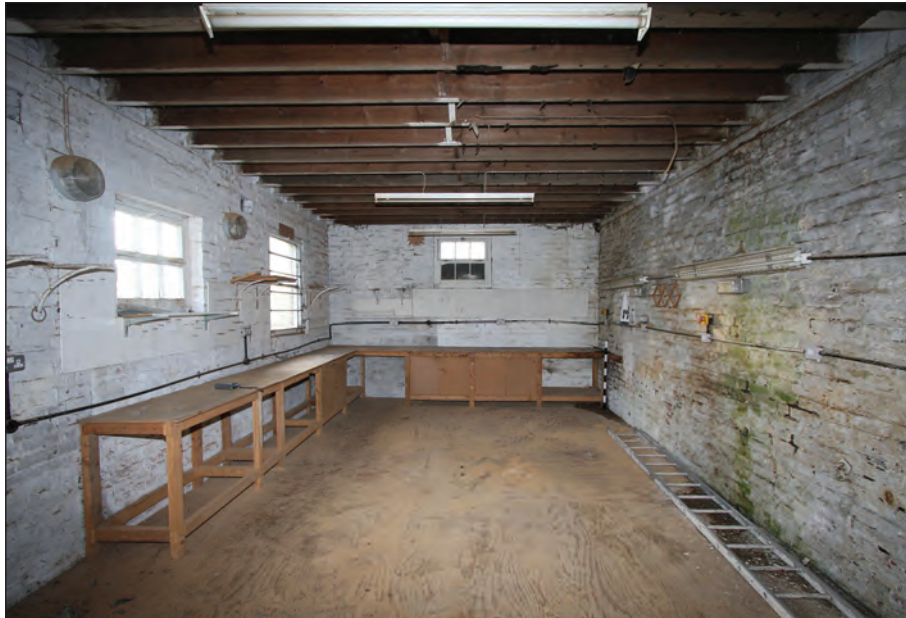
Plate 32: Rear workshop: ground floor interior (2009)
