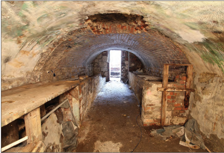
Plate 57: Rear chamber viewed from the east
