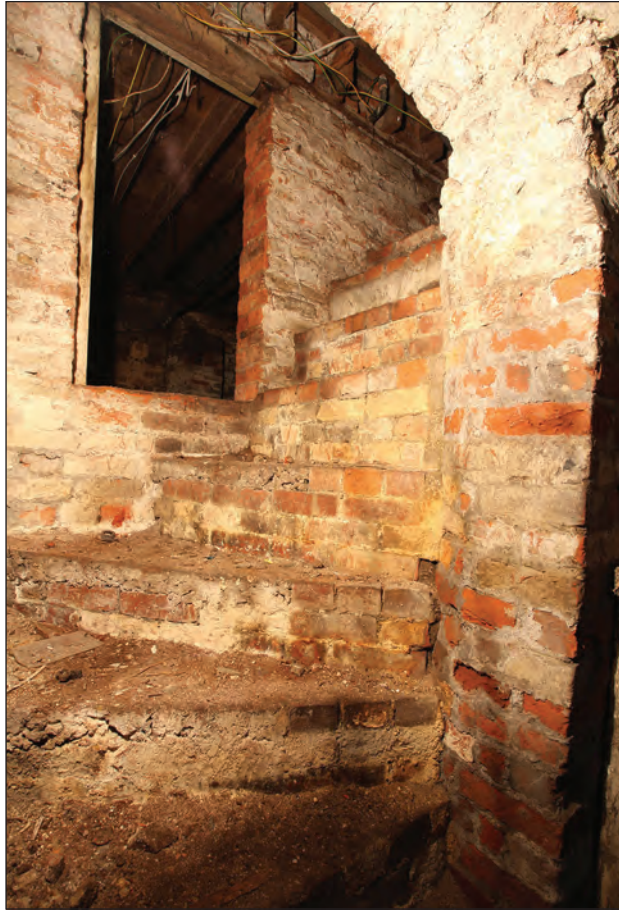
Plate 65: Straight flight with winder stair viewed from the north-west
