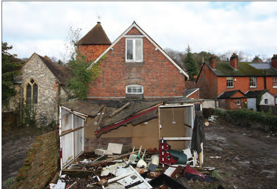
Plate 31: Rear workshop: west elevation with dilapidated lean-to (2009)
