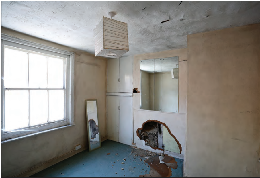
Plate 45: 20 Chesil Street: front bedroom (2019)
