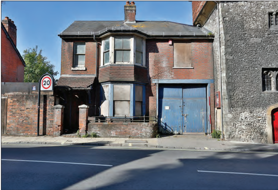
Plate 17: East elevation of 14 Chesil Street and St Peter's Church (2019)
