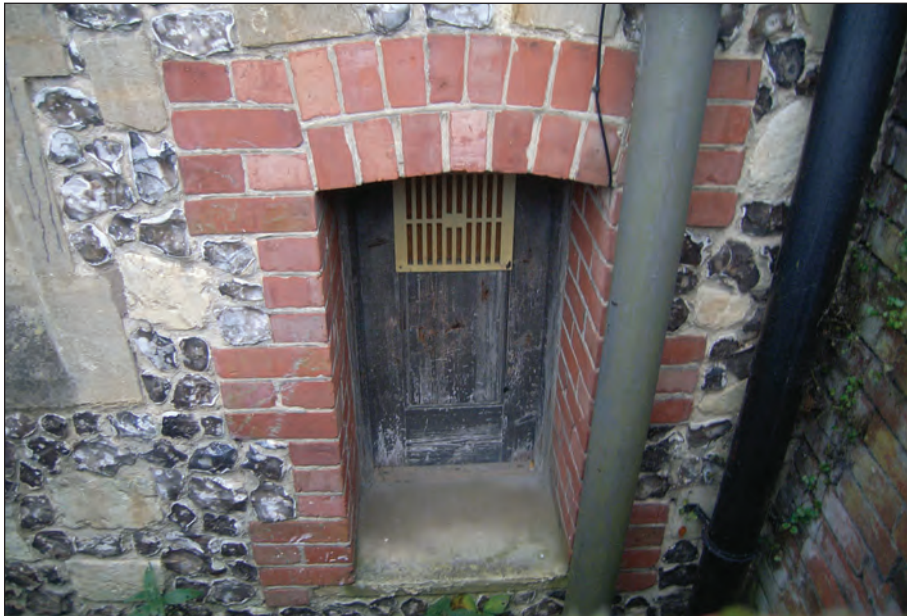
Plate 6: Access hatch in the west wall of the Vestry (2012)
