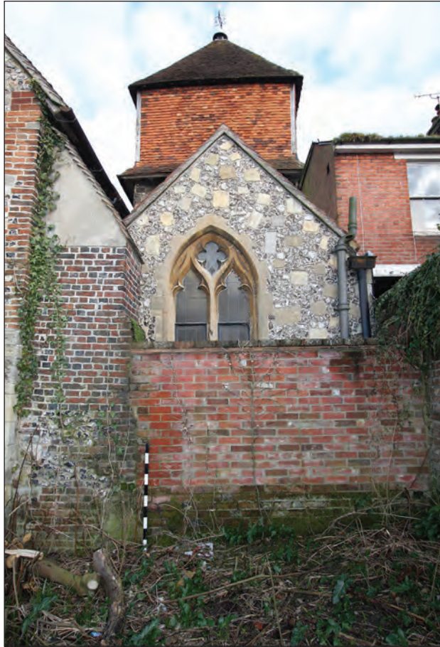
Plate 5: The Vestry viewed from the west
