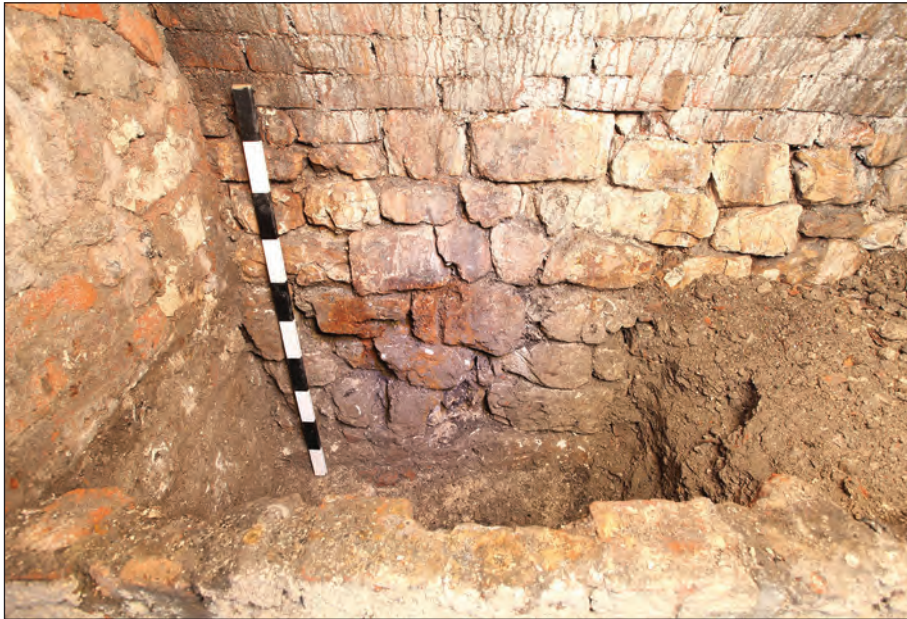
Plate 59: Exposed north wall of rear chamber
