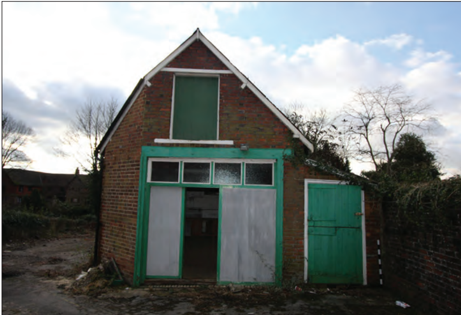
Plate 30: Rear workshop: east elevation (2009)
