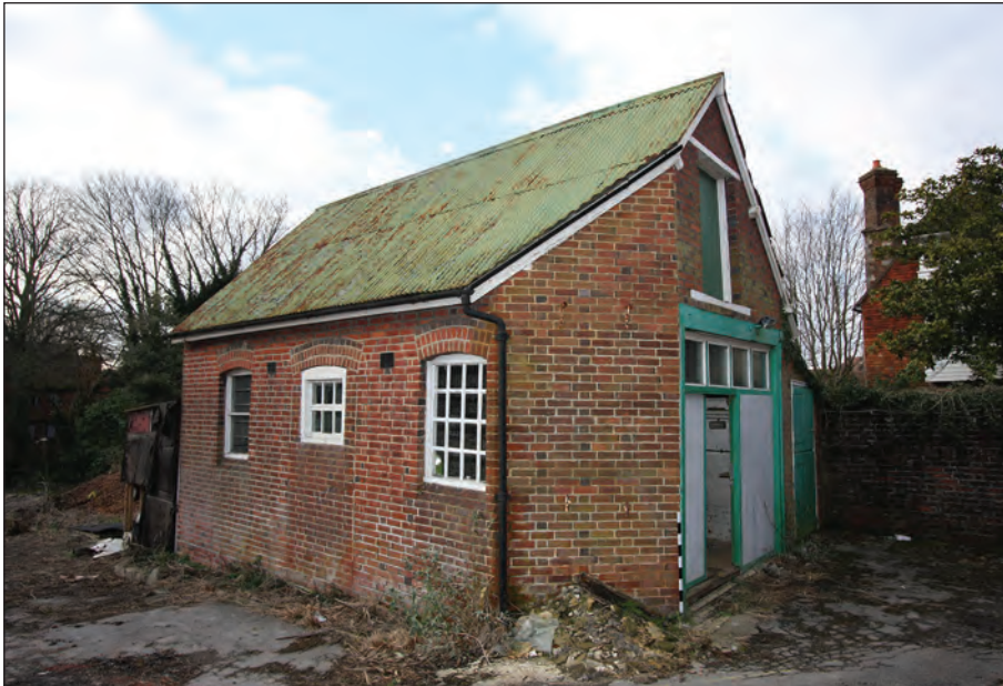
Plate 26: Rear workshop viewed from the south-east (2009)
