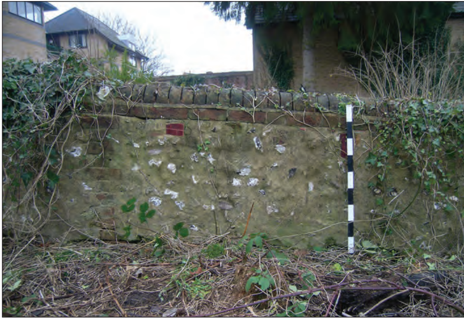
Plate 75: Wall 3 viewed from the north
