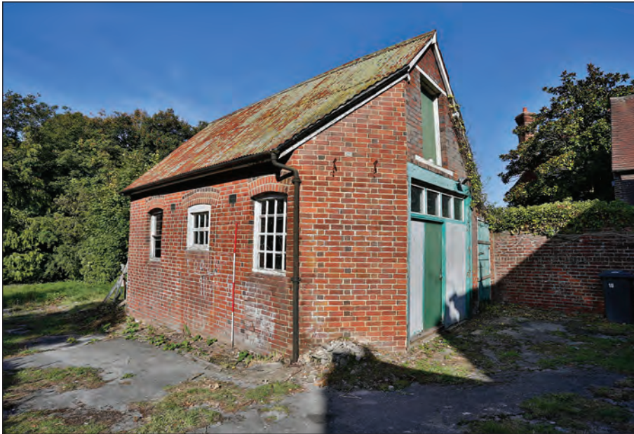
Plate 27: Rear workshop viewed from the south-east (2019)
