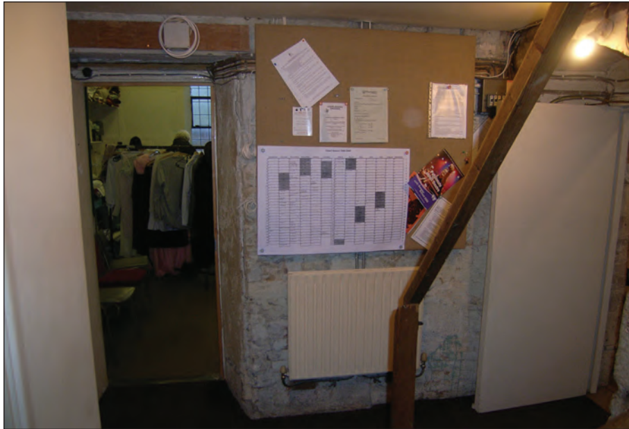
Plate 11: West wall of the Bell Tower viewed from the east (2012)
