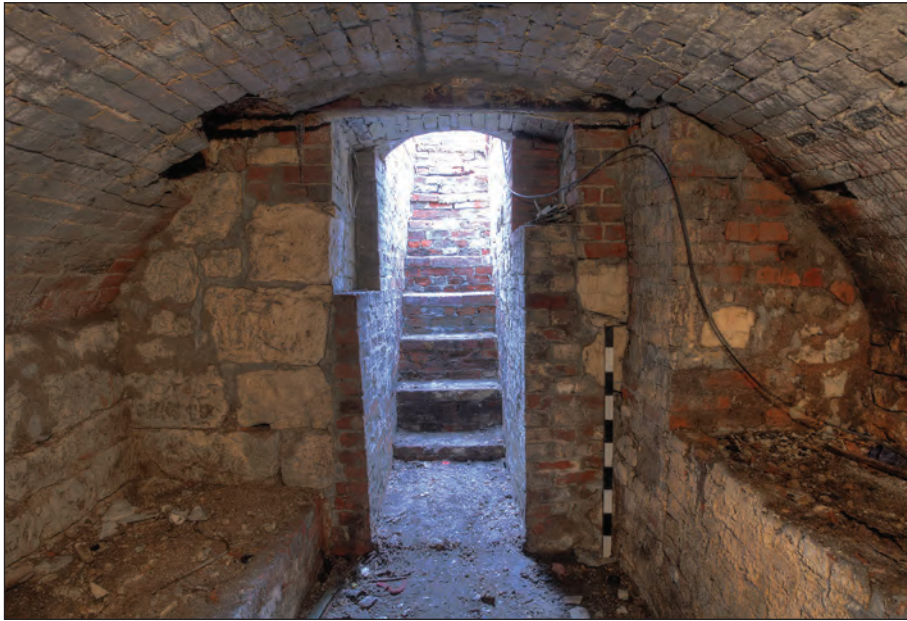
Plate 63: West wall of rear chamber
