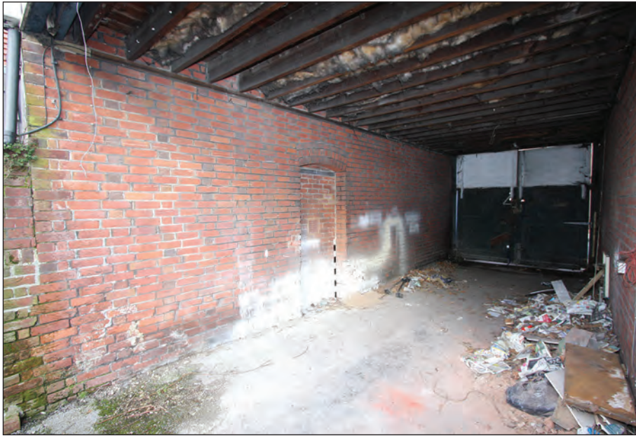
Plate 3: Blocked entrance in the north wall of the covered carriageway at 14 Chesil Street (2012)
