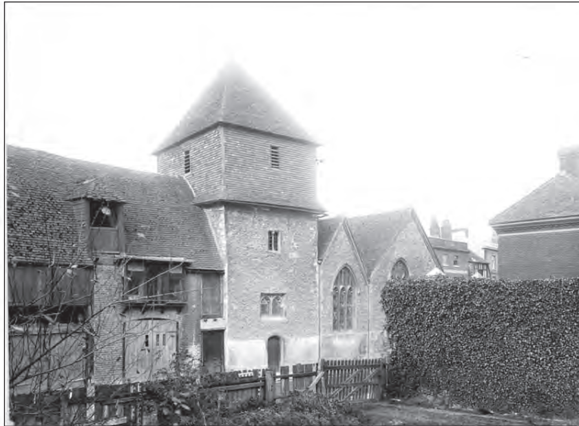
Plate 1: Photograph dated c.1880 showing former industrial building at 14 Chesil Street adjoining St Peter's Church
