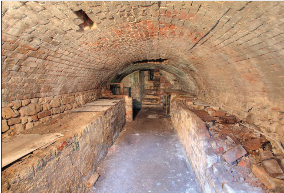
Plate 56: Rear chamber viewed from the west
