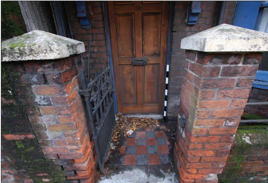
Plate 18: Front gates and entrance to 14 Chesil Street (2009)
