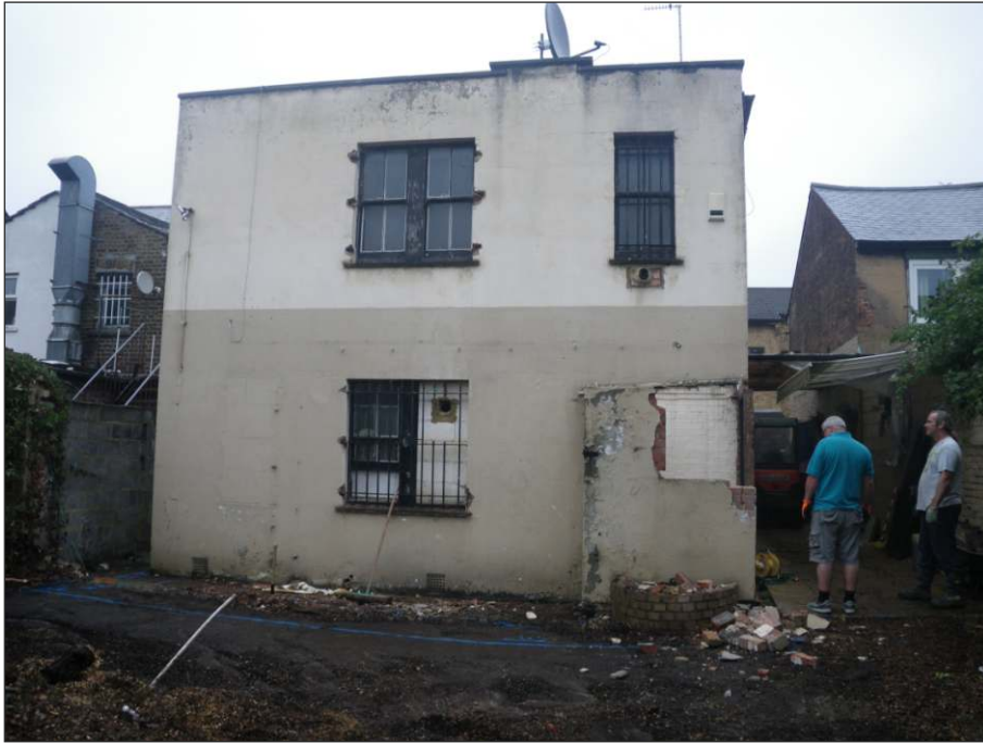
Plate 1: North-east facing shot of foundation trench and rear of existing building
