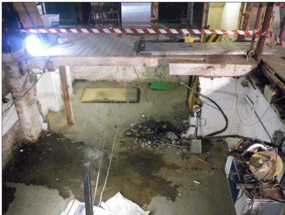
Plate 6: South-west facing shot of interior basement
