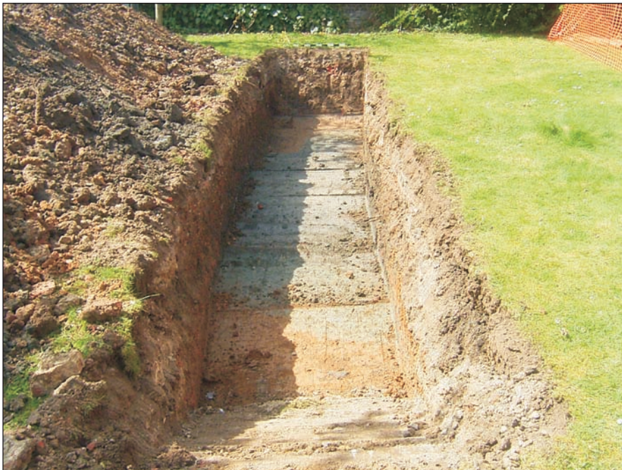
Plate 1: Trench 1, view from east
