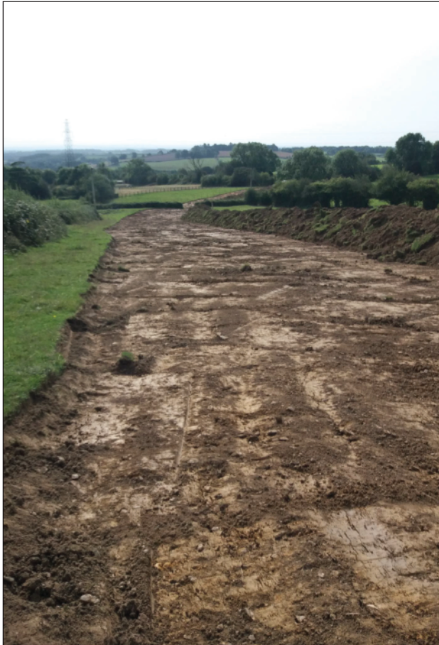
Plate 1: Northern end of scheme following topsoil removal, view from east
