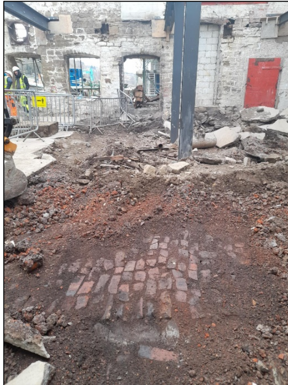
Plate 9: Client photograph 6, exposed brick-paved surface within Building 10, facing southeast
