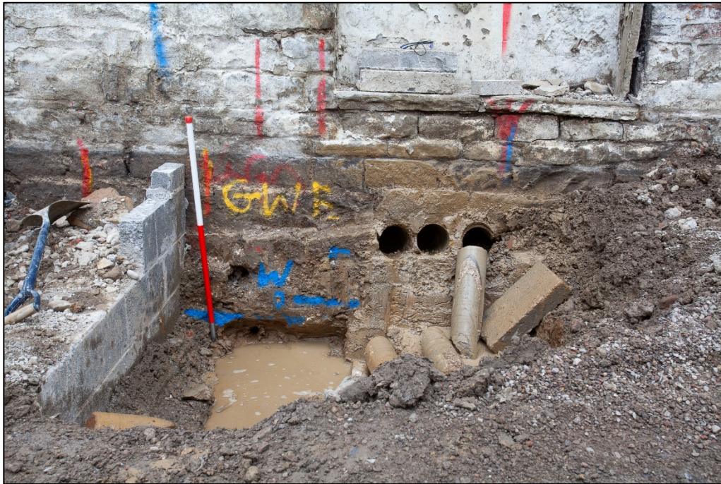
Plate 1: Re-excitation to the north-eastern end of the northwest wall of Building 10, facing northwest
