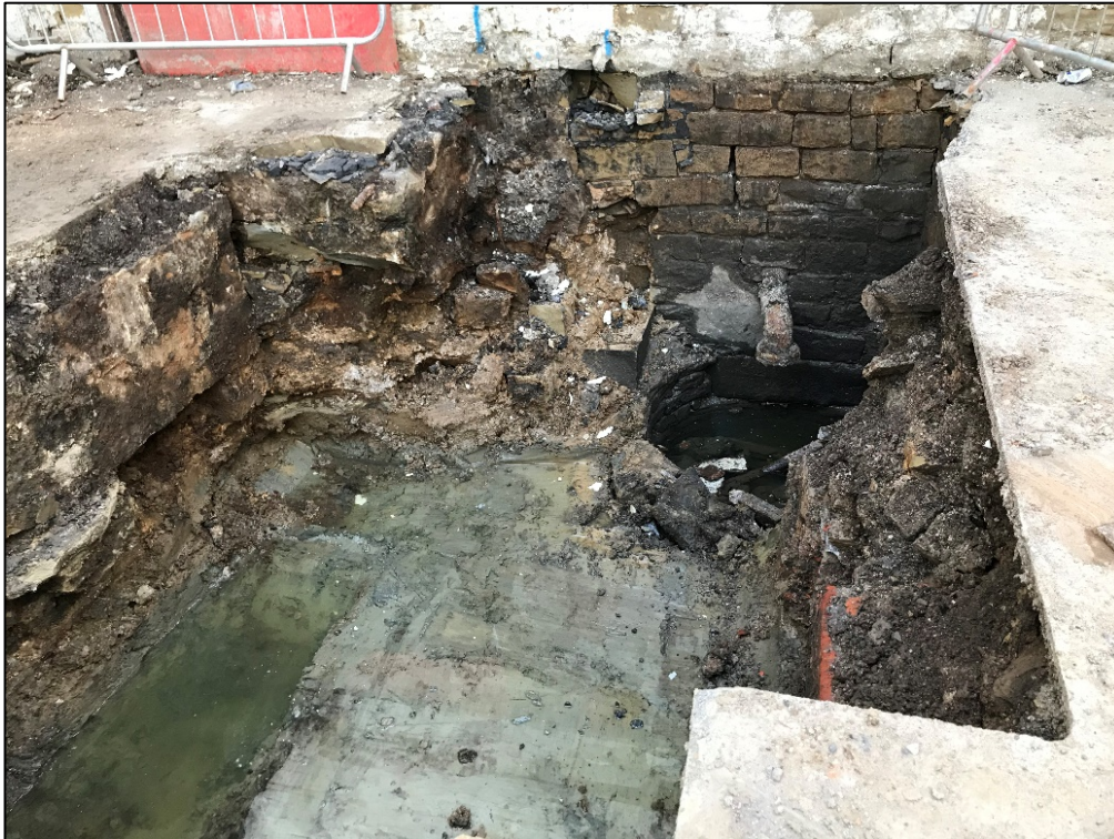
Plate 5: Client photograph 2, showing excavations within the southwest end of Building 10, facing southwest. Note the machine bases (left), redeposited natural (1002), and underlying natural (1001), with a linear brick structure right, leading to a cistern / well abutting the wall to Building 11
