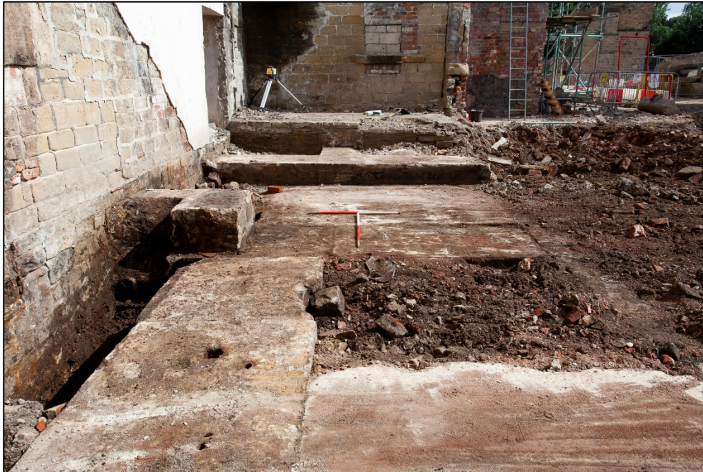
Plate 11: Exposed engine bed (2007), with abutting concrete plinths (2006) for the later press, Building 11, facing southwest (see Figure 3)
