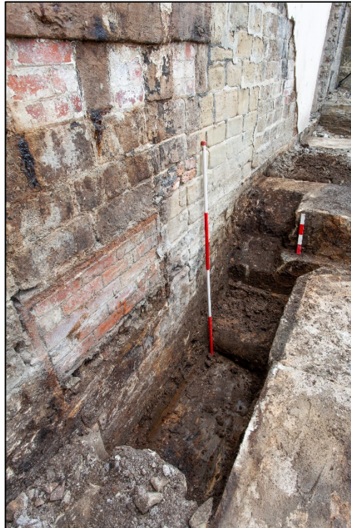
Plate 13: Excavated sondage within the wheel pit, facing southeast. Note the exposed pipe to its base
