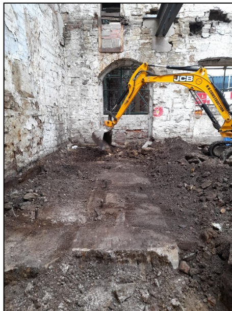
Plate 6: Client photograph 5, showing excavations within the southwest end of Building 10, revealing large stone machine beds, facing northwest
