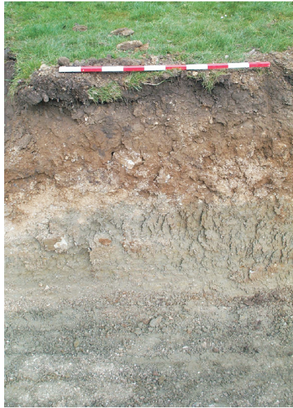
Representative section of foundation trench
