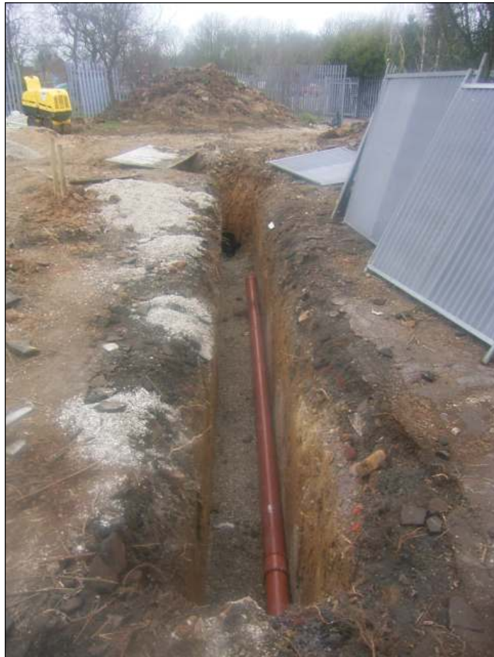
Plate 2: Pipe trench from northeast
