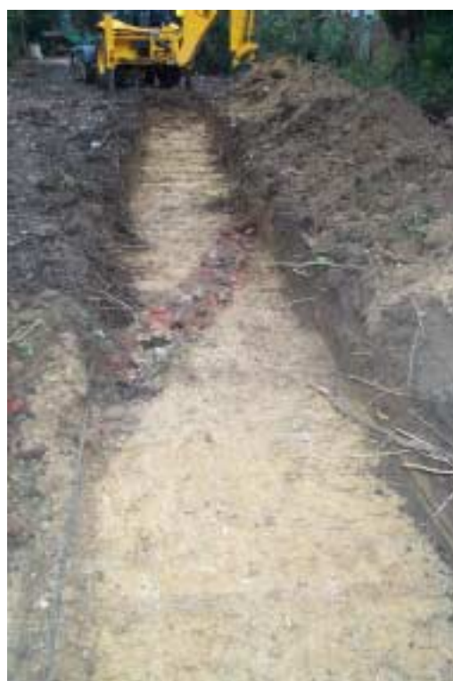
Plate 3: General view of Trench 3 taken from west
