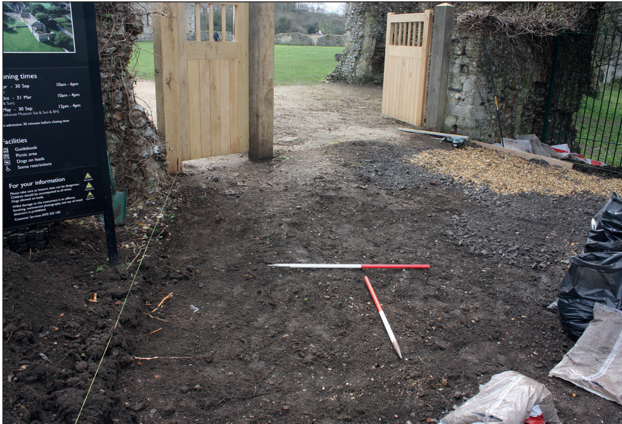
Plate 4: Gatehouse apron with surface removed, view from the north-west (1 m and 2 m scales)
