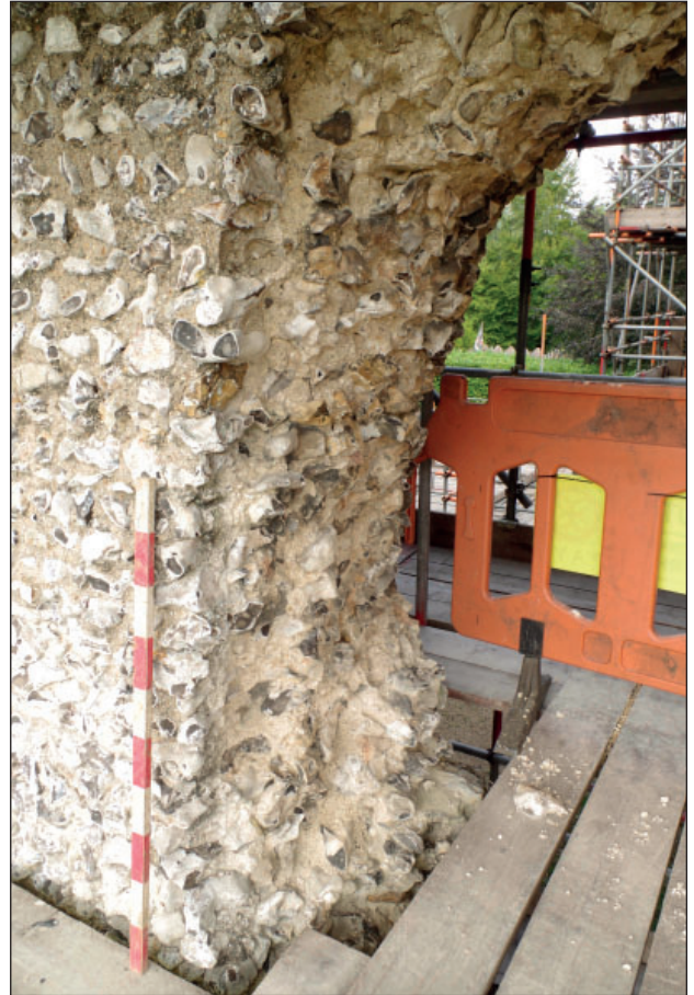
Plate 40: East wall arch in Kitchen from the north-east (1 m scale)
