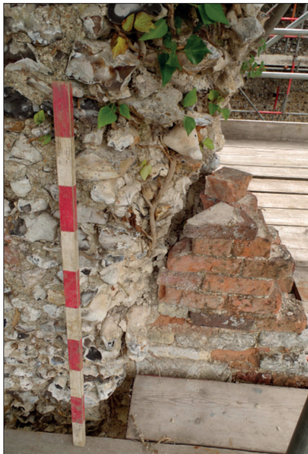
Plate 42: West wall of Kitchen from the west (1m scale)
