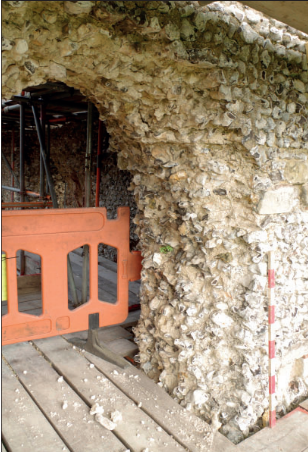
Plate 39: East wall arch in Kitchen from the south-east (1 m scale)
