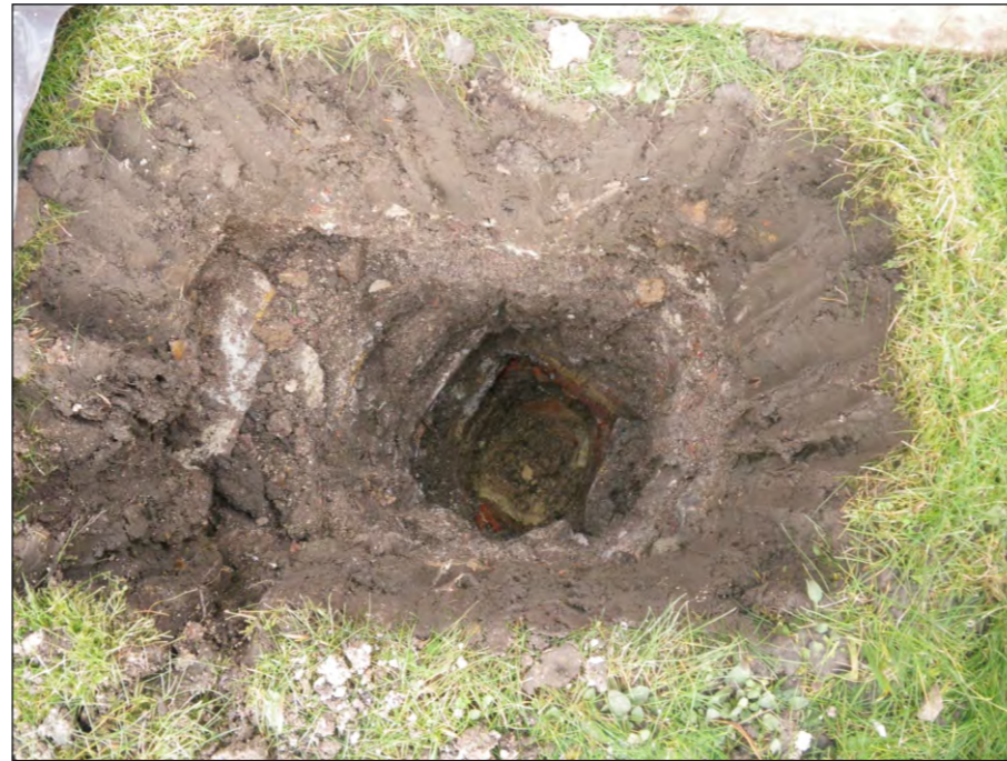
Plate 2: WS1 hand dug hole to 1.25m
