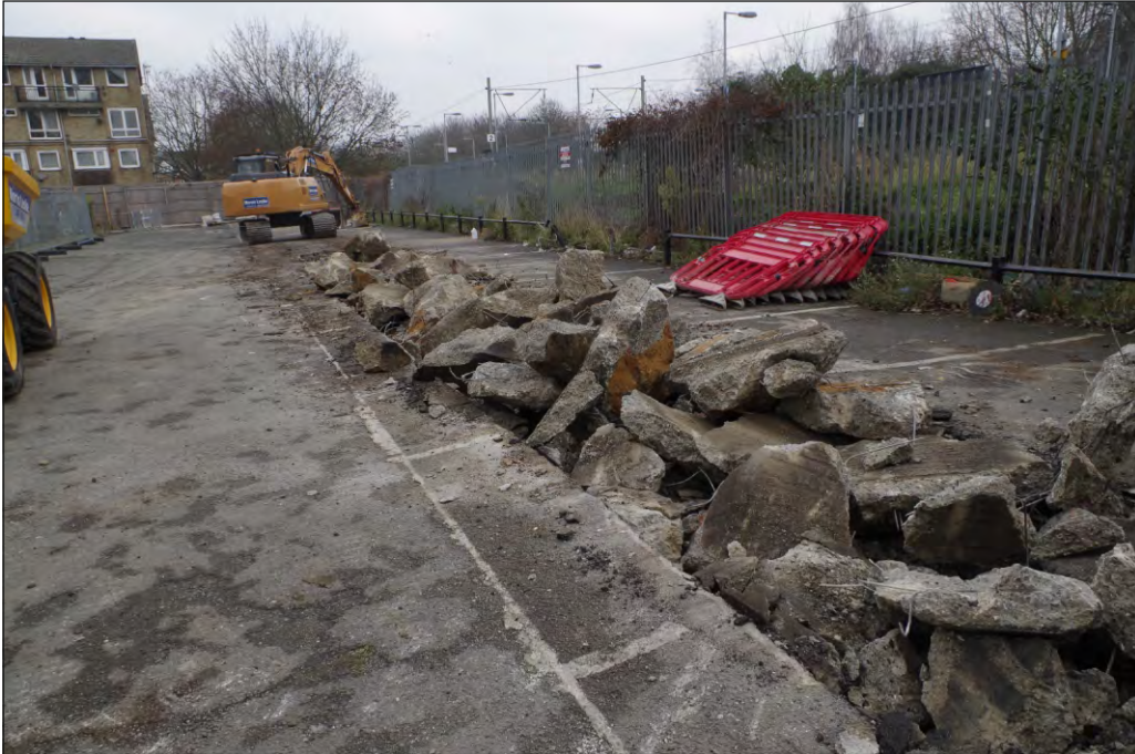
Plate 9: Trench 6, reinforced concrete layer
