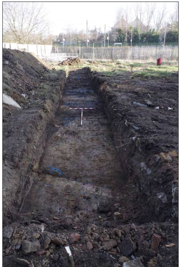
Plate 4: Trench 3, viewed from the west. 19th century terraced housing wall in foreground, modern truncation in the background
