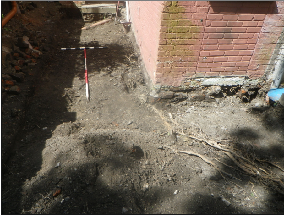
Plate 1: Trench 1 shot of 'raft' excavation. View from the north-east
