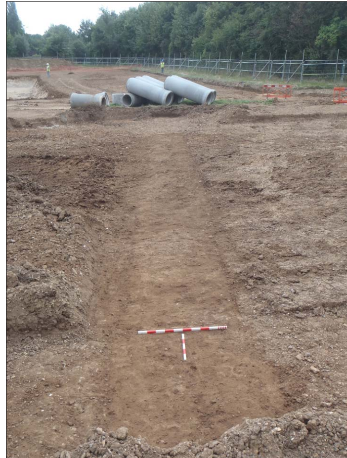
Plate 2: Ditch 6315: view looking south-west (to north of 2010 recorded stretch of ditch)
